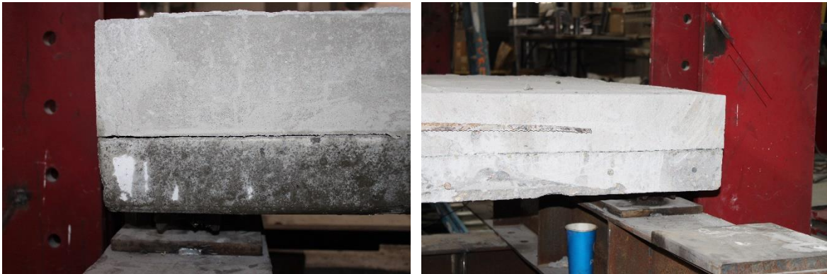
Figure 5.1 Unmodified deck panel prior to starting testing with delamination shown. Southwest; left, Northwest; right.
