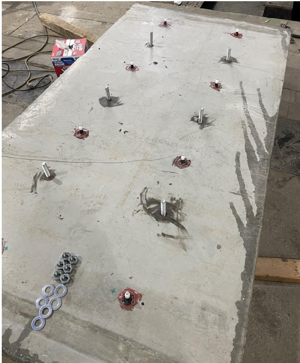
Figure 3.17 Completed installation of proprietary anchors and epoxy injection ports.
