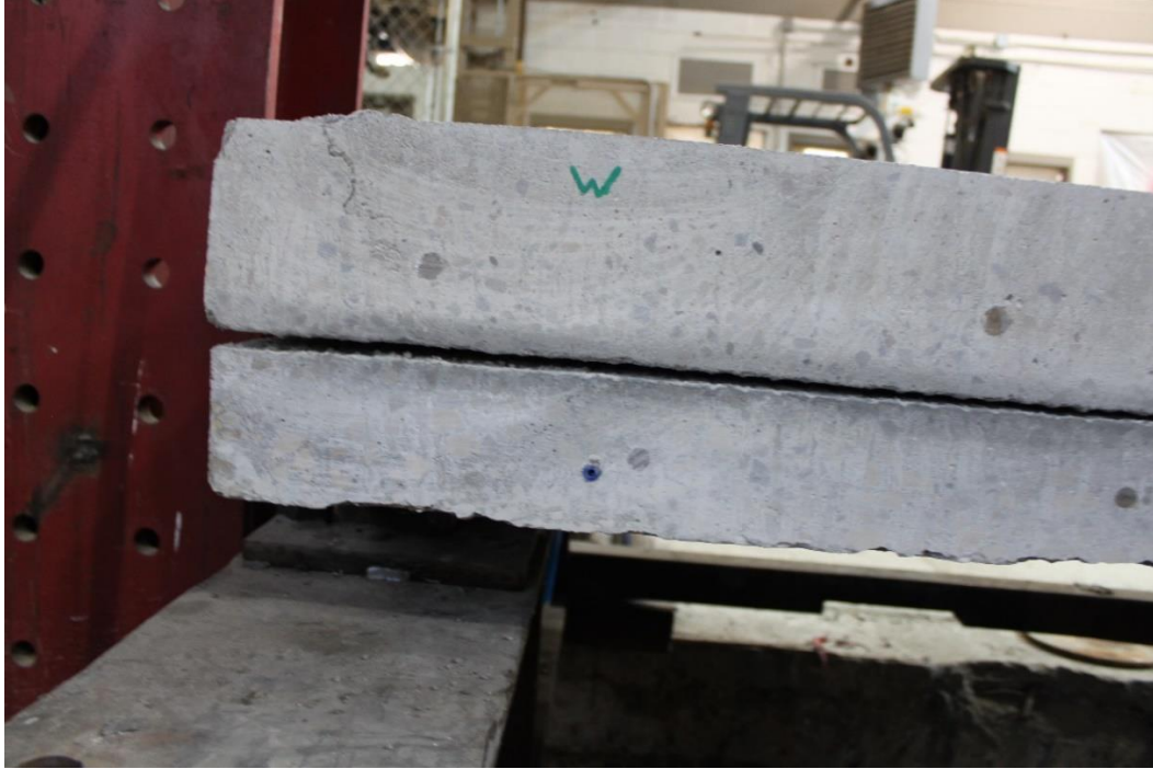
Figure 5.9 Delamination of epoxy retrofit deck panel at applied displacement of 4.0 in. (Location: northwest)
