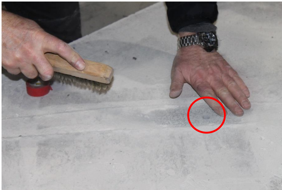
Figure 3.3 Epoxy injection port hole preparation.
