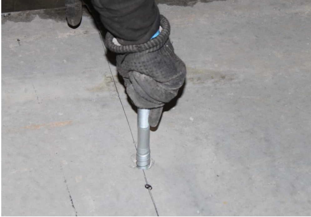
Figure 3.8 Proprietary anchor being placed into the concrete panel.
