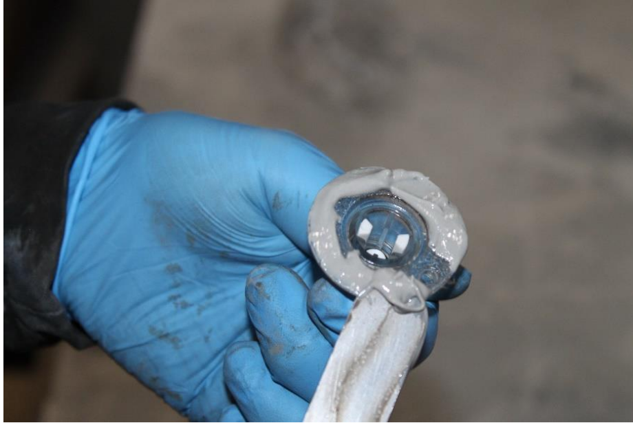
Figure 3.4 Application of adhesive to epoxy injection port.
