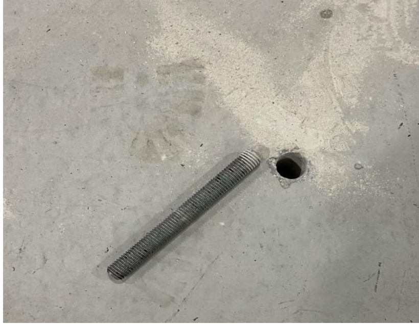
Figure 3.15 Nonproprietary shear anchor prior to installation.
