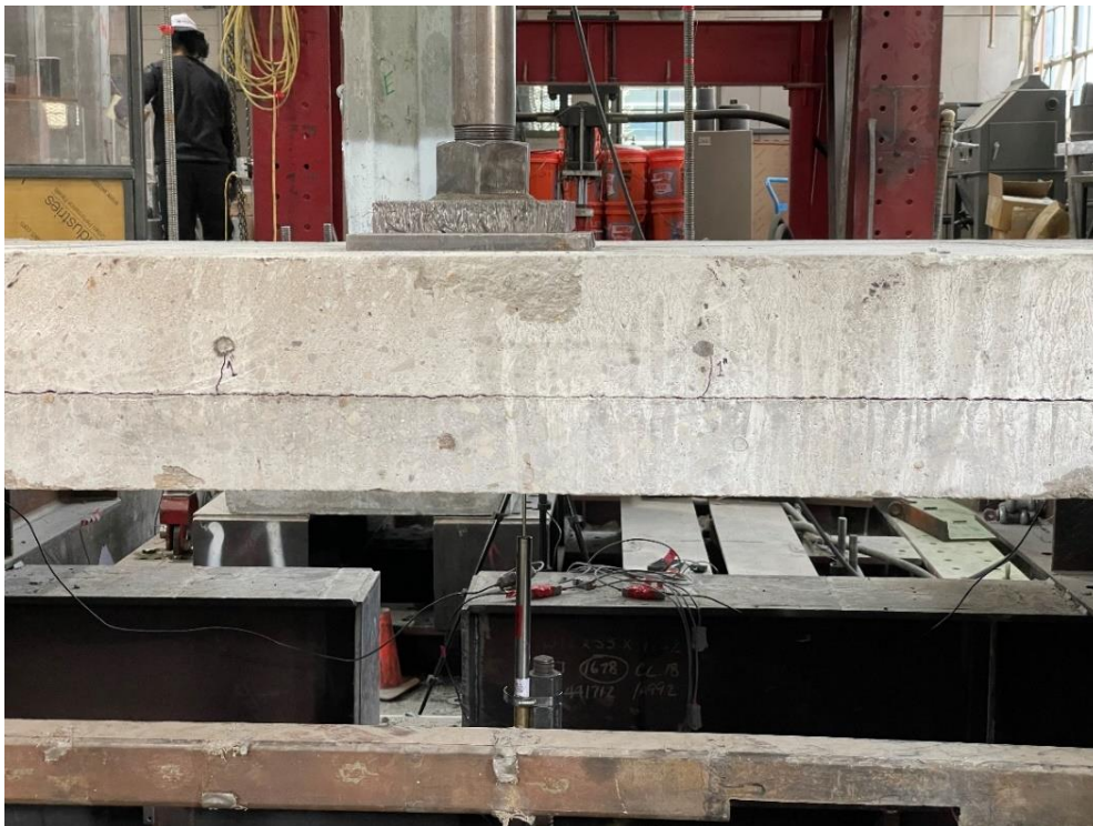
Figure 5.18 CFRP retrofit deck panel cracks at 1.0-in. displacement. (Location: east, mid-span)
