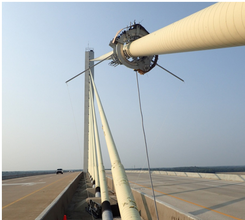
Figure 32. Photo. Protective tape wrapped on HDPE pipe on stay cables.
