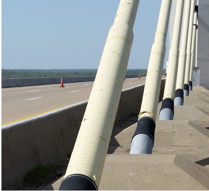
Figure 32. Photo. Protective tape wrapped on HDPE pipe on stay cables.
