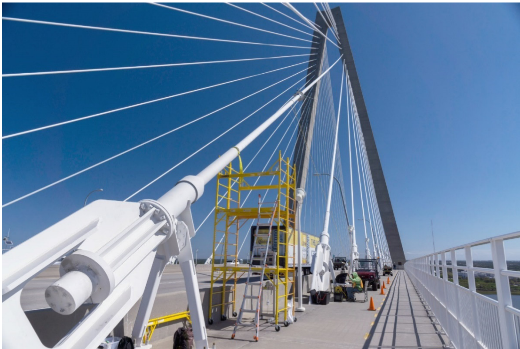
Figure 114. Photo. The anchorages and external dampers at the center of the main span of the bridge.
