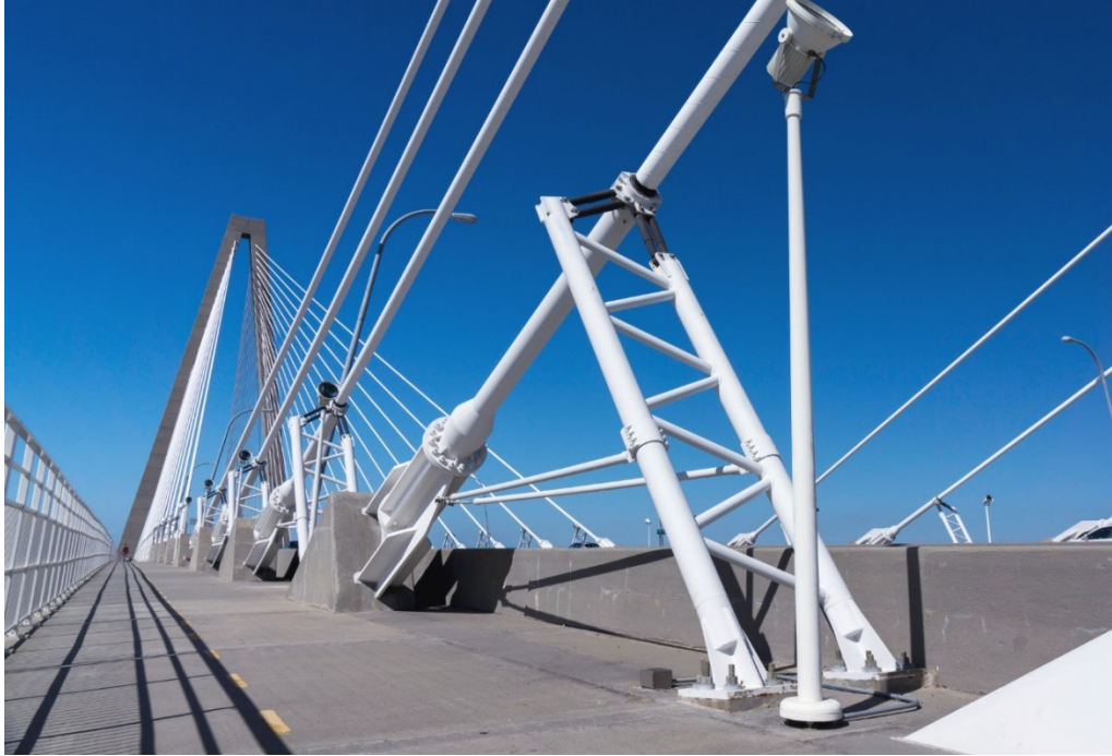
Figure 114. Photo. The anchorages and external dampers at the center of the main span of the bridge.
