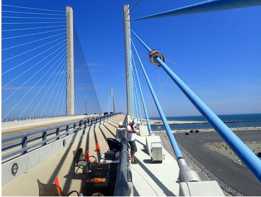
Figure 21. Photo. The cable robot climbing a cable with the Indian River Inlet Bridge in the background.
