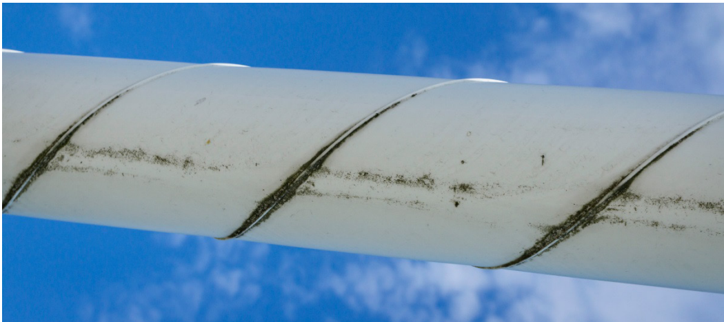
Figure 102. Photo. Dirt collecting on the underside of a cable from the Pomeroy-Mason Bridge.
