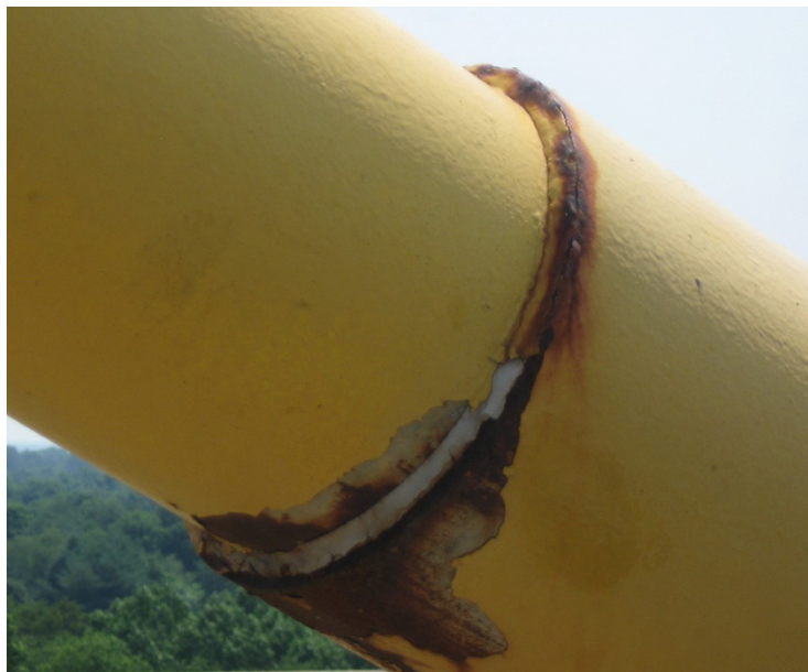
Figure 9. Photo. Surface texture of steel pipe sheathing stay cable.
