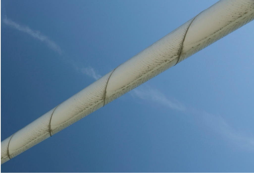
Figure 111. Photo. Rain flow patterns in dirt on the underside of a stay cable.
