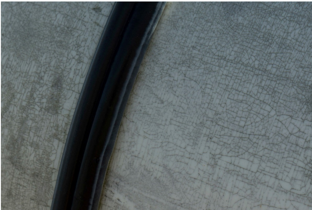
Figure 111. Photo. Rain flow patterns in dirt on the underside of a stay cable.
