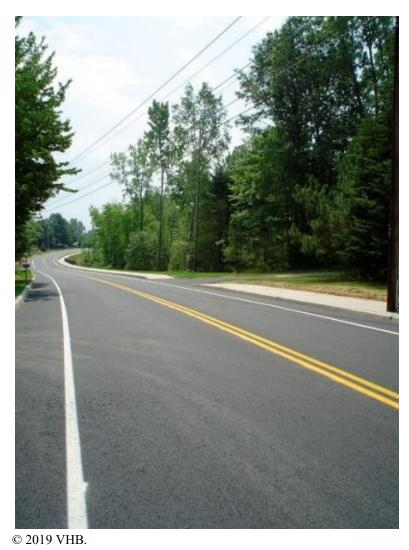
Figure 83. Photograph. Example of road where width was increased to add bike lanes.
