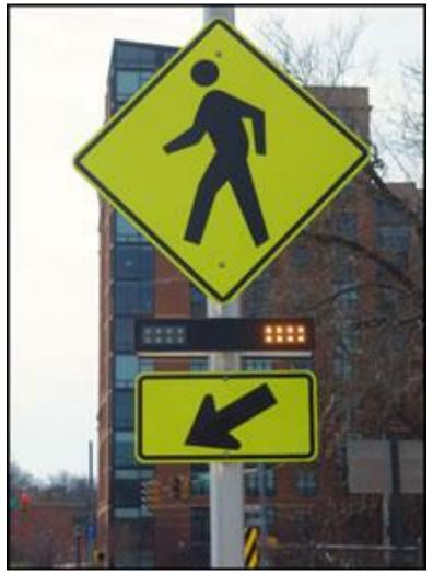
Source: FHWA. Figure 79. Photograph. Example of an RRFB (FHWA 2018c).
