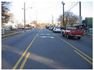
Source: FHWA. Figure 100. Photograph. Example of a TWLTL (Persaud et al. 2007).
