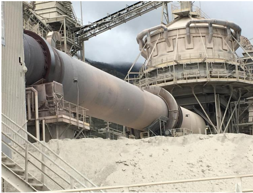
Kiln of a Lime Producing Plant
