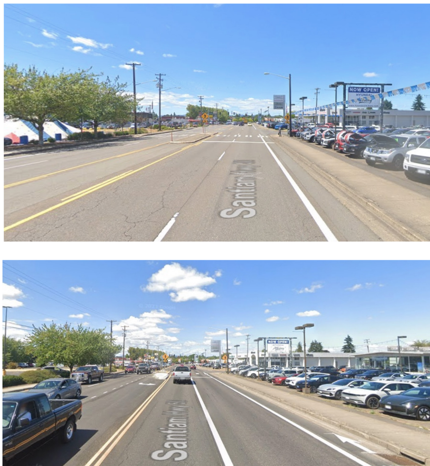
FIGURE 3.2: ALBANY – SANTIAM HIGHWAY REFERENCE IMAGE (TOP IMAGE IS PRIOR TO CONSTRUCTION AND BOTTOM IS AFTER CONSTRUCTION)
