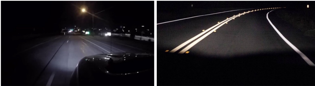
FIGURE 2.7: CONTRAST BETWEEN LOW RETROREFLECTIVITY PAVEMENT MARKINGS TO THE LEFT AND HIGH RETROREFLECTIVITY MARKINGS TO THE RIGHT (GOOGLE, 2021)
