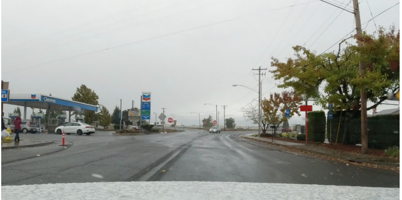
SCENARIO 7 - AIRPORT ROAD AND HIGHWAY 99 IN ALBANY WET/DAY/HYDROBLASTING
