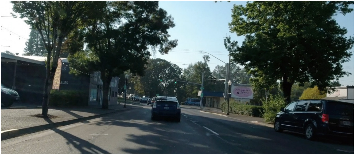
FIGURE 3.5: SPRINGFIELD – MAIN STREET REFERENCE IMAGE (TOP IMAGE IS PRIOR TO CONSTRUCTION AND BOTTOM IS AFTER CONSTRUCTION)
