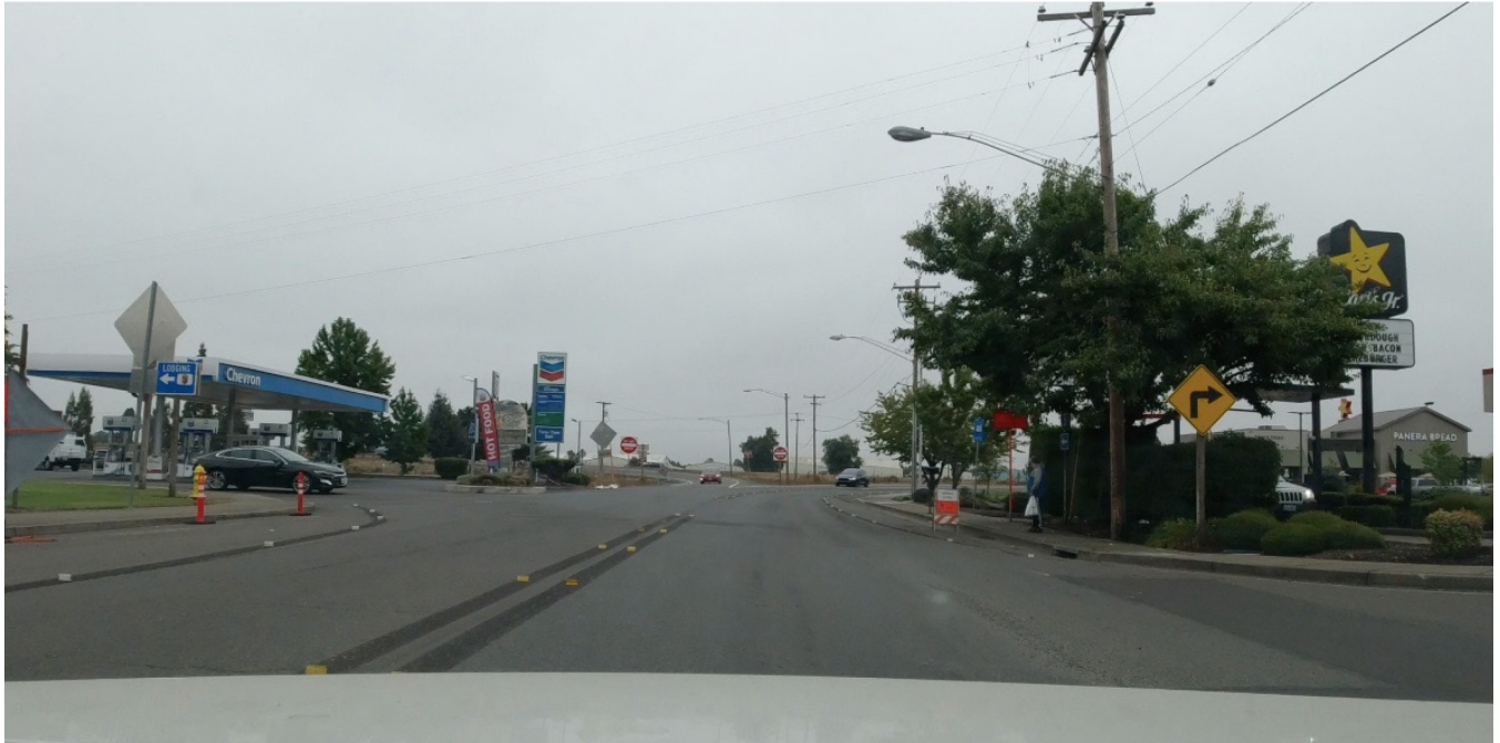
SCENARIO 1 –AIRPORT ROAD AND HIGHWAY 99 IN ALBANY DRY/DAY/HYDROBLASTING
