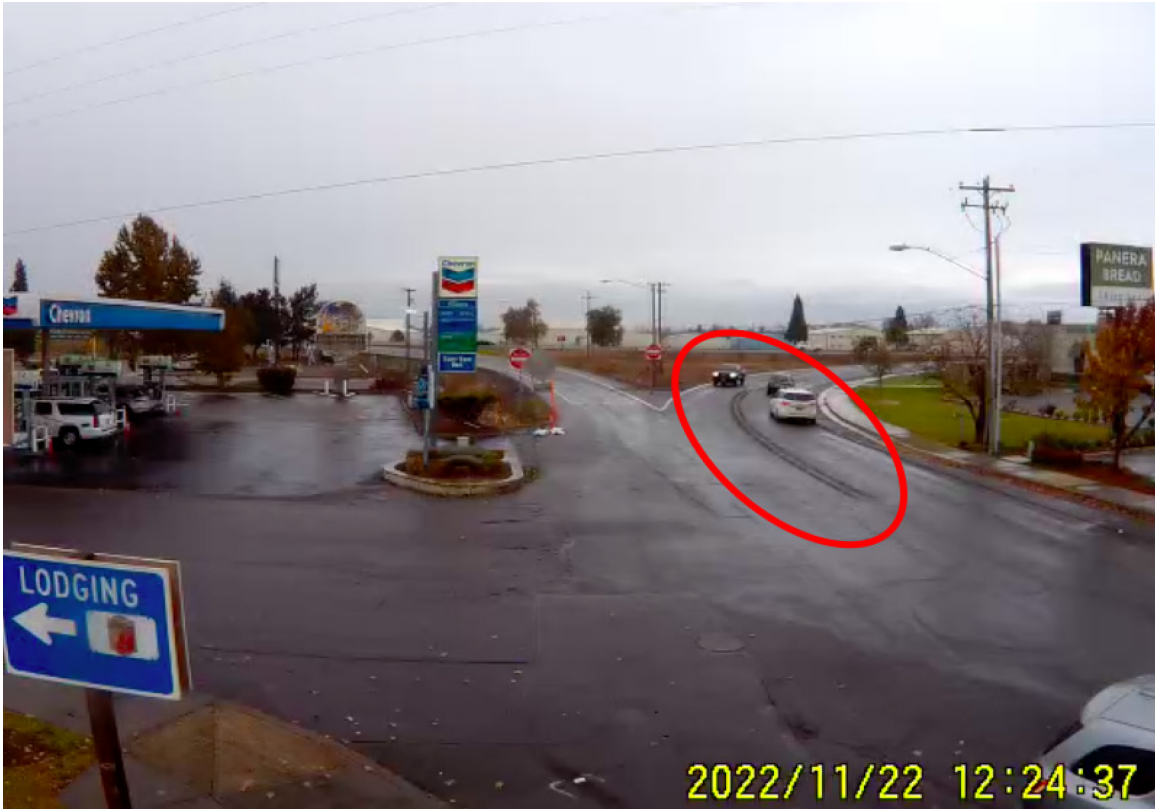
FIGURE 5.2: PAVEMENT MARKING REMOVAL ON OR 99 E, ALBANY, OR
