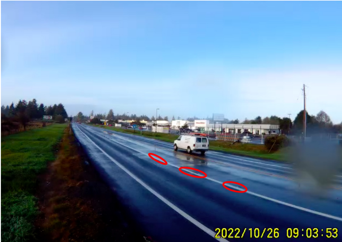
FIGURE 5.4: PAVEMENT MARKING REMOVAL ON US 101, WARRENTON, OR
