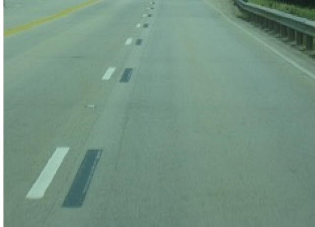
FIGURE 2.5: MASKING BEING USED TO COVER UP PAVEMENT MARKING (NCHRP, 2013)
