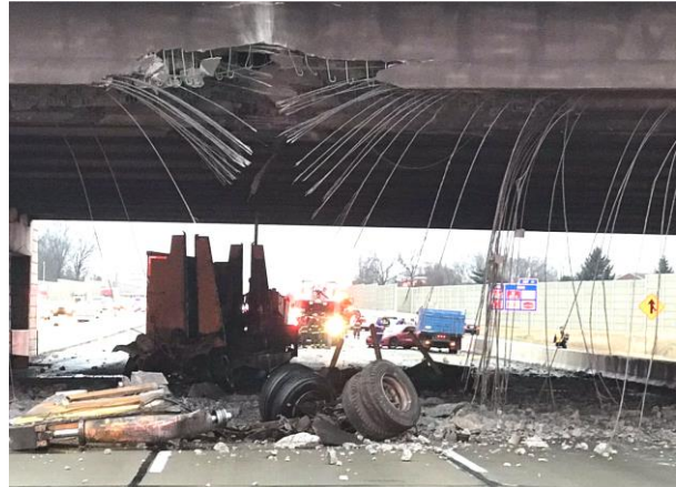
(b) Sudden, man-made. Interstate bridge collapse from truck collision with underpass, 2015, Indianapolis . (Source: Anon)
