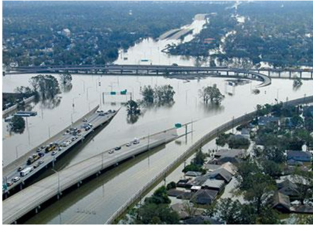
(a) Sudden, natural. Destruction of bridge after Hurricane Katrina, 2005. (Source: George Armstrong, FEMA, https://highways.dot.gov/public-roads/mayjune-2010 )
