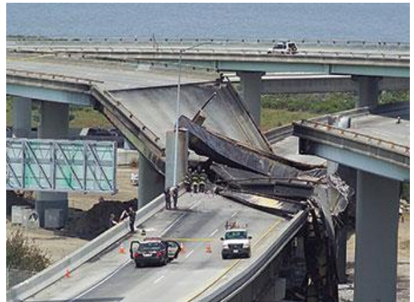
(d) Sudden, man-made. I-80 bridge collapse from truck collision with underpass, 2007, San Francisco. (Source: John Huseby, https://highways.dot.gov/public-roads/mayjune-2010 )
