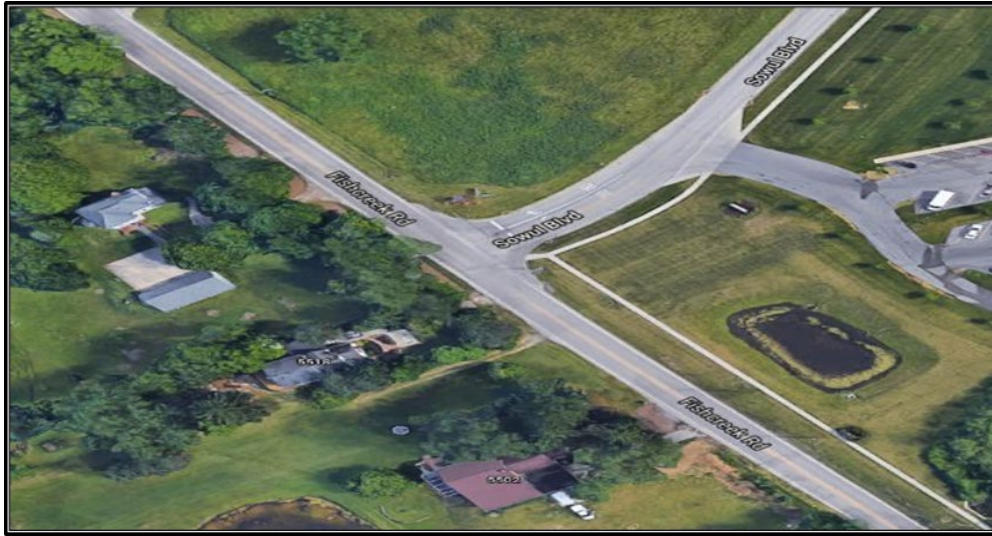
Figure IV.3 - First Test Site (Fishcreek Road at Sowul Blvd, Stow, Ohio 44224)
