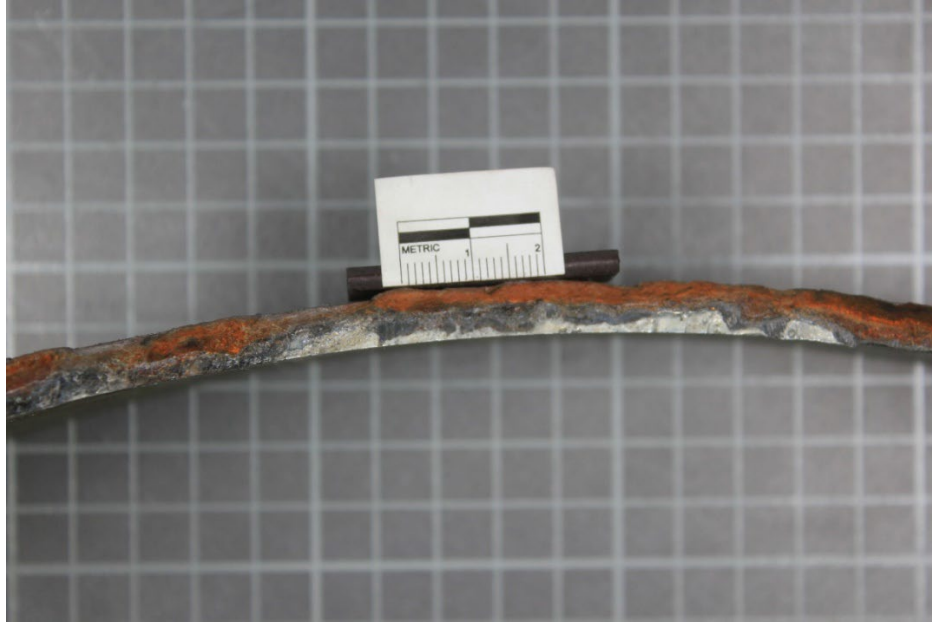
Figure 3.9: Lack of Fusion in the Center of the Pole B Crack Surface
