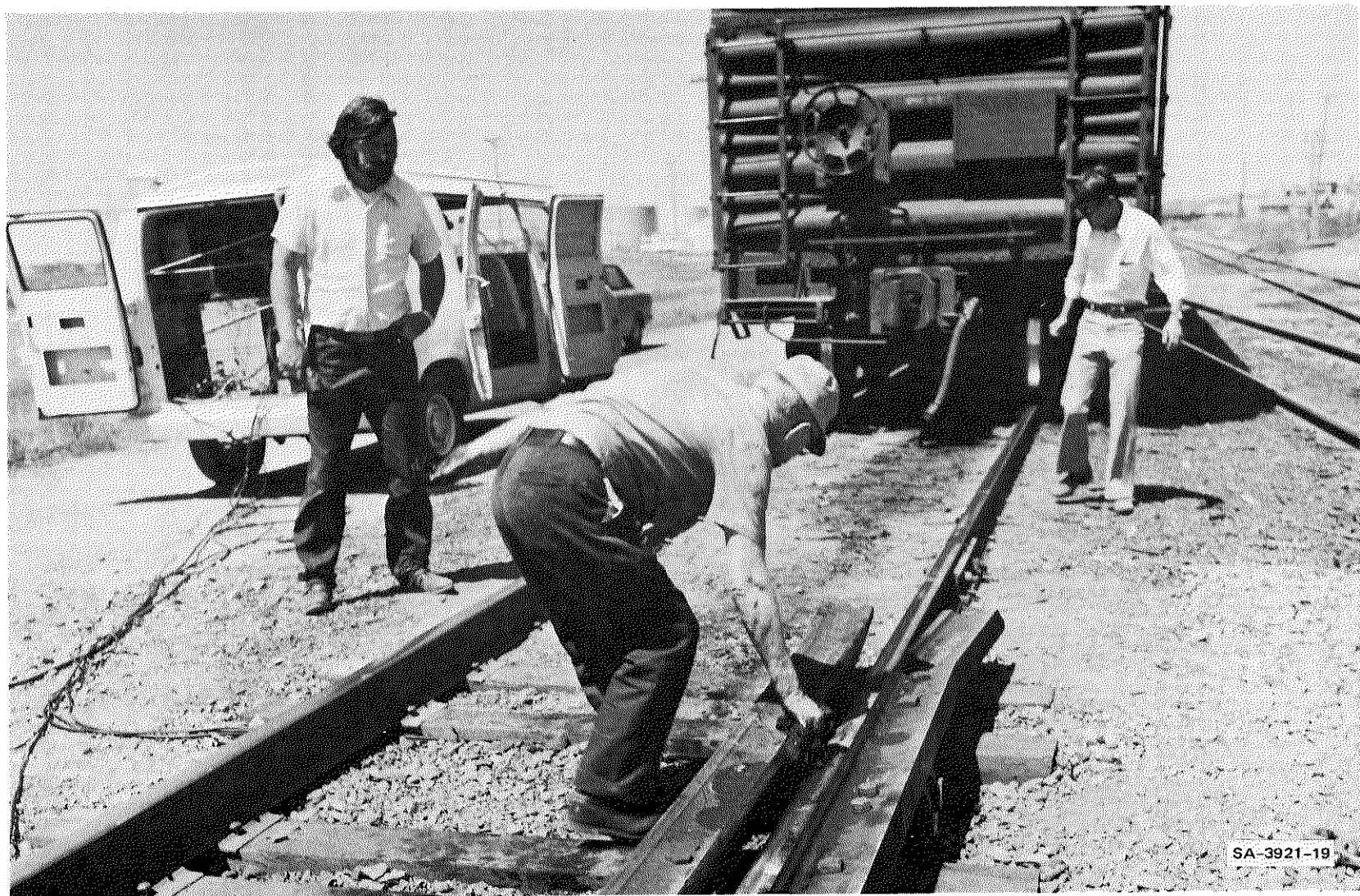
FIGURE X-1 GREASING THE INSTRUMENTED RETARDER SHOES
