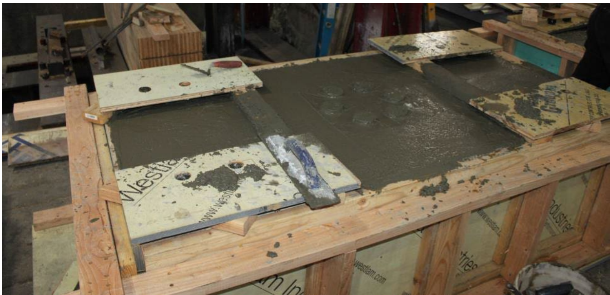
Figure 2.17 Footing concrete casting
