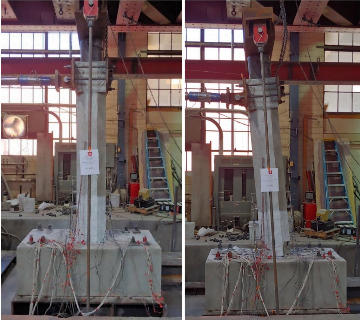
Figure 2.27 Experimental configuration for column test
