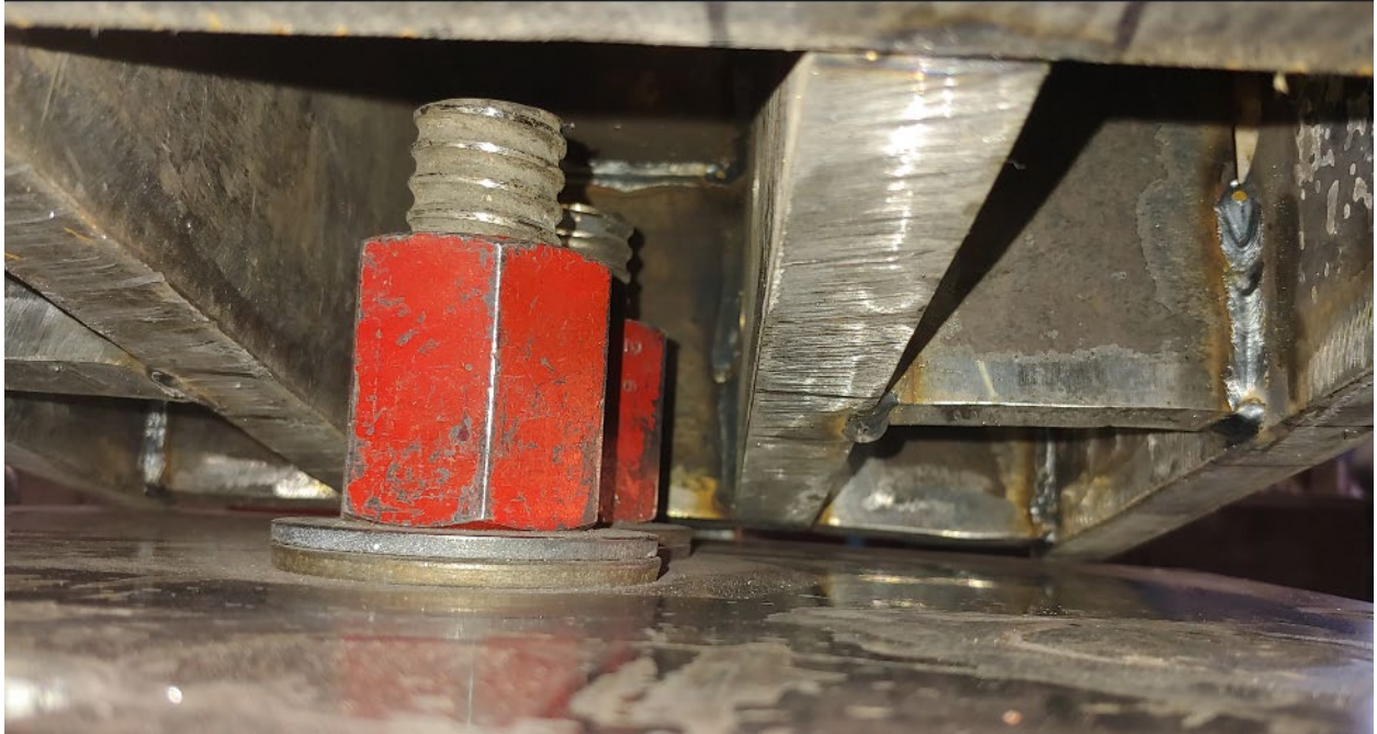
Figure 2.22 PT bars were nested inside the custom steel box
