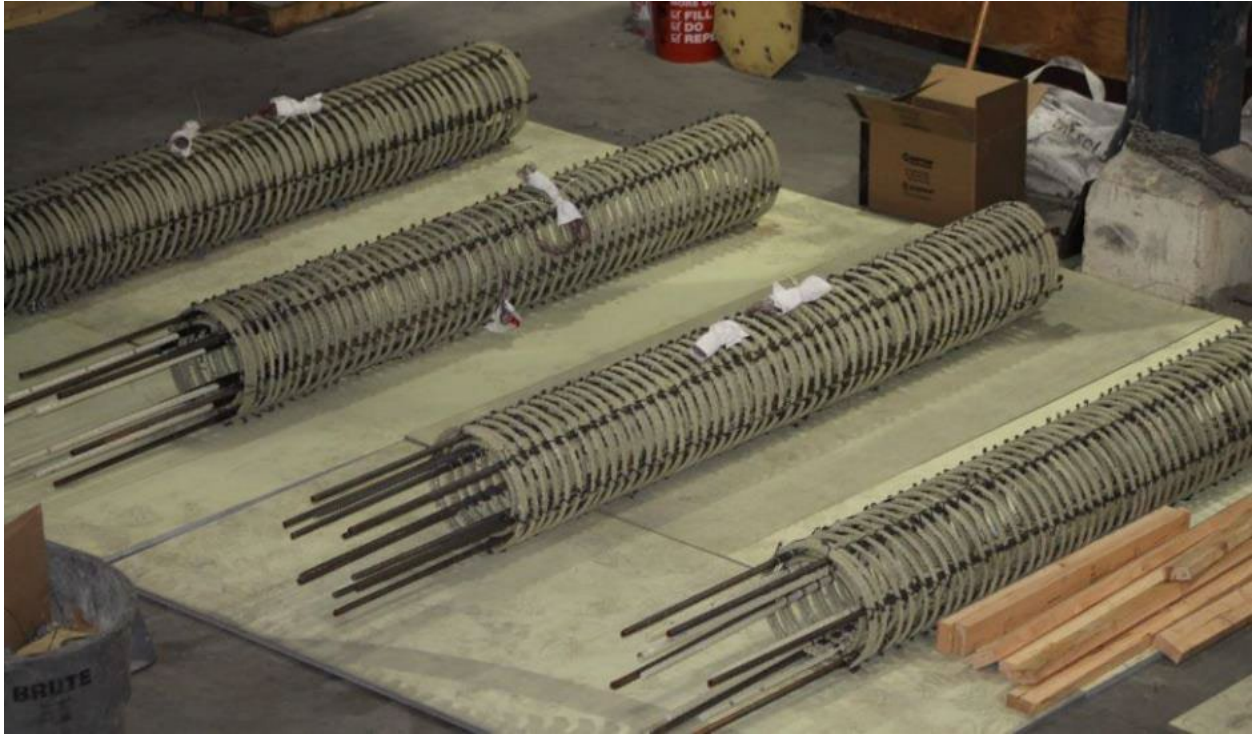
Figure 2.12 Column reinforcement cages
