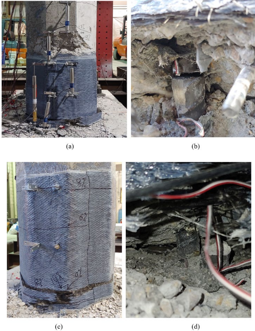
Figure 3.4 PT column damage: (a) PT-HYB column overall damage at 12% drift ratio; (b) PT-HYB column steel bar fracture at 12.0% drift ratio; (c) PT-STL column overall damage at 12% drift ratio; and (d) PT-STL column steel bar fracture at 12.0% drift ratio
