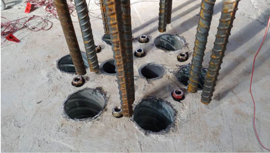
Figure 2.18 Nuts were used as spacers to create the grout bed
