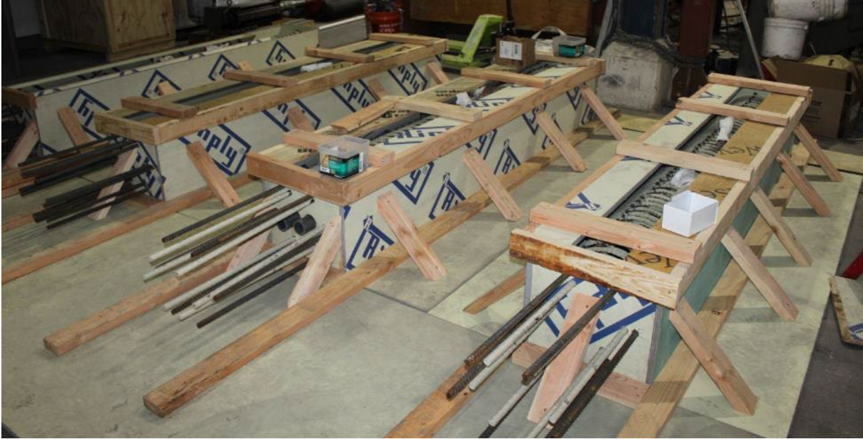
Figure 2.14 Column concrete casting formwork
