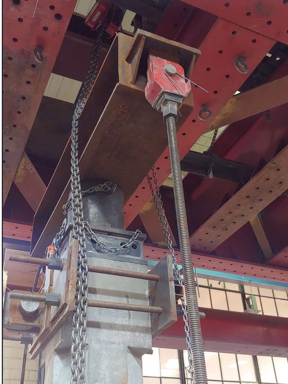
Figure 2.23 The complete top setup of the axial load for PT columns
