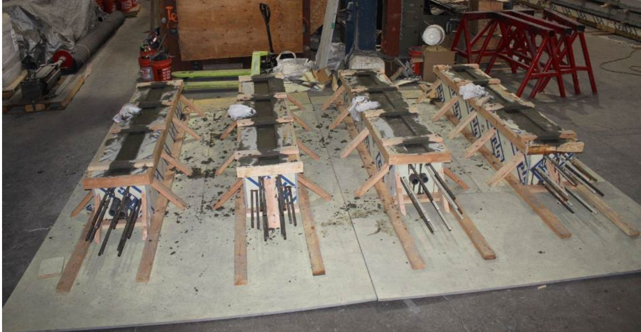
Figure 2.16 Column concrete casting
