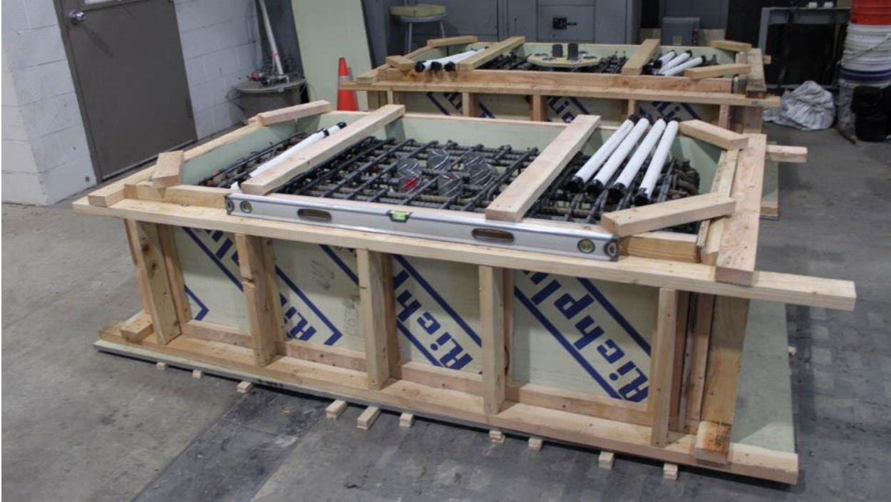
Figure 2.15 Footing concrete casting formwork
