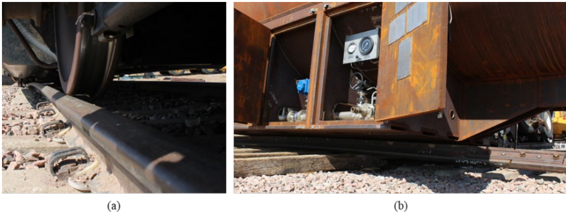
Figure 29. Rolled Rail Under (a) the East-side Locomotive and (b) the South-side LNG Fuel Tender Housing (Non-impacted Side)
