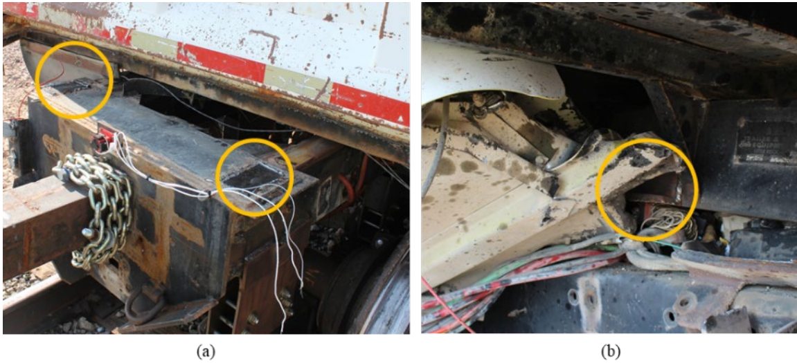
Figure 26. Failed Welds Between Dump Bed and Underframe at (a) the Rear Hinges and (b) the Angle Iron Shown in Figure 8(a)
