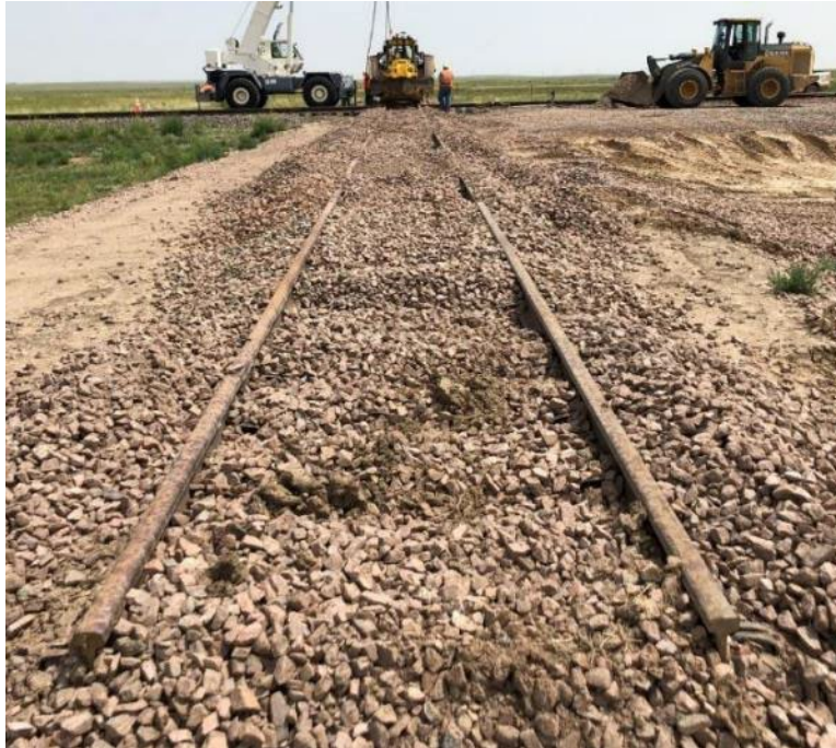
Figure 11. Track Section Under Construction (West View)
