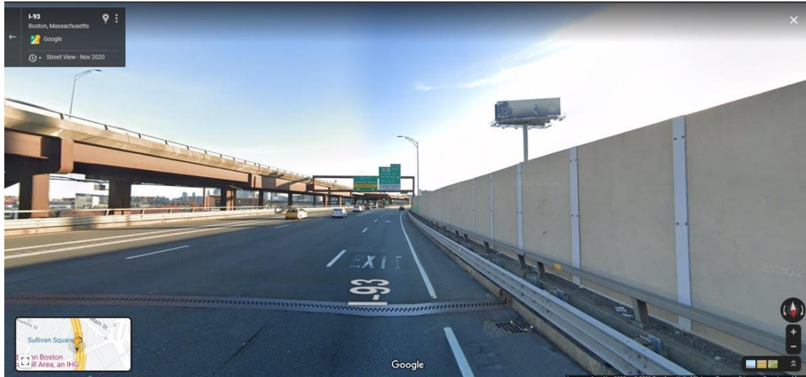
Figure 3.4: An example of Google Street View of OIP location
