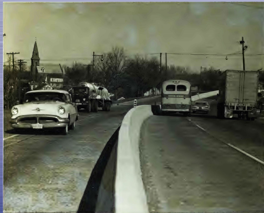
New 32" high solid concrete center barrier being installed on Route 46 in Leonia and Fort Lee.
