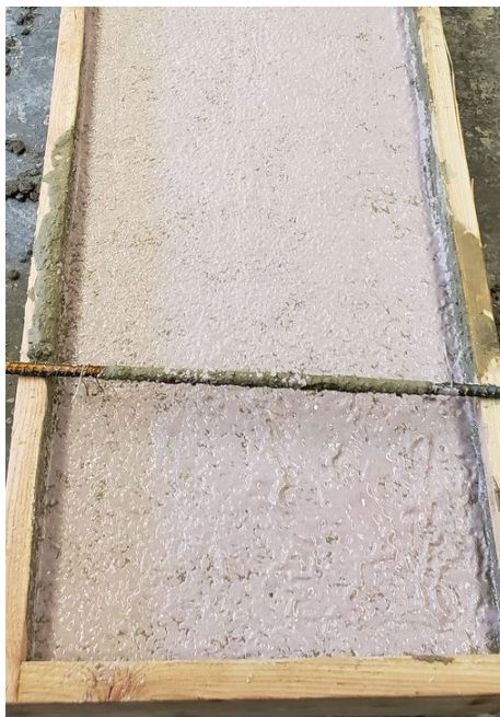
a) After surface retarder applied
