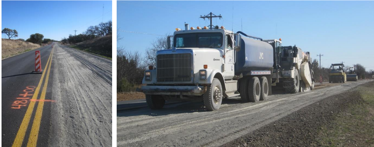
Figure 39. Cement Treatment on FM 205.
