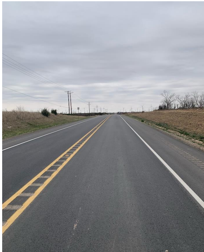
Figure 37. Completed US 180 Project.
