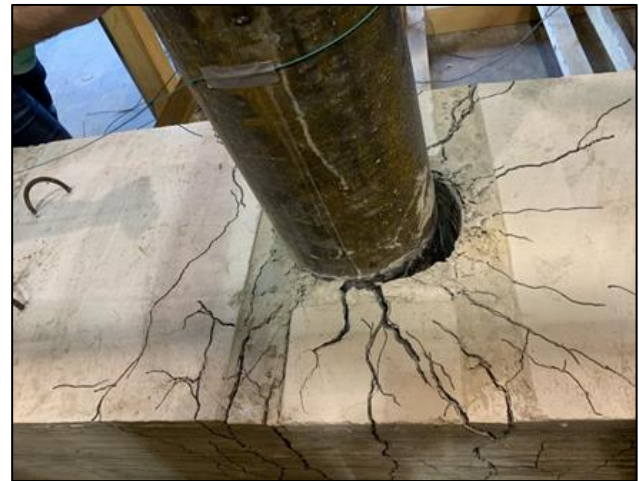
Figure 44: VT2/3-6 failure from reverse loading direction
