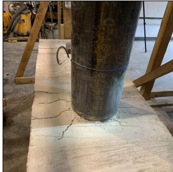
Figure 48: VT2/3-4U 45-degree cracks (184 k-ft)
