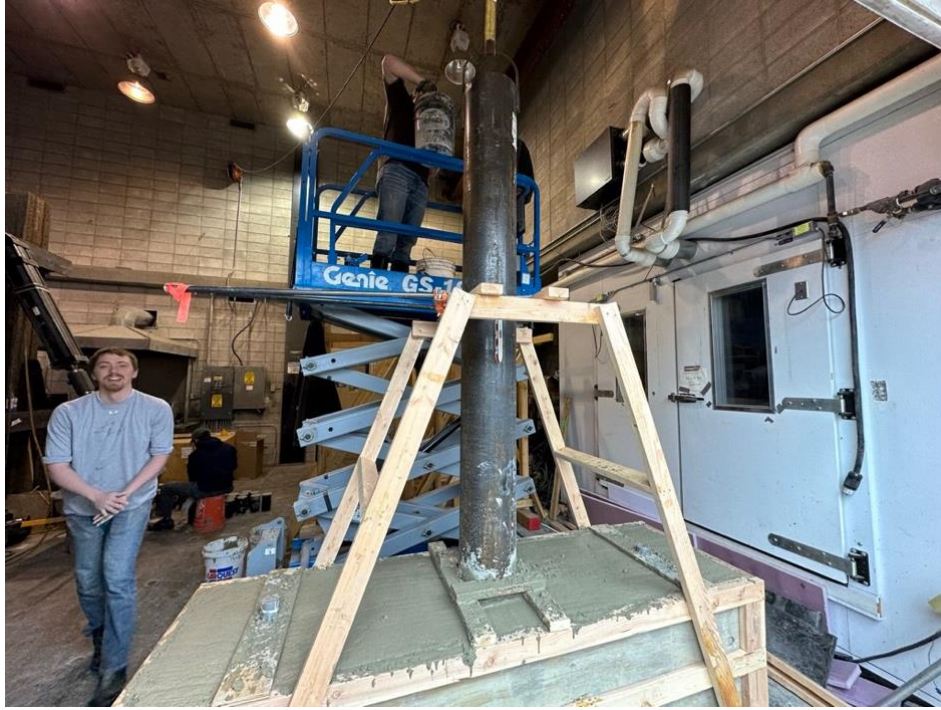
Figure 21: Filling CFST with Concrete
