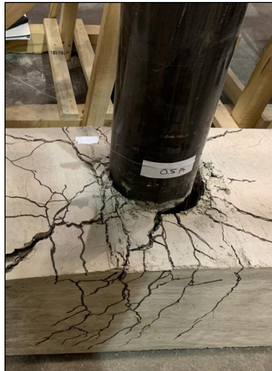
Figure 29: VT1/2-4 failure from reverse loading direction
