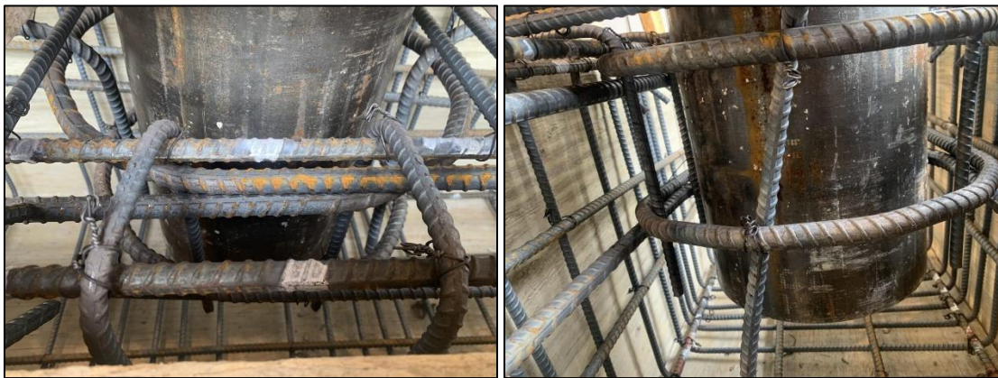
Figure 17: U-Bar placement in VT2/3-4U
