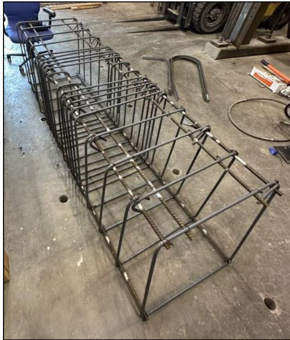
Figure 18: Reinforcing cage under construction
