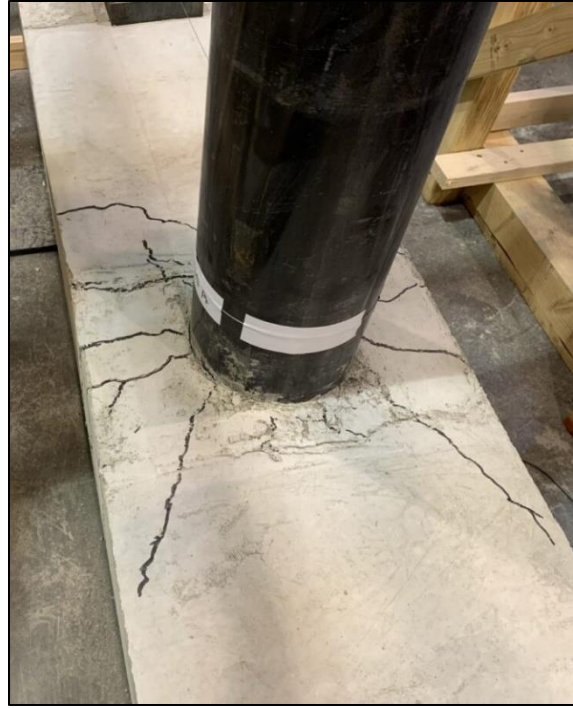
Figure 27: VT1/2-4 45-degree cracks (63 k-ft)
