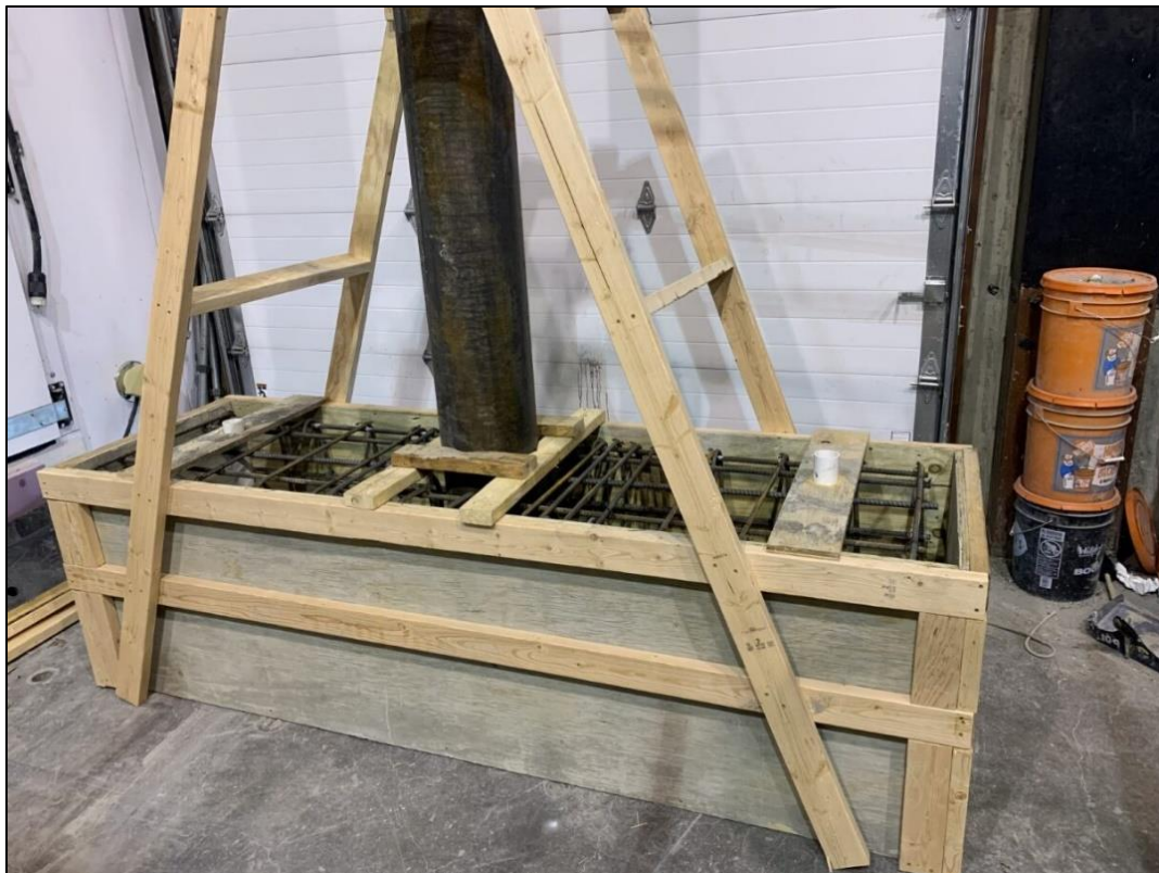
Figure 19: Full specimen setup before concrete pour
