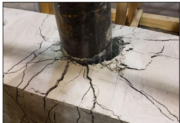
Figure 38: VT2/3-4 failure from reverse loading direction
