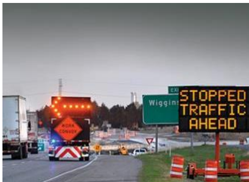
(c) Construction work zones (Source: FHWA.gov)
