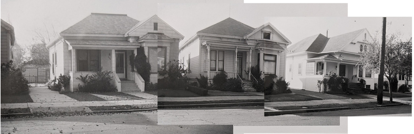
A composite photo created to show a street-level, mid-block perspective of homes that were demolished. L to R: 451, 449, and 441 Delmas Ave. Original photos from Caltrans Right of Way Assessments 1960 - 1970 archival collection, San José Public Library.
