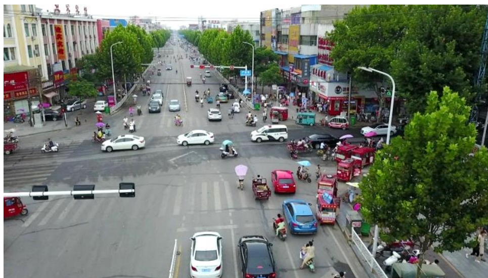
Figure 4. The intersection used in the case study.
