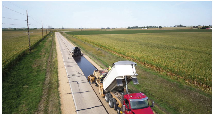
Otta seal construction
