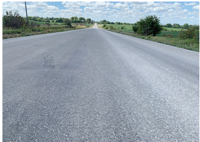
Otta seal on test site TS-2 one month after construction
