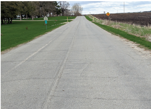
Buchanan County Otta seal site built in July 2018 (photo taken April 2023)
