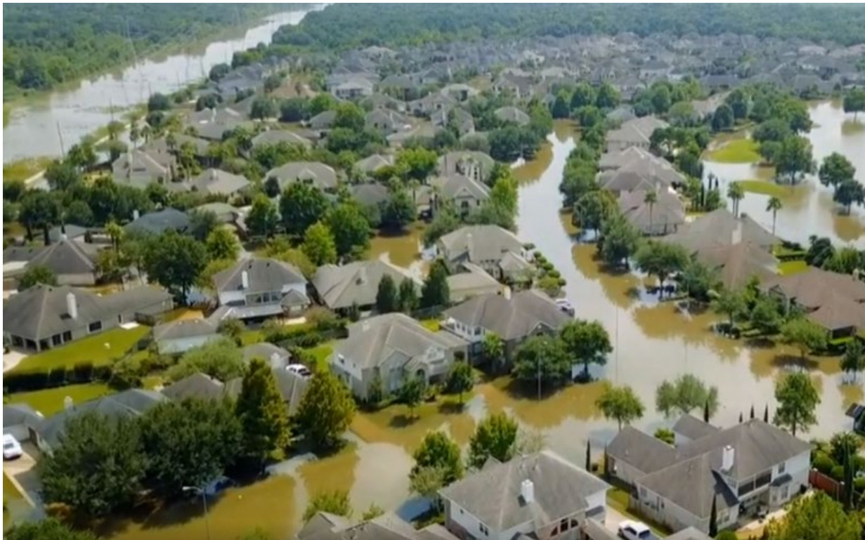
Figure 7. UAS Assessment of Flood Damage in Texas. (Image Fort Bend County Office of Emergency Management)
