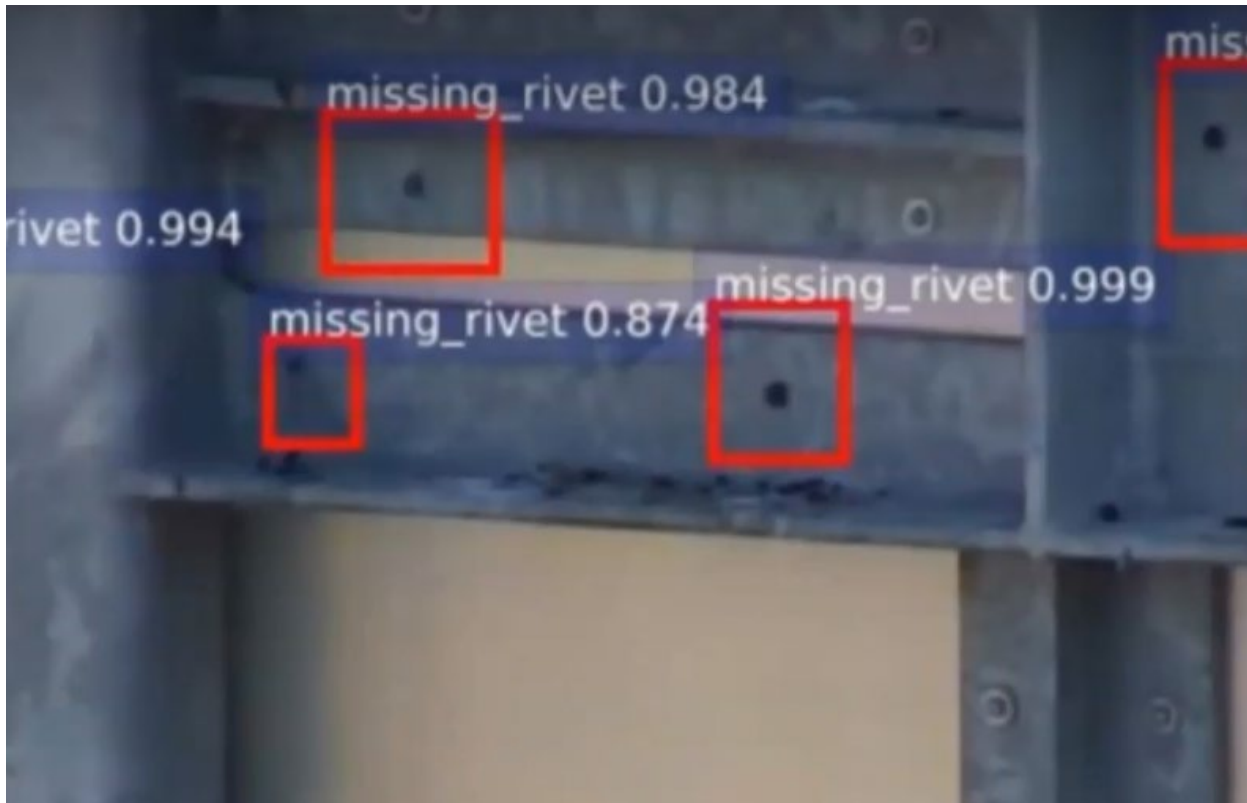
Figure 24. Example of Machine Learning Report for Overhead Sign Inspections (Source: UDOT)
