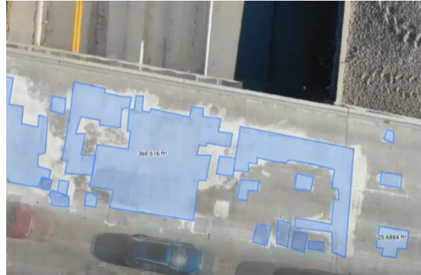
Figure 12. UAS Mapping Bridge Decks (Source: UDOT)
