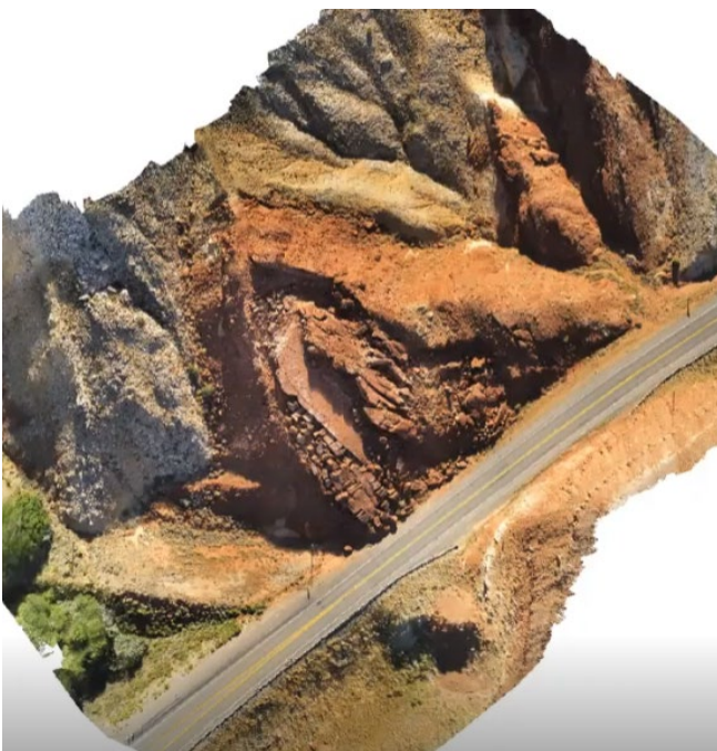
Figure 7. UAS-Collected Data Point Cloud (Source: WYDOT)
