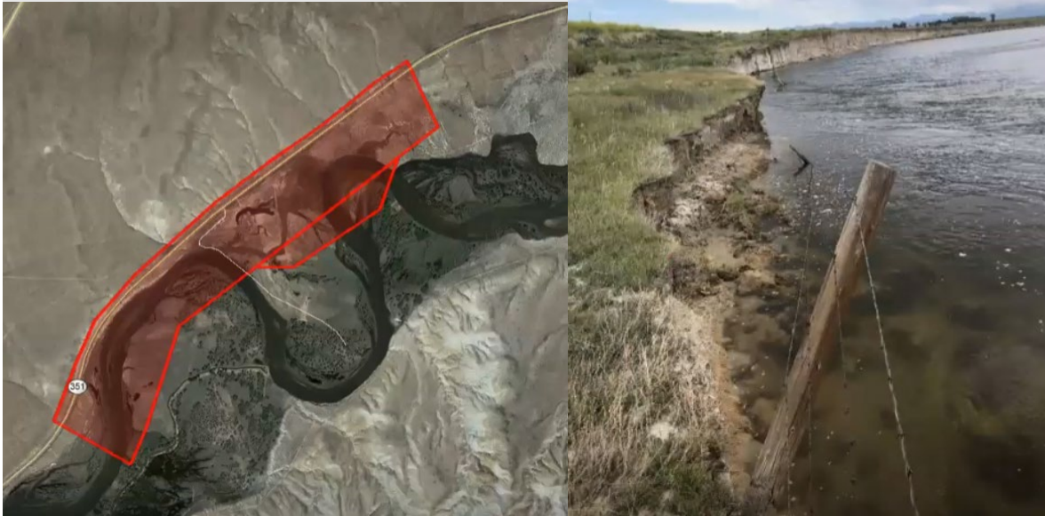
Figure 8. Survey Area of the Big Piney Cutoff and Riverside View of Erosion (Source: WYDOT)
