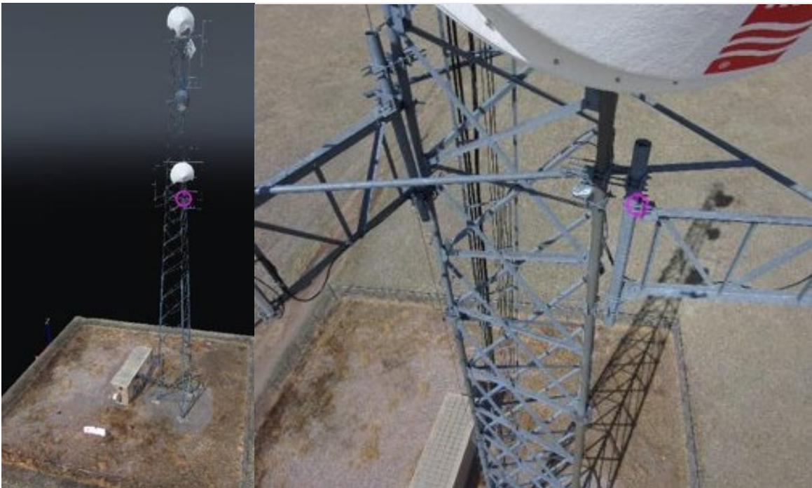
Figure 1. UAS-Collected Data Creates 3D Model of WYOLINK Communications Tower (Source: WYDOT)
