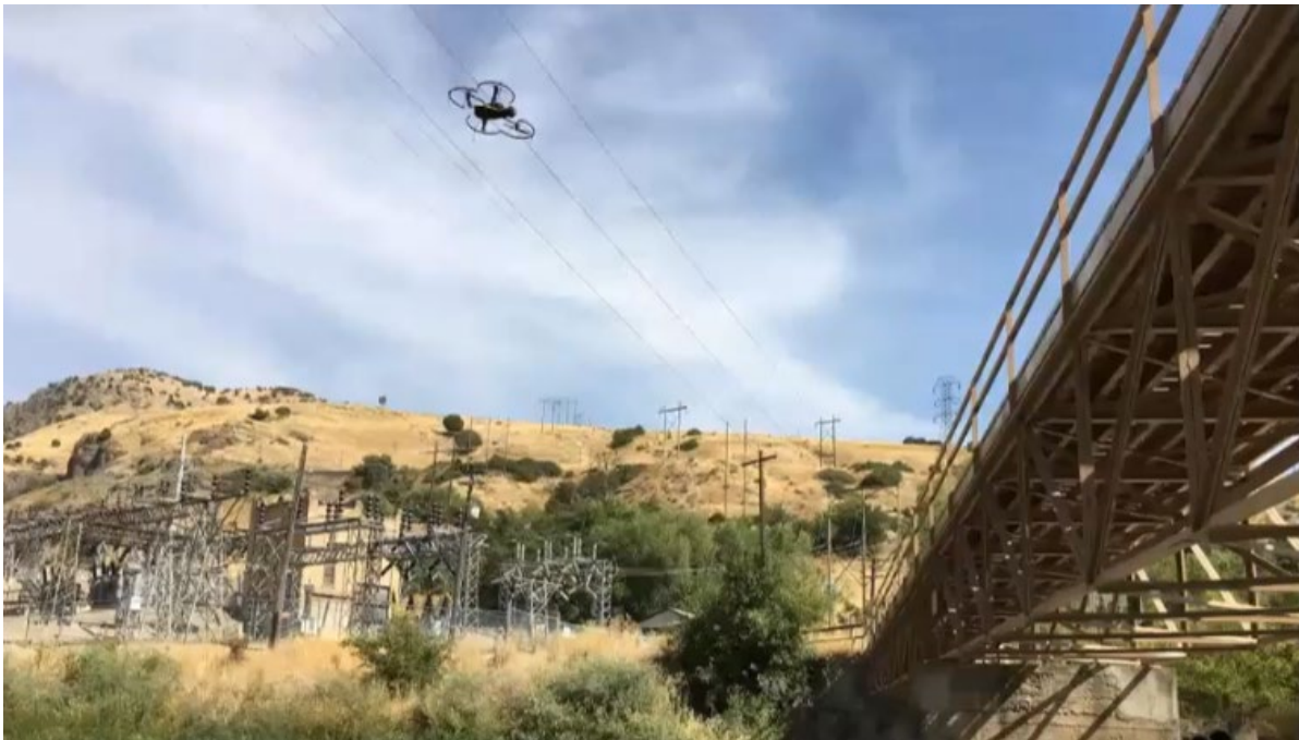
Figure 11. Utah Bridge Inspectors using UAS on a Routine Bridge Inspection (Source: UDOT)
