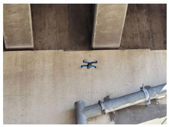
Figure 5. CDOT UAS on Bridge Inspection. (Source: CDOT)
