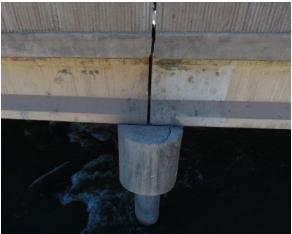
Figure 18. Cracked Substructure Support on Large Figure 19 Bridge. (Source: UDOT) Deck. (Sc
