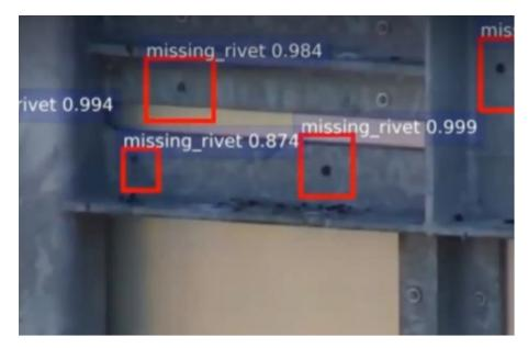
Figure 22. Machine Learning Detecting Mission Rivets on UAS Collected Data. (Source: UDOT)
