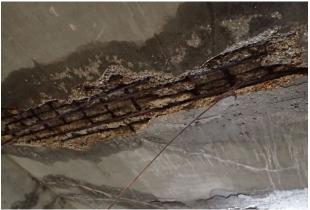
Figure 12. Deteriorating Culvert Infrastructure. (Source: NMDOT)
