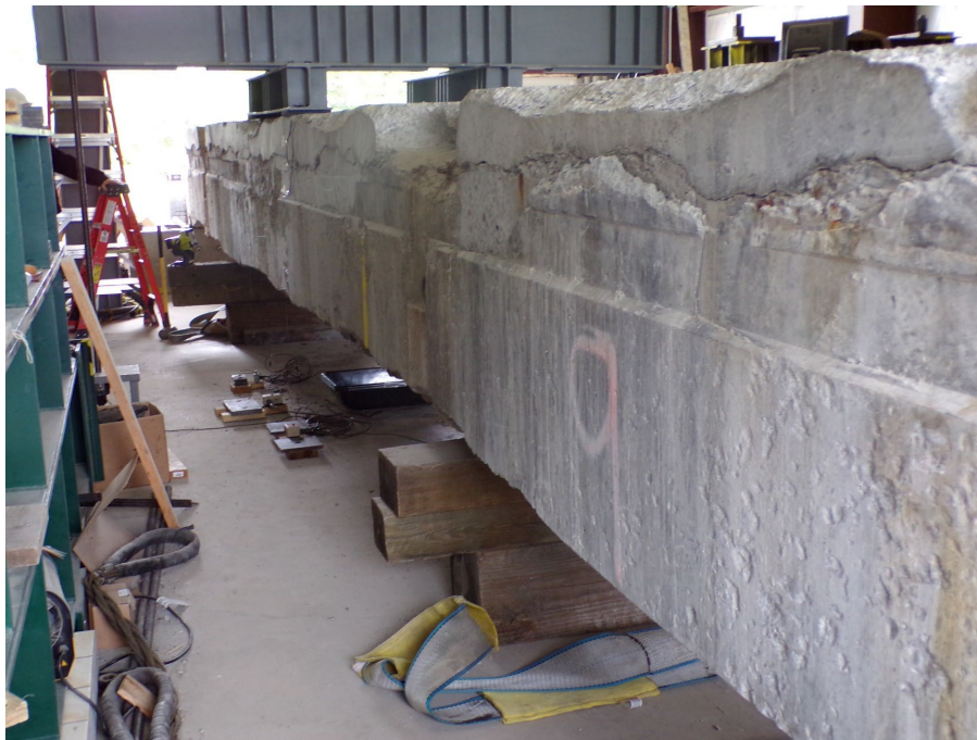
Figure 4.25: Concrete patching along top of Specimen E9
