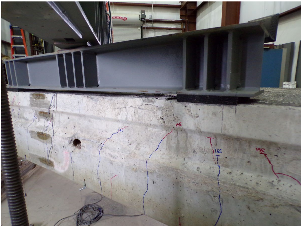
Figure 5.12: Cracking of Specimen R3 at concrete crushing (northwest load point)
