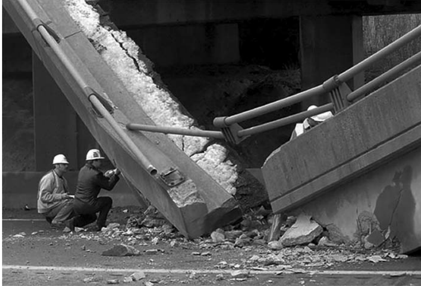
Figure 2.1: Lake View Bridge collapse
