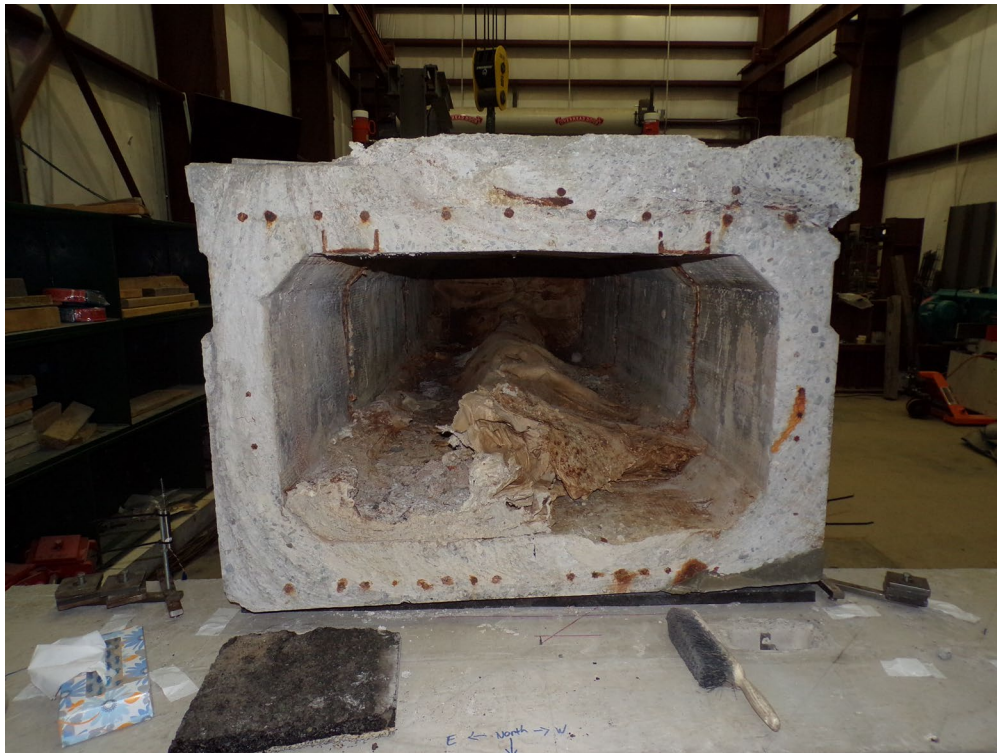
Figure 4.21: North end of Specimen E3
