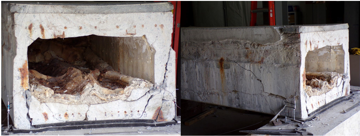
Figure 5.22: South end failure of Specimen E4
