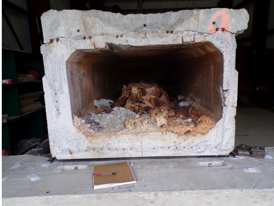
Figure 4.24: North end of Specimen E9
