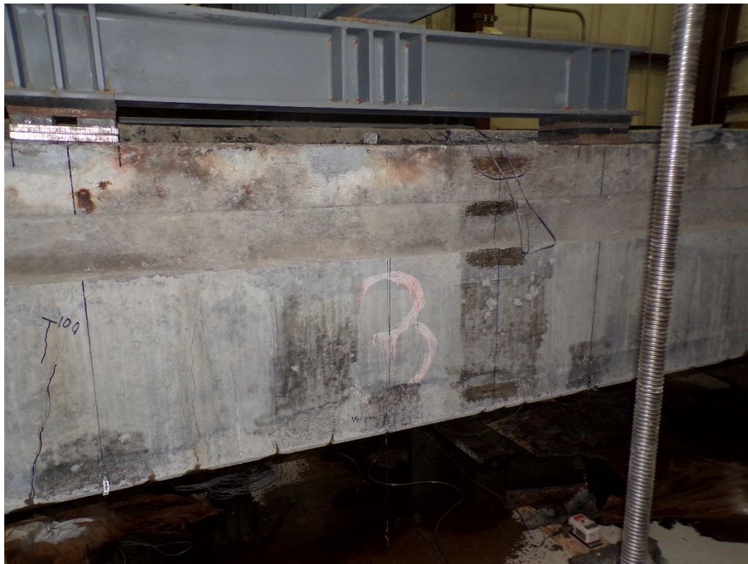
Figure 5.25: Flexural cracking of Specimen E3 and water leakage
