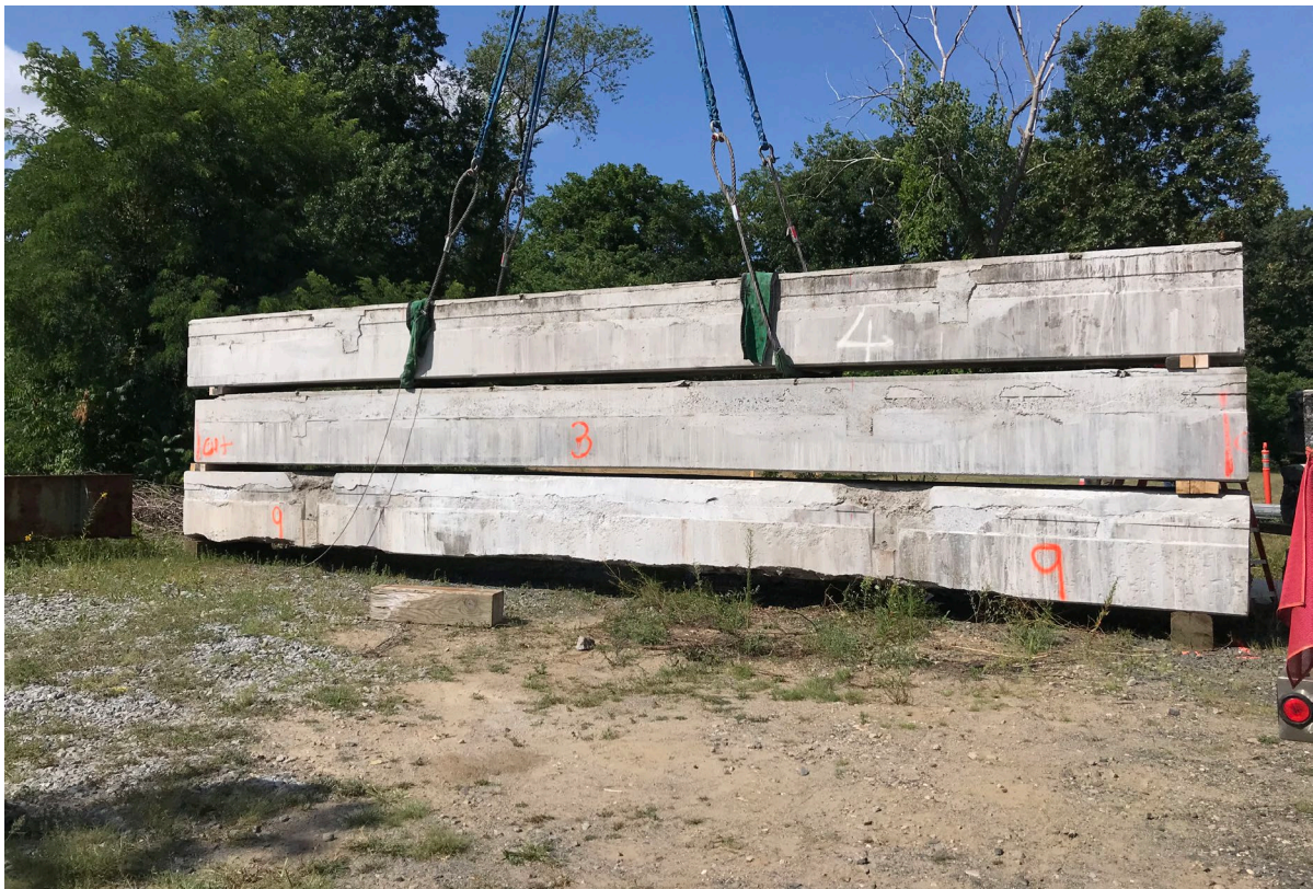
Figure 4.9: Essex Bridge beams at the Brack Structural Engineering Laboratory
