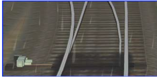
Figure 22. Close-up of Track Split Setting
