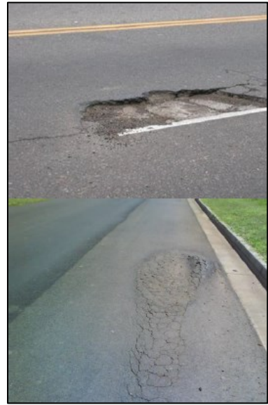
Damages to the flexible pavements due to weak geomaterial and soil characterizations
