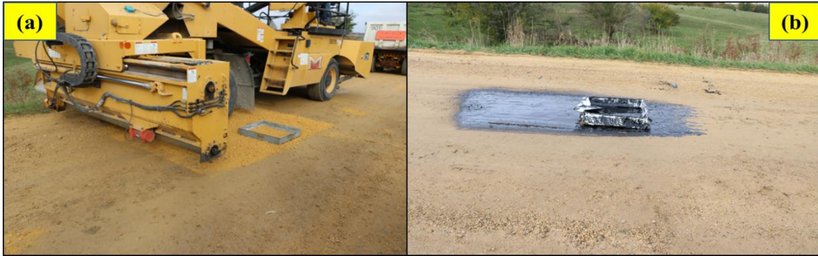
Figure A6. Calibration of (a) aggregate spreader and (b) asphalt distributor
