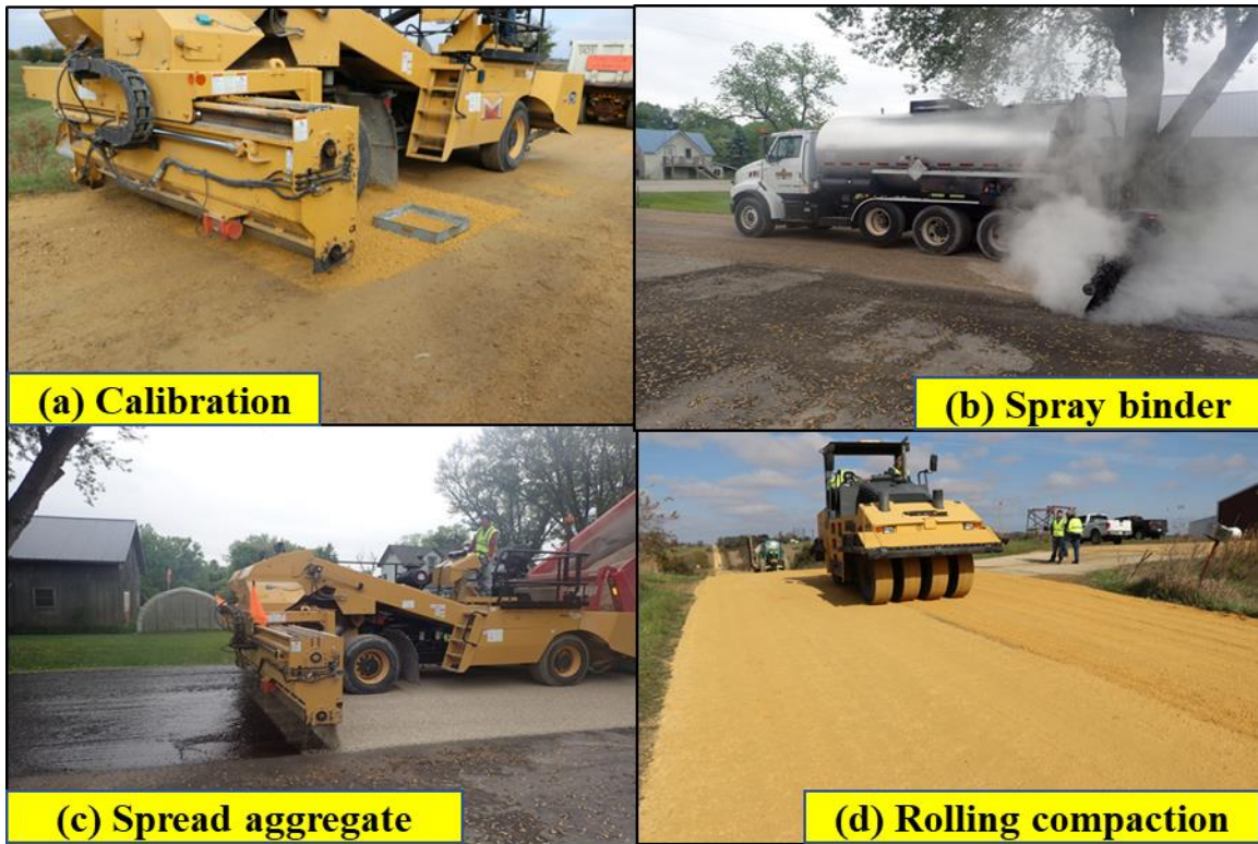
Figure 4. Typical Otta seal field construction procedures in Iowa
