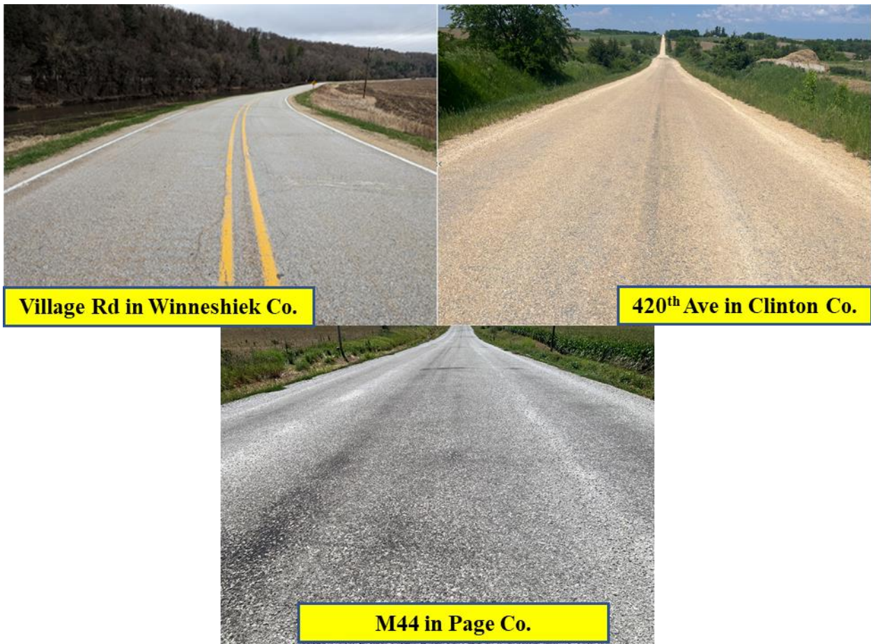
Figure B5. Otta seal site appearance in Winneshiek County (photo taken on April 21, 2023), Clinton County (photo taken on June 2, 2023), and Page County (photo taken on June 29, 2023)
