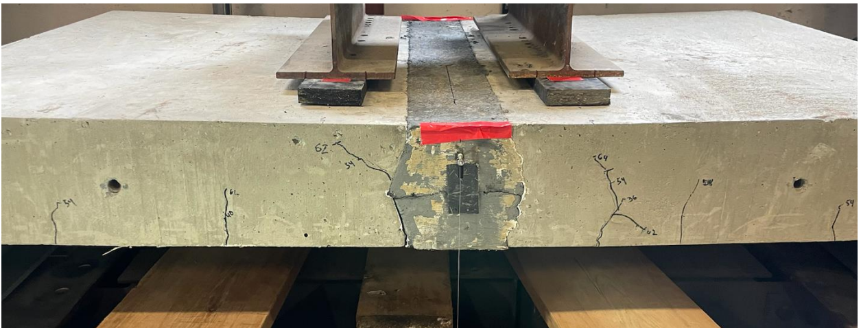
Figure 7.11: Initial cracking behavior of specimen 2
