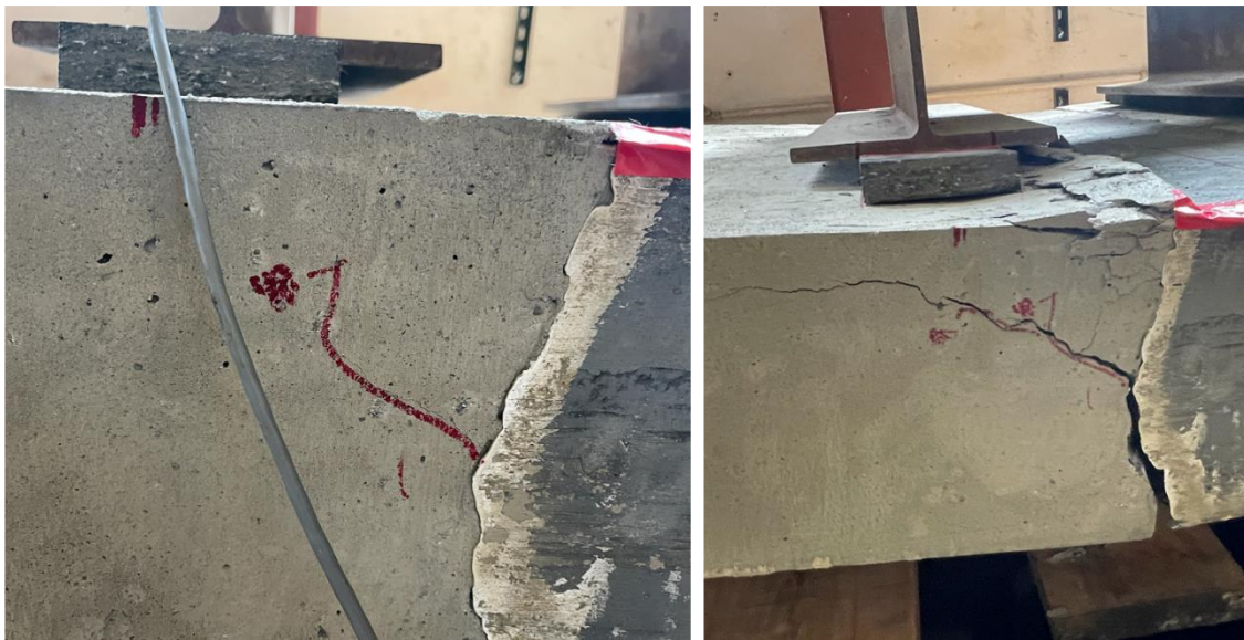
Left: 48 kips, Right: maximum load Figure 7.7: Crack from shear key of specimen 1
