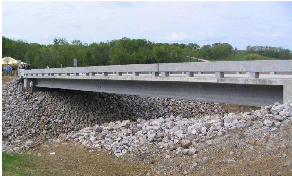
Figure 2.3: Mars Hill Bridge completed.
