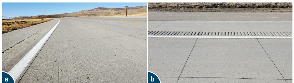
Figure 4. Current condition of the overlay: (a) close-up of pavement surface and edgeline and (b) edgeline, shoulder, and rumble strips
