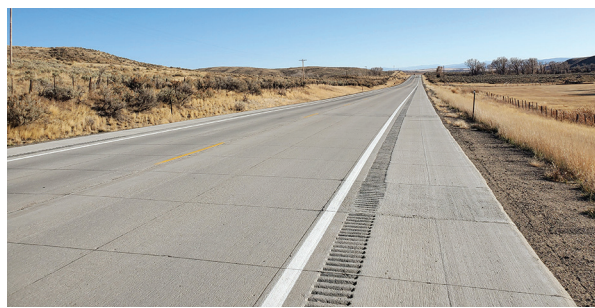
Figure 3. Completed concrete overlay on asphalt-bonded overlay
