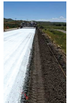
Figure 2. Asphalt millings placed on the shoulder
