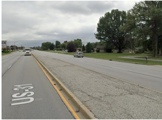
Figure 59. Photo. Roadway Raised Median
