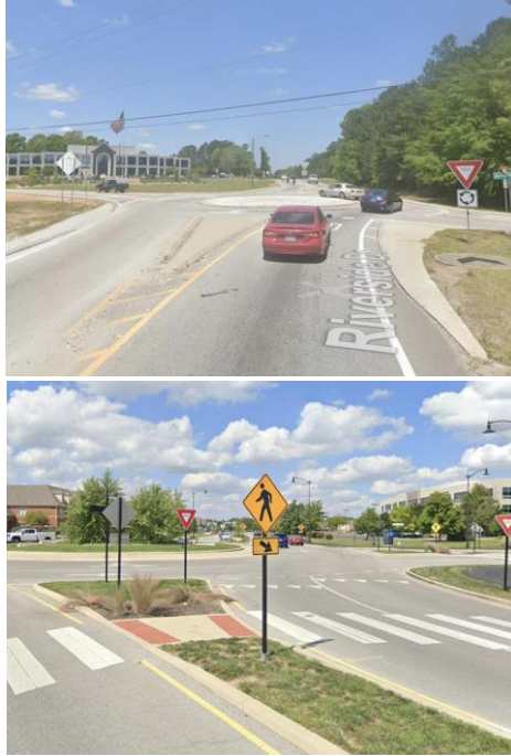
Figure 61. Photo. Approach Splitter Island (Left to right: Raised Splitter Island without a Crosswalk, Raised Splitter Island with a Depressed Crosswalk)
