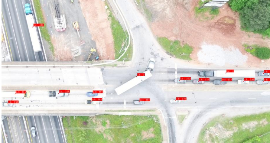
Figure 5. Photo. Overhead views of the four data collection locations at the selected truck stop
