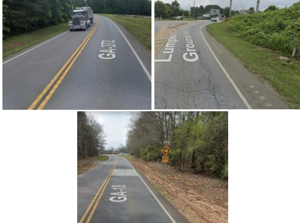
Figure 66. Photo. Rumble Strips. (Left to right: Centerline, Shoulder, Transverse Rumble Strips)
