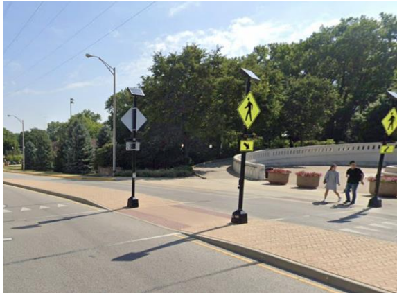
Figure 64. Photo. Pedestrian Refuge Island
