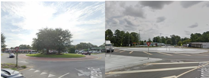
Figure 62. Photo. Central Island (Left to right: Raised Central Island with Plants, Raised Central Island with Chevron Signs)
