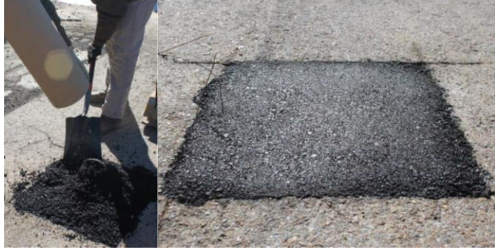
Figure 23. Field repair of pothole using induction heating (59)
