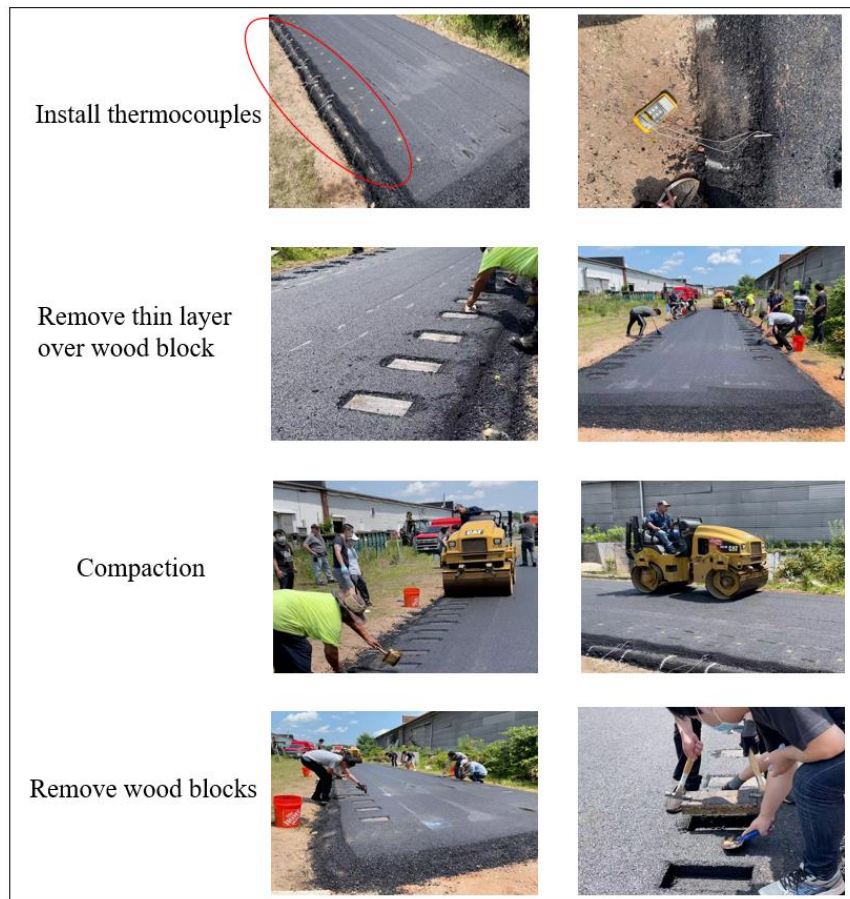
Figure 35. Second layer construction
