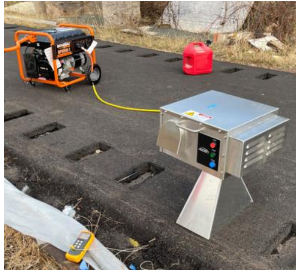
Figure 41. The second heating test
