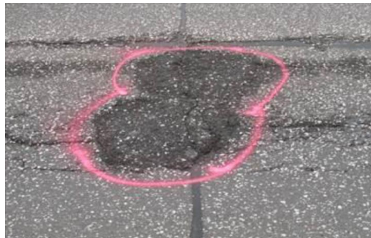
Figure 20. Microwave repaired pothole (5)
