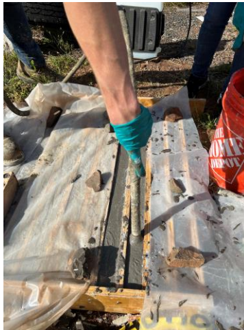
Figure 18. Vibrating the layers of concrete
