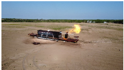
Test in Progress (PRV operating)
