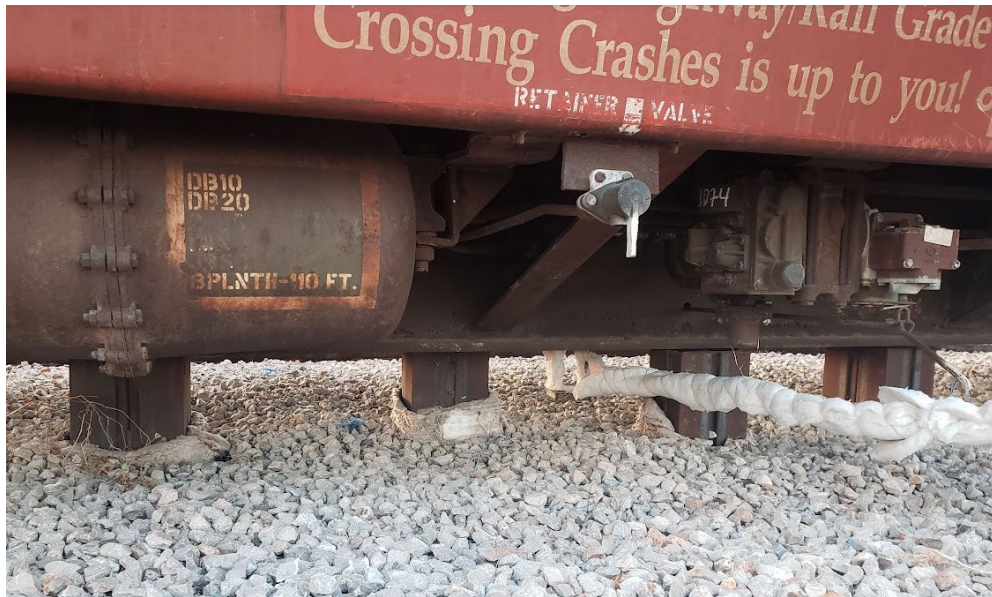
Figure 7. Structural Steel Pilons Installed to Support the Flatcar During the Test
