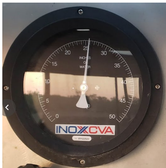
Figure 36. Liquid-level Gauge on Tank Indicating ~25.9" H 2 O 1 H Prior to Test
