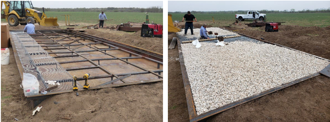
Figure 9. Phase 2 Propane Test Burner Photographs
