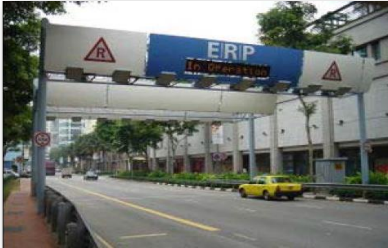
Electronic Road Pricing Gantry at North Bridge Road, Singapore
