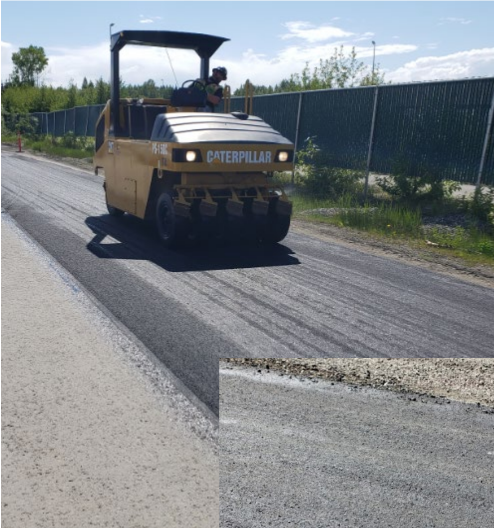
A mask on the micro surfacing test strip after the roller has made its passes and it has set.
