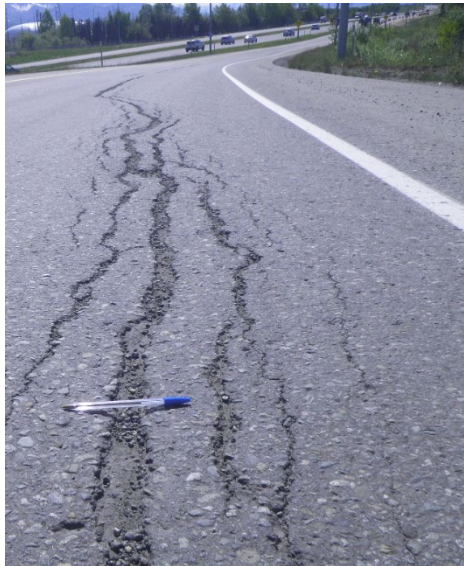
Ramp 1 Prior to Surface Preparation
