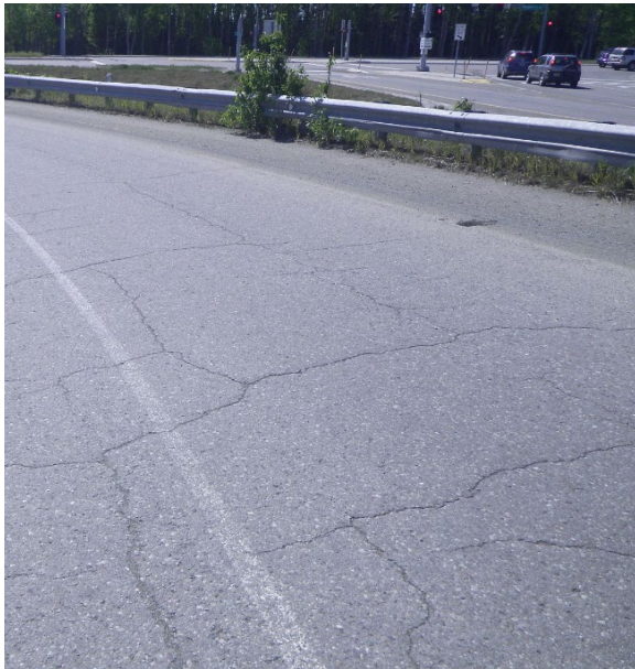
Photo 1 - Ramp 8 General Condition
