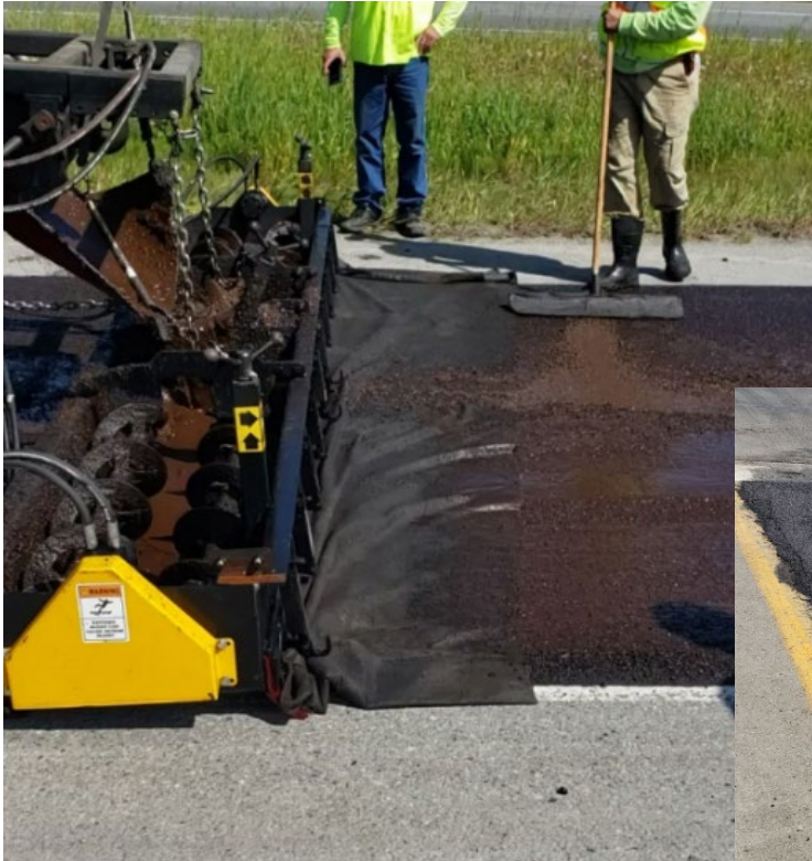
Photo 2 - Secondary Strike Off and Hand Working
