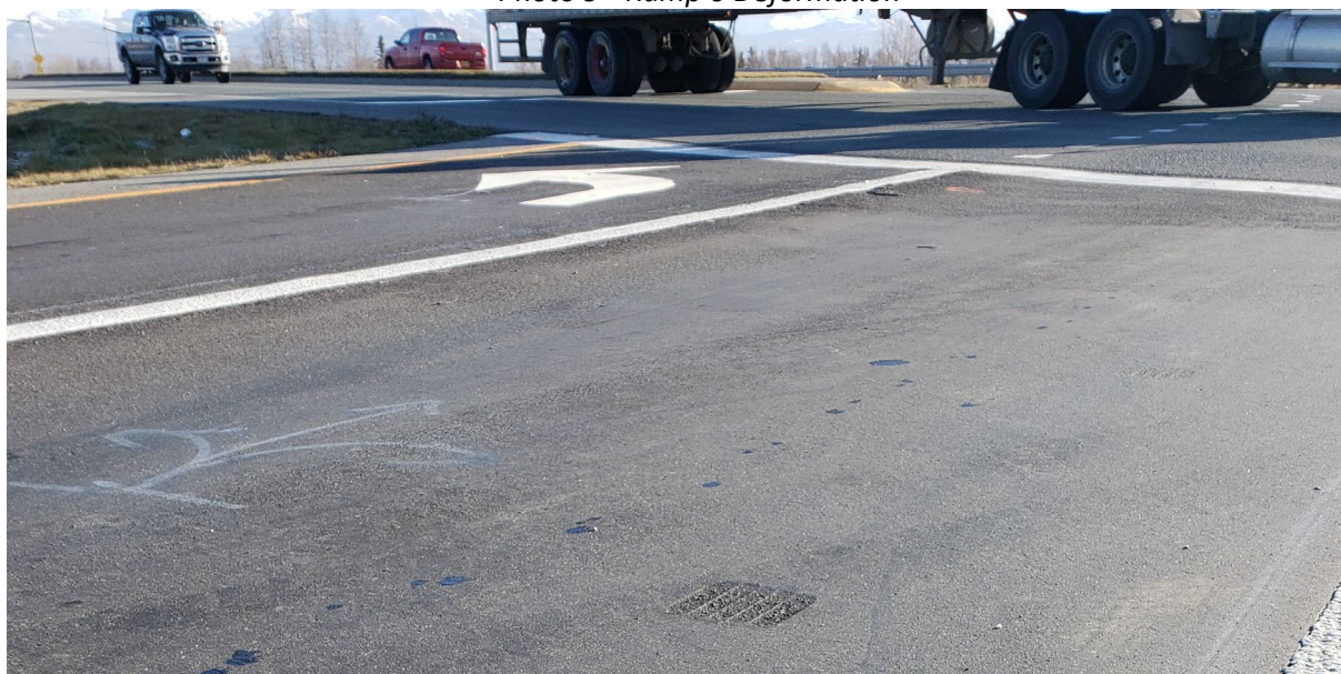
Photo 9 - Ramp 6 Deformation
