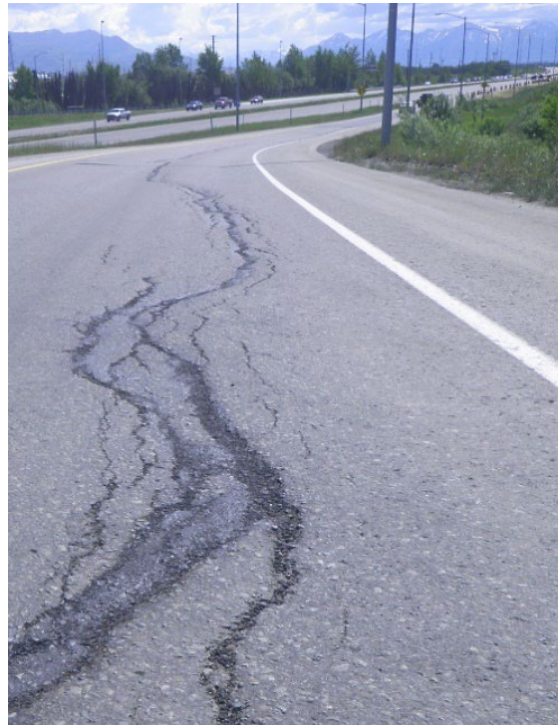
Ramp 1 After Surface Preparation
