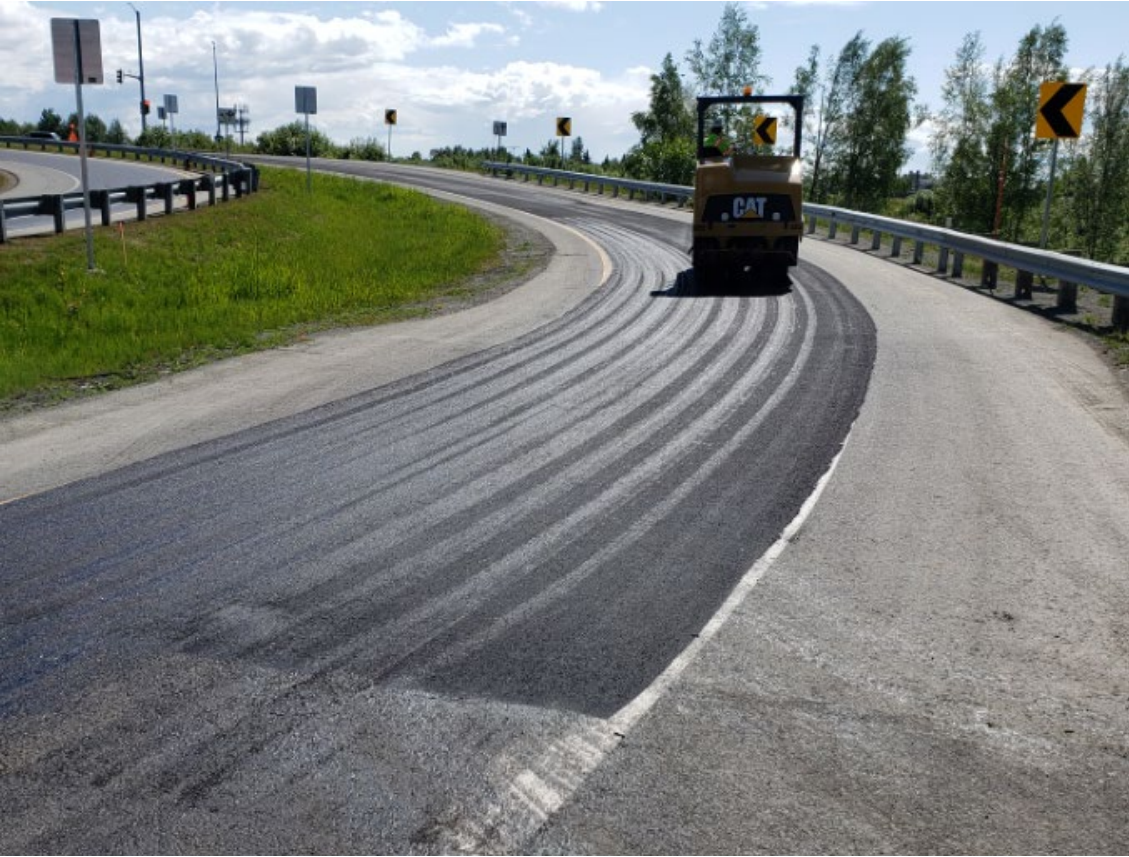
Hand worked areas on the scratch course on Ramp 3 on the fourth day of production.
