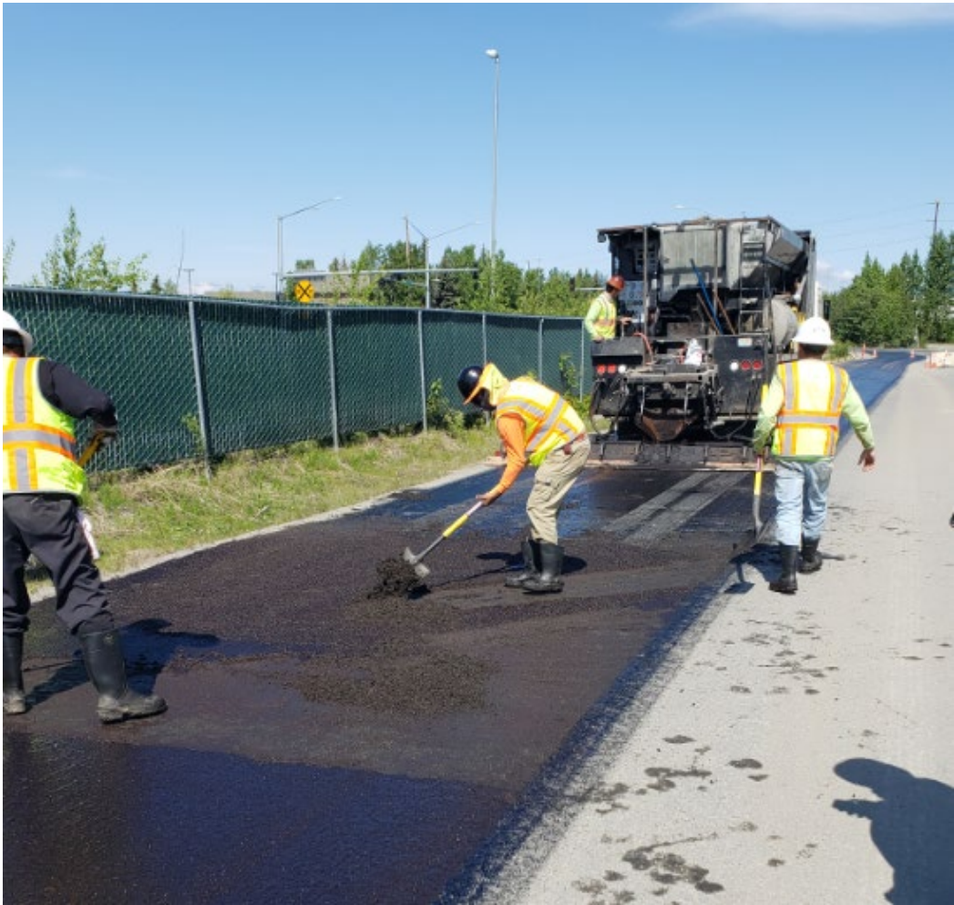
Micro surfacing slurry as it is setting on tack coated pavement
