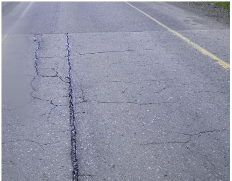
Photo 2 - Ramp 9 General Condition
