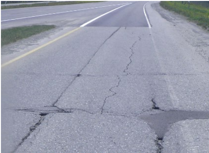
Photo 3 - Ramp 11 Prior to Surface Preparation
