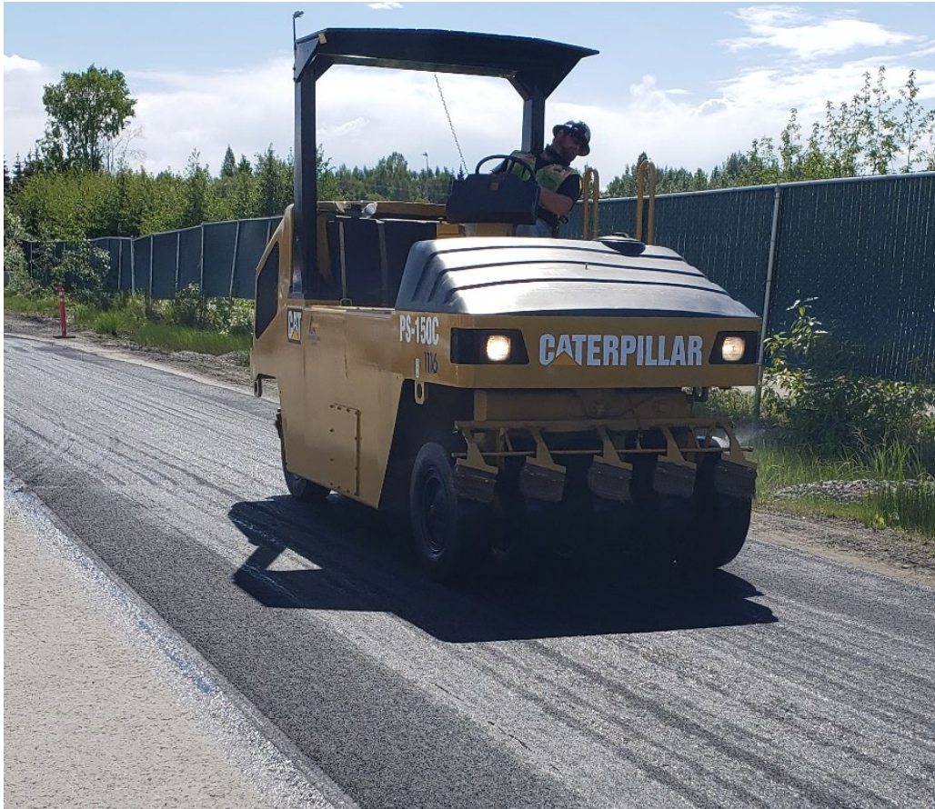
Photo 4 - Pneumatic Roller on Test Strip
