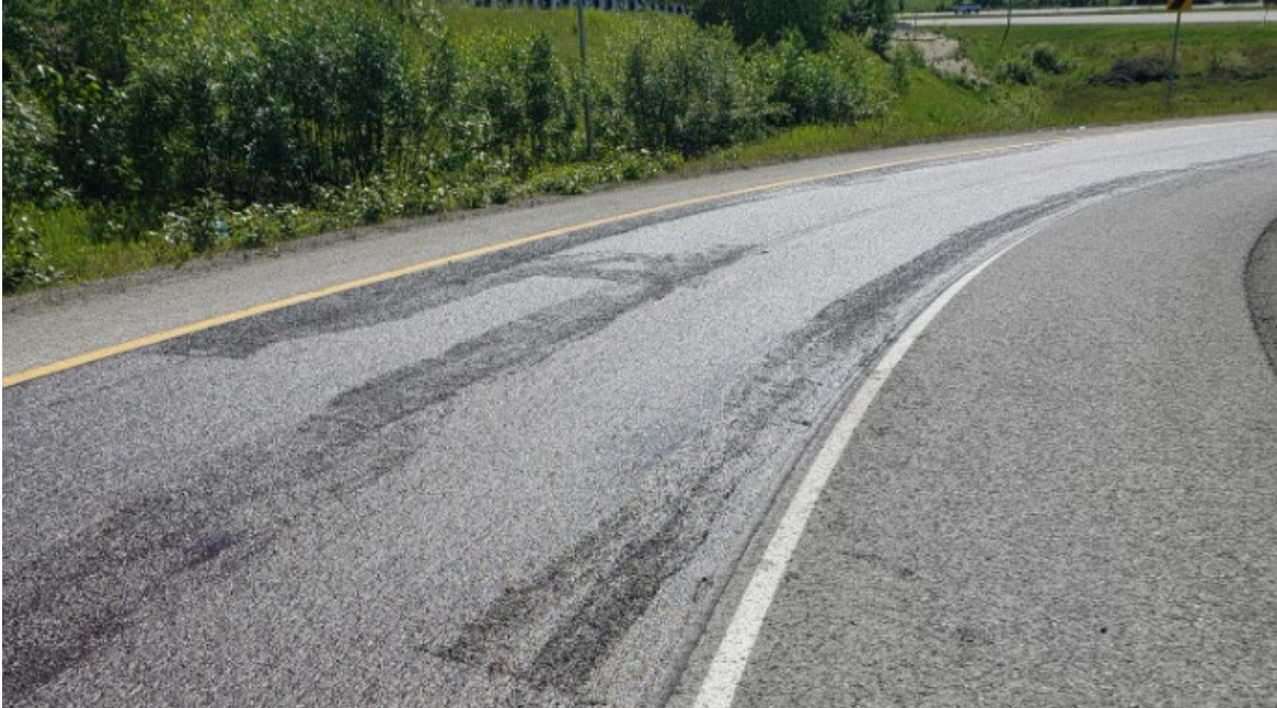
Hand worked areas on the scratch course on Ramp 3 on the fourth day of production.
