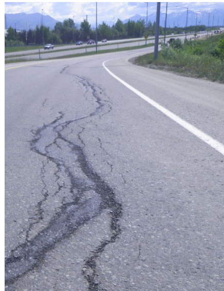
Ramp 1 After Surface Preparation
