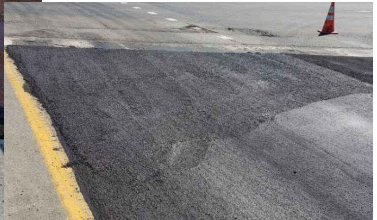
Photo 3 - Hand Worked Area on Ramp 6
