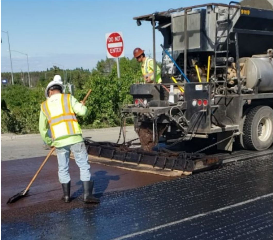
Scratch course placed on Ramp 5 prior to stopping production.
