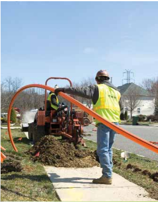
FIBER OPTIC CABLE INSTALLATION
