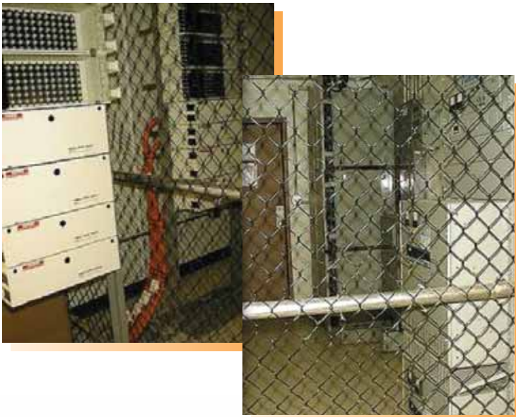
FIGURE 6: REGENERATION BUILDING – INTERIOR
