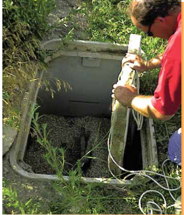
TYPICAL HANDHOLE OR ACCESS POINT
