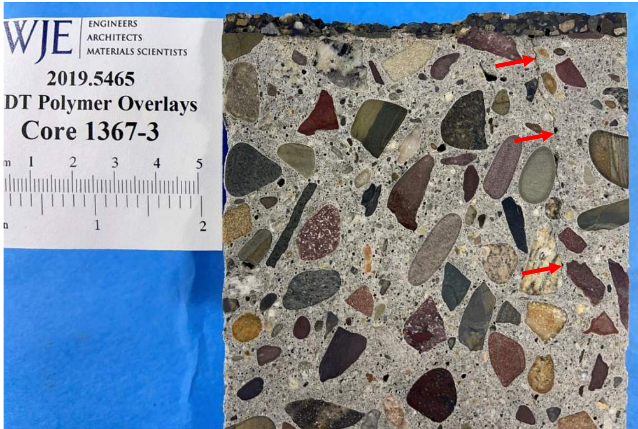
Figure C.1. Core 1367-3. Lapped cross section shows the overall appearance of the PPC overlay and top ~4 inches of the substrate concrete. Arrows indicate a vertical crack, further shown in the figure below.
