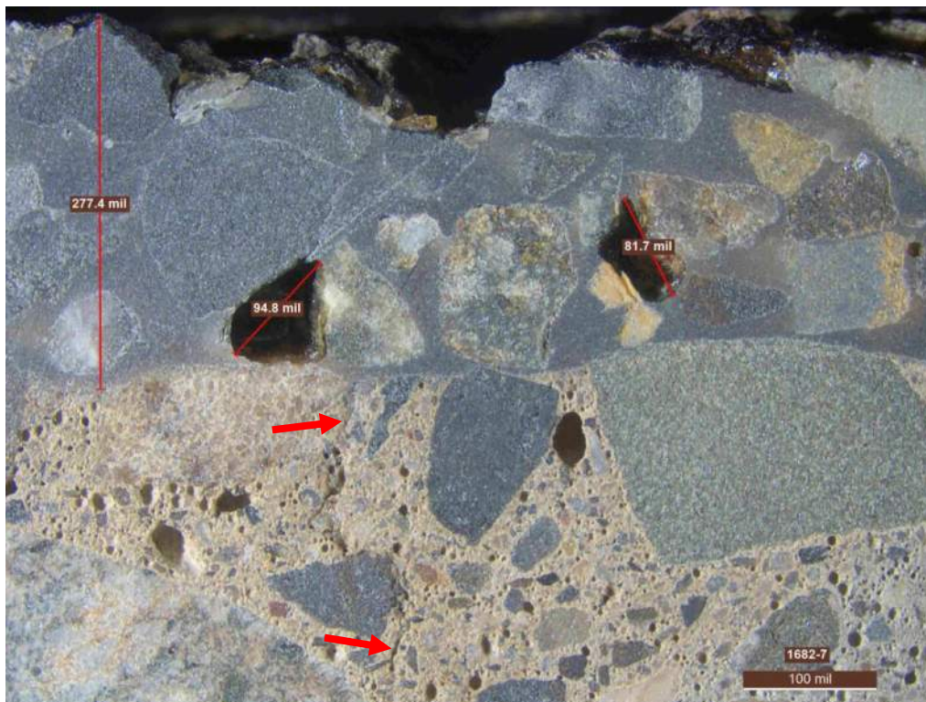
Figure C.18. Core 1682-7. Close-up views show the PPC overlay, a barely visible vertical crack and paste discoloration likely due to carbonation along the crack.
