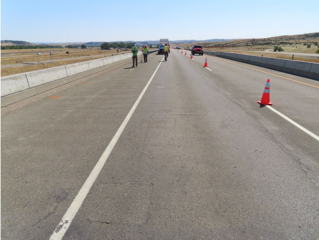
Figure 10. Overview of the driving lane and shoulder for Bridge 1670 in 2020.
