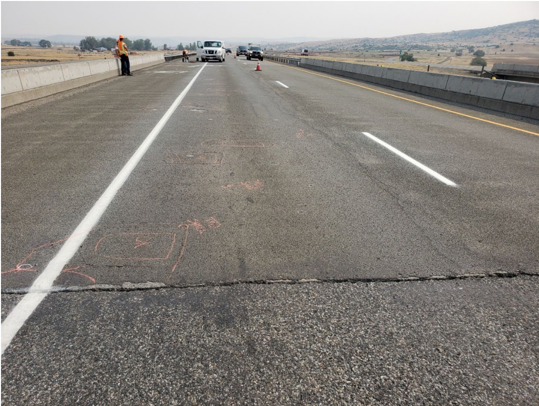
Figure 11. Overview of the driving lane and shoulder for Bridge 1670 in 2022.
