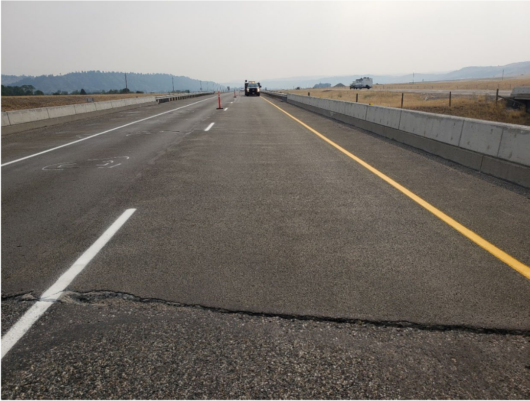
Figure 21. Overview of Bridge 1682 in 2022. Note photographer is facing into oncoming traffic.
