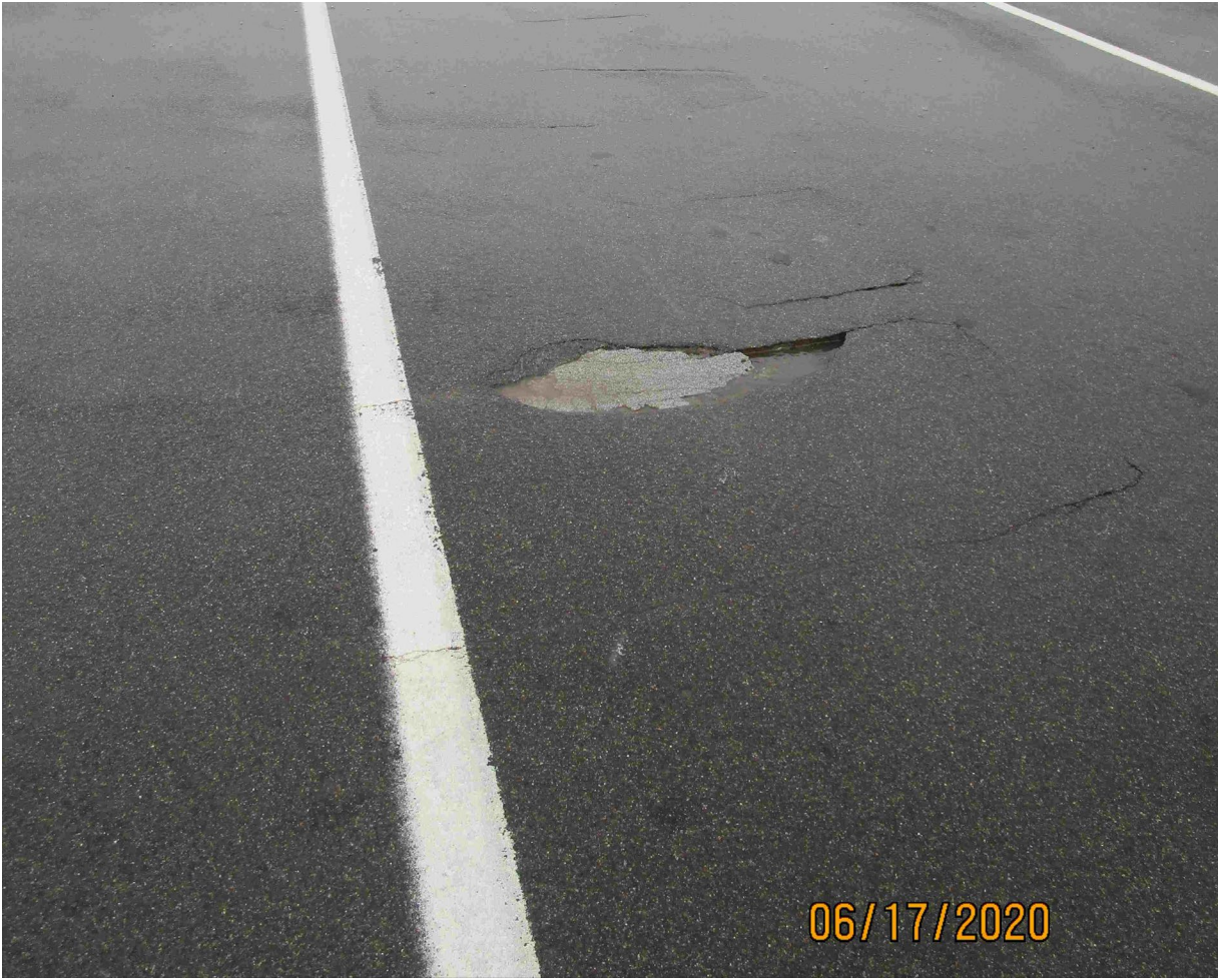
Figure 8. Reflective cracking and spalling over partial-depth repairs on Bridge 1682 in the Billings District. Image provided by MDT.
