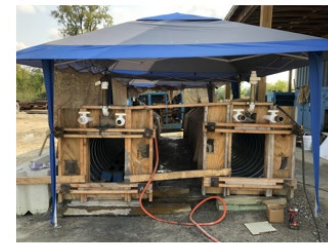
Grout Inlet End
