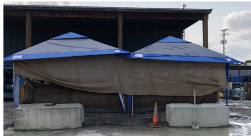
Figure 4: Culvert Grouting Test Setup.
