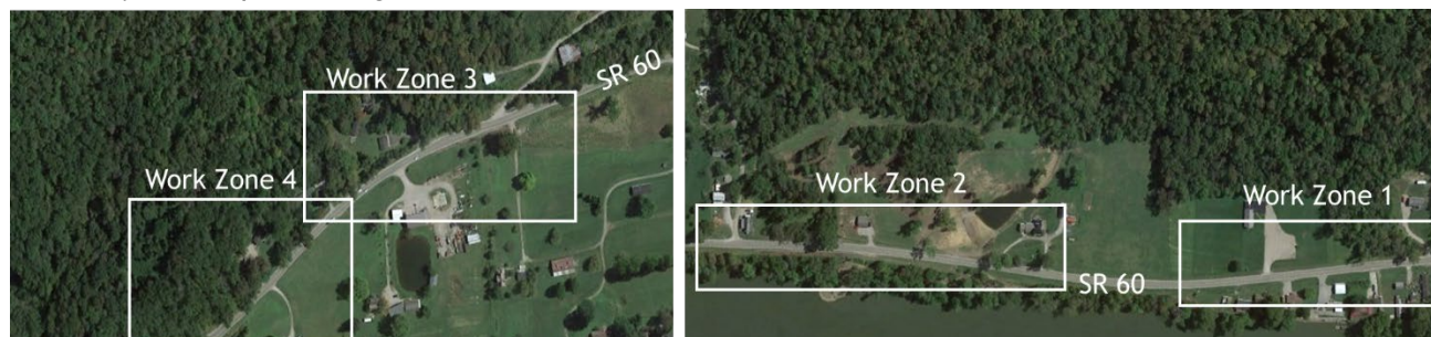
Figure 1. State Route 60 Project Area
