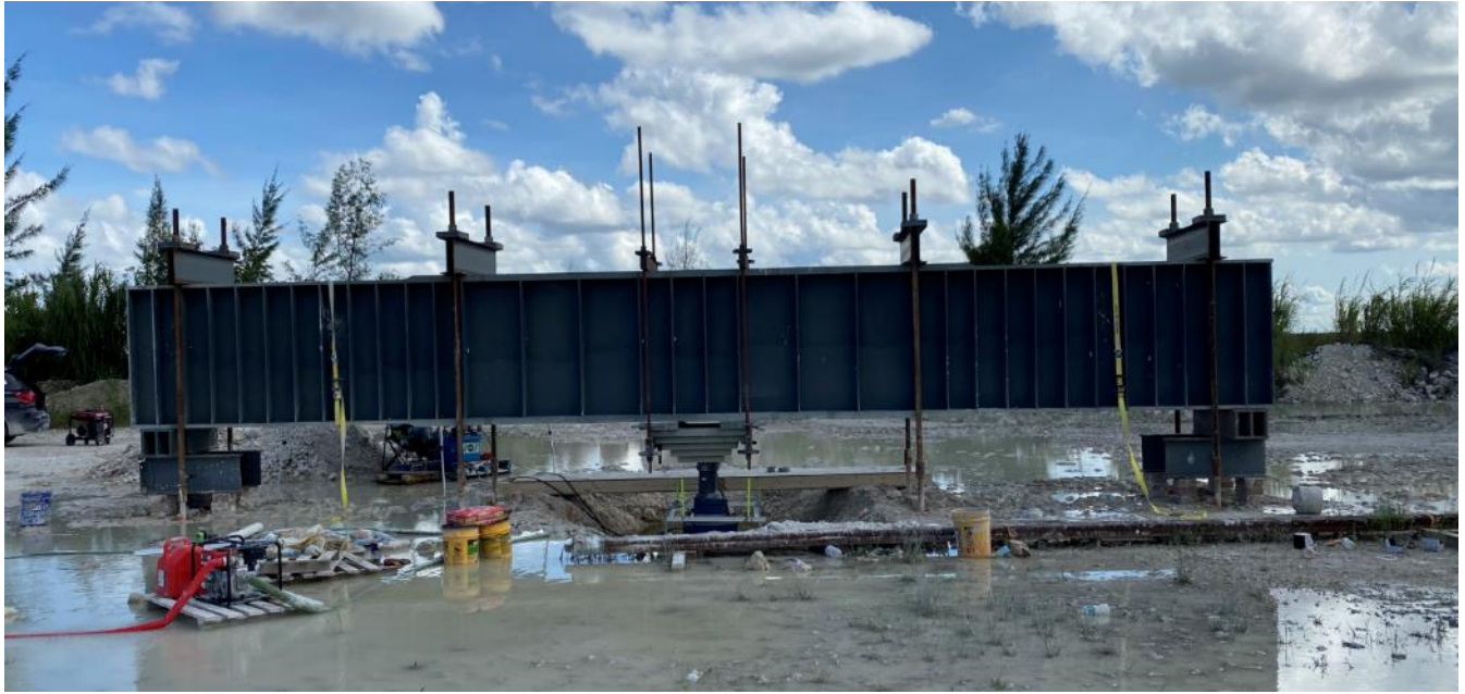
Figure 5-27 Completed construction of load test at Cemex site
