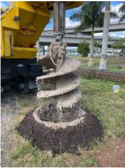
Figure 6-15 Drilling for the East shaft: (a), (b), and (c): 42-in rock auger bit; (d): 42-in temporary casing
