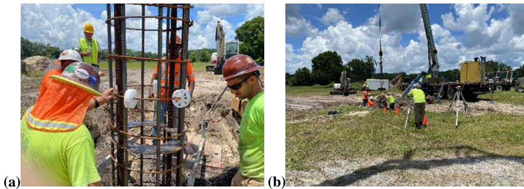
Figure 7-12. Completed construction of the East shaft: (a) cage spacer installations and (b) leveling both shafts
