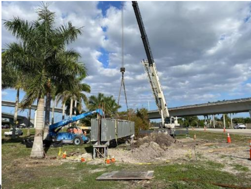
Figure 6-29 Placement of girders: (a-b) girders lifted by the crane; (c) using forks to against the girders; (d) ratchet straps around the girders
