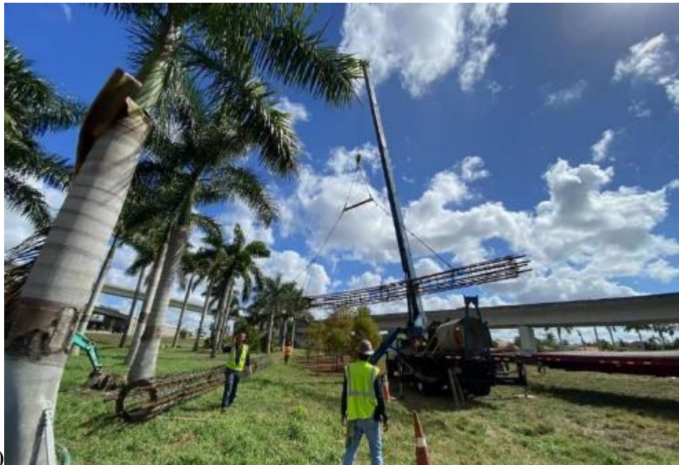
Figure 6-12 Picture of steel rebar cages: (a) templates position: top, middle, bottom; (b) William threaded rods with templates secured by the nuts; (c) 8 of No. 10 rebars; (d) rebar cages at the site; (e) unloading the rebar cages at the site
