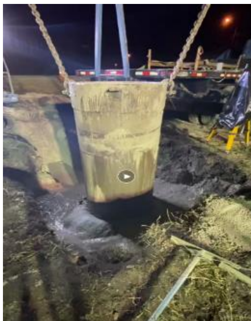
Figure 6-21 Temporary casing pull out and concrete overflow
