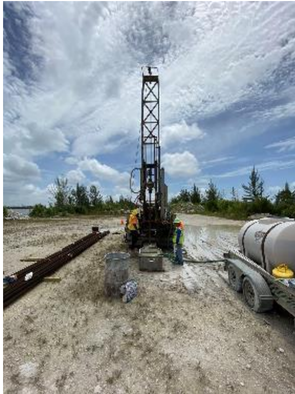
Figure 5-13 Drilling process with threaded rods nearby
