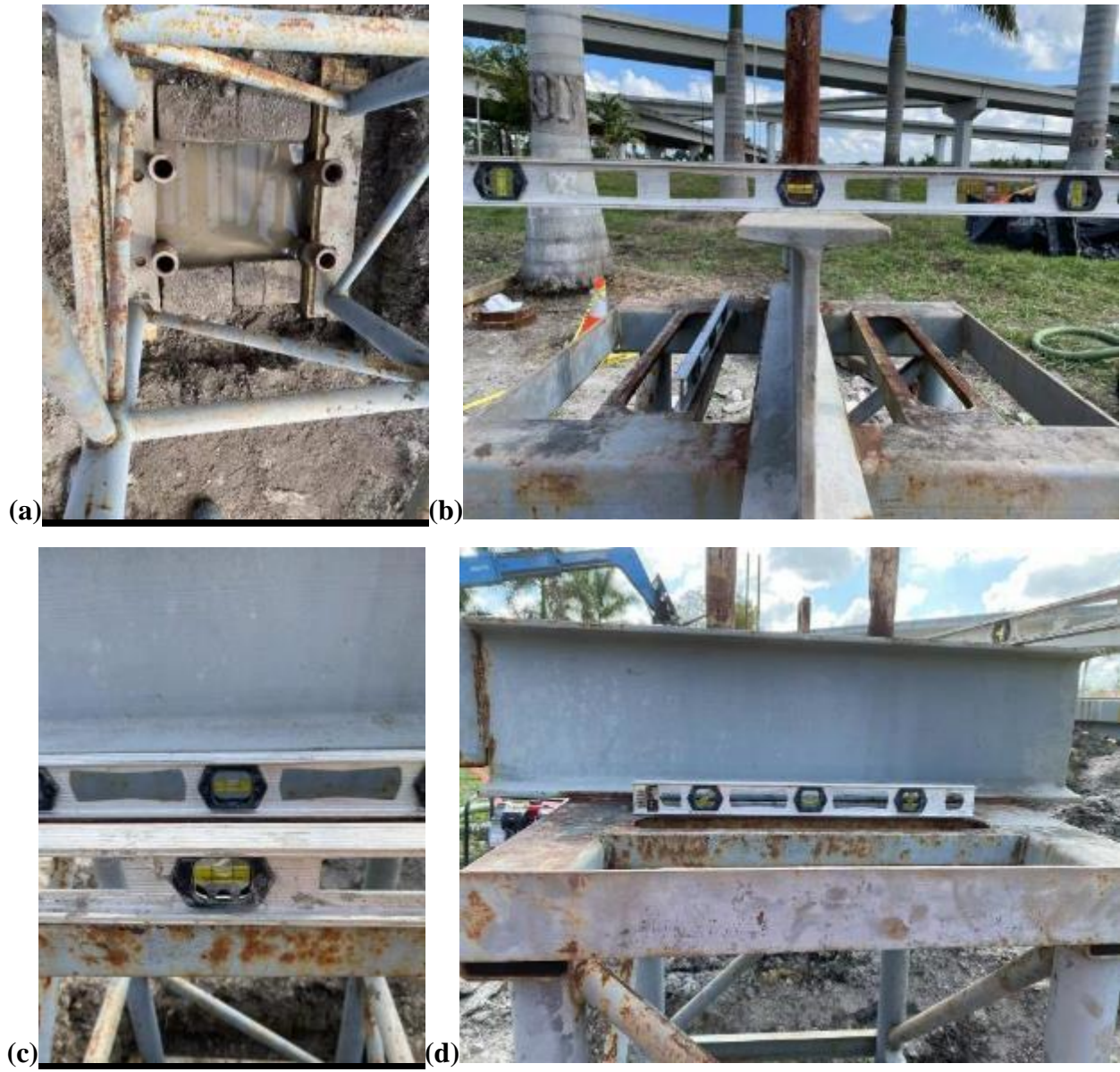
Figure 6-28 (a) stands on the top of bricks; (b-d) stands are leveled in both directions
