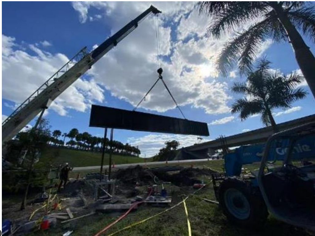
Figure 6-29 Placement of girders: (a-b) girders lifted by the crane
