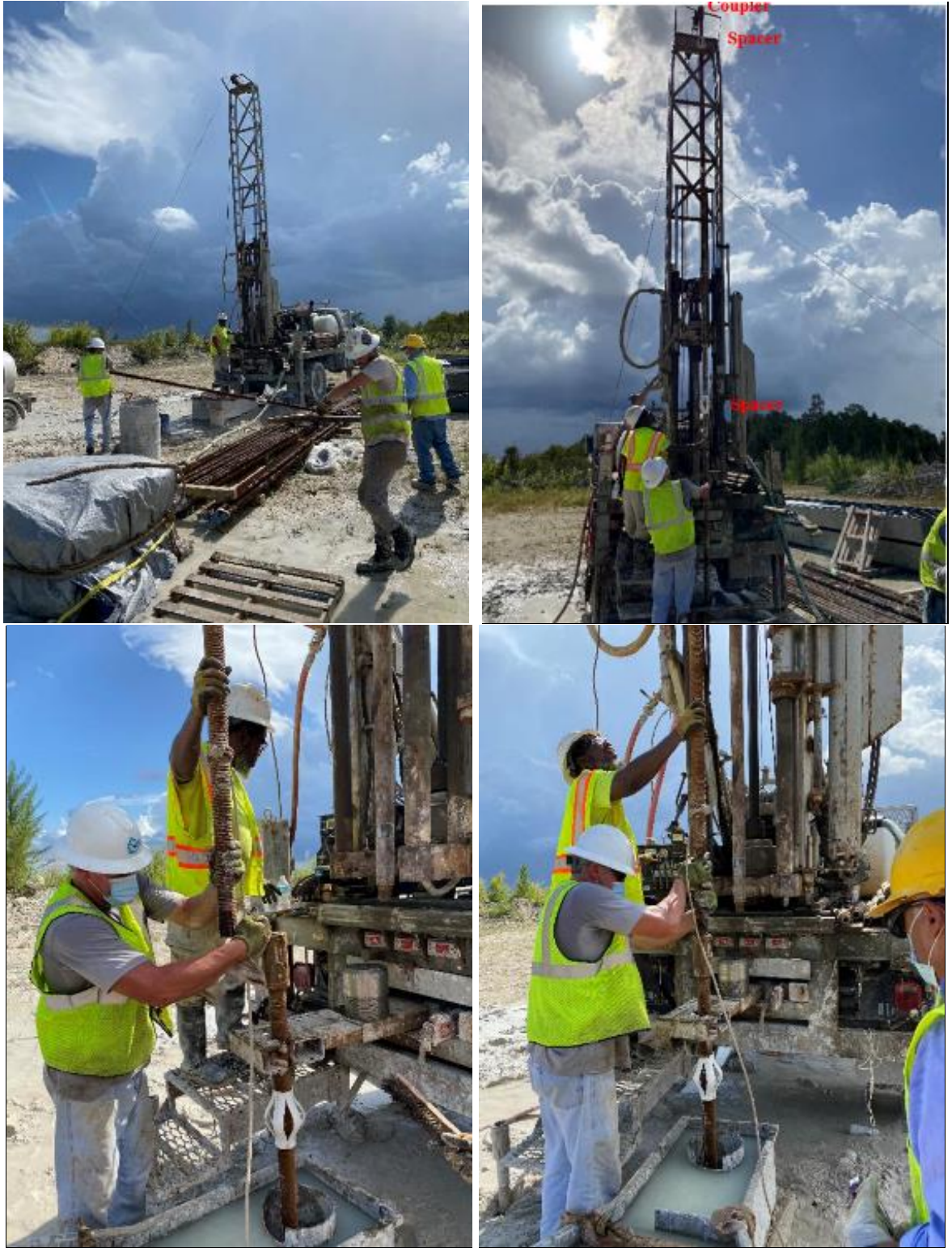
Figure 5-14 Placement of 36-ft- and 20-ft-long threaded rods with centralizers
