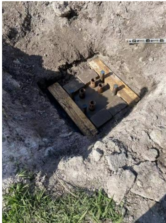
Figure 6-27 Bricks and wood spacers on top of shafts beneath test stands
