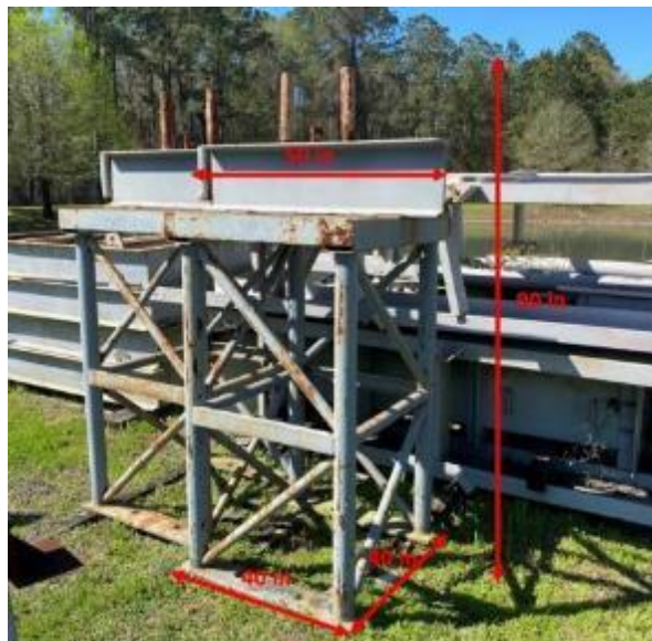
Figure 6-25 Stands to support the girders
