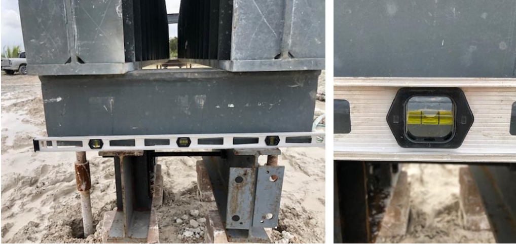
Figure 5-23 Bubble level on the two wide flange beams
