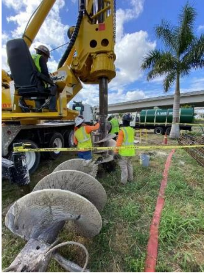
Figure 6-16 Change to the 36-in rock auger bit
