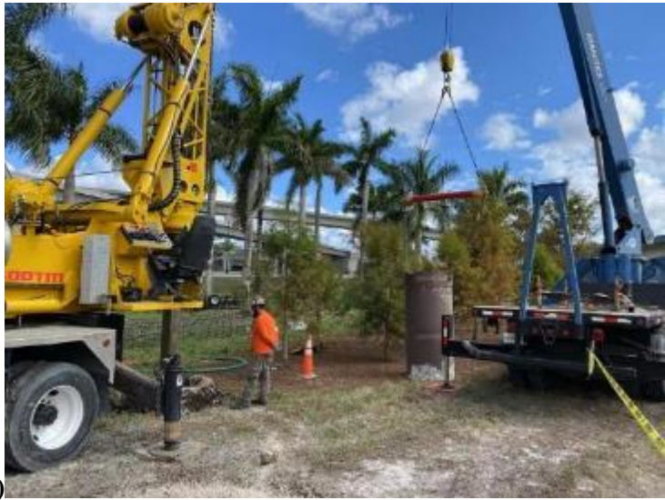
Figure 6-15 Drilling for the East shaft: (a), (b), and (c): 42-in rock auger bit; (d): 42-in temporary casing
