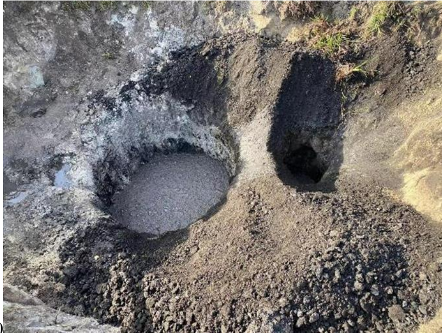
Figure 7-11. Sinkholes that opened during the East shaft construction: (a) 12 in chimney sinkhole opened at 45ft depth near the East shaft; (b) filling the East shaft with asphalt waste (rap) to plug the chimney sinkhole alongside the shaft and (c) another sinkhole at 15' depth in wall of the East shaft
