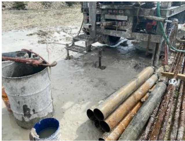
Figure 5-9 6 in casing used for drilling
