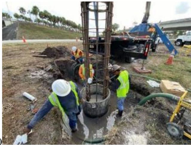
Figure 6-18 (a) Placement of the rebar cage (b) spacer installation
