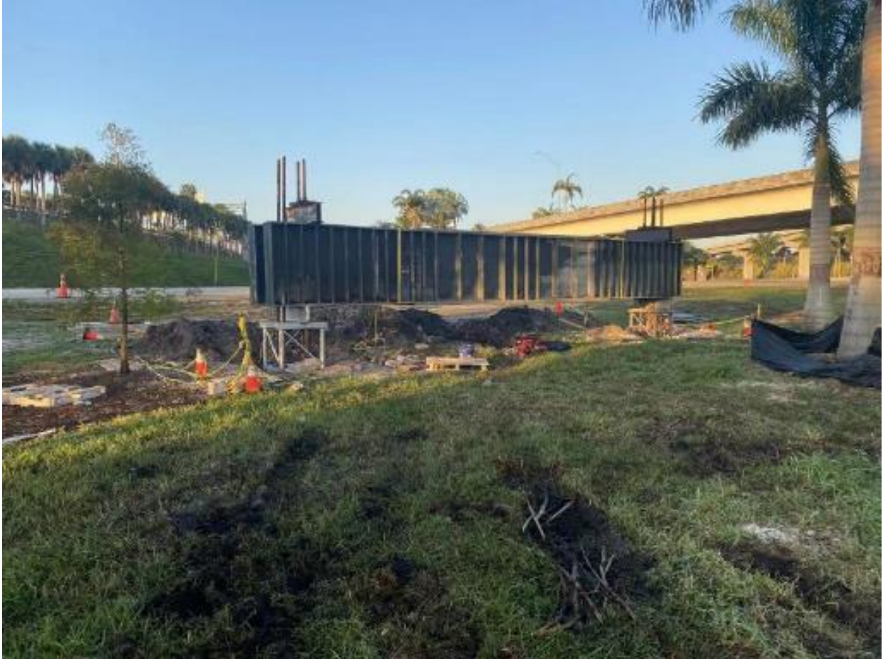
Figure 6-30 Installation of two sets of C channels and plates
