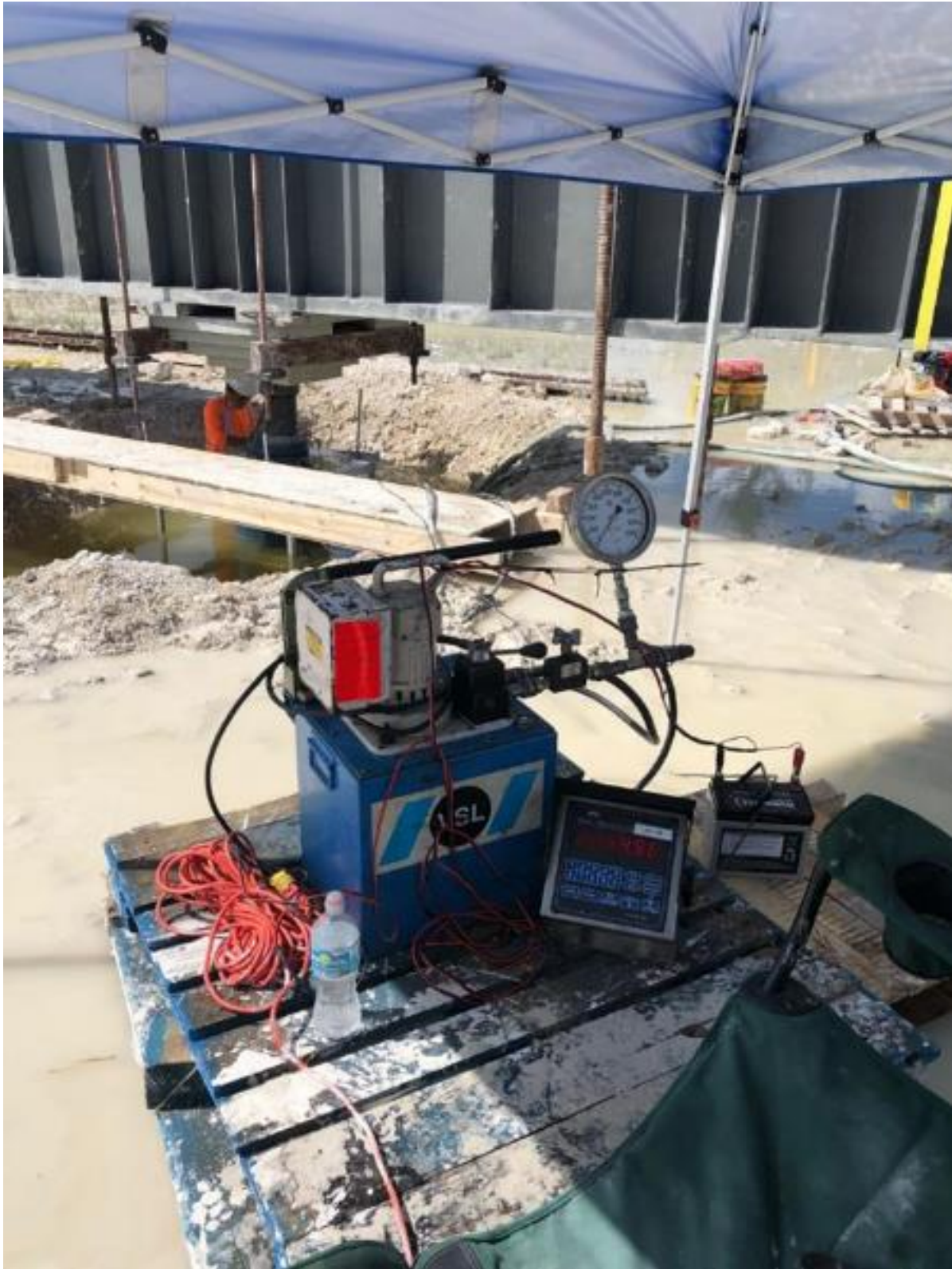
Figure 5-25 Hydraulic jack and load cell setup
