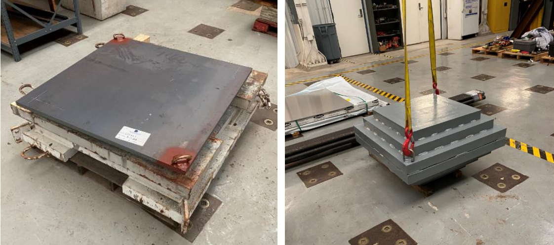
Figure 5-21 D-rings welded on the plates and the new load spreader
