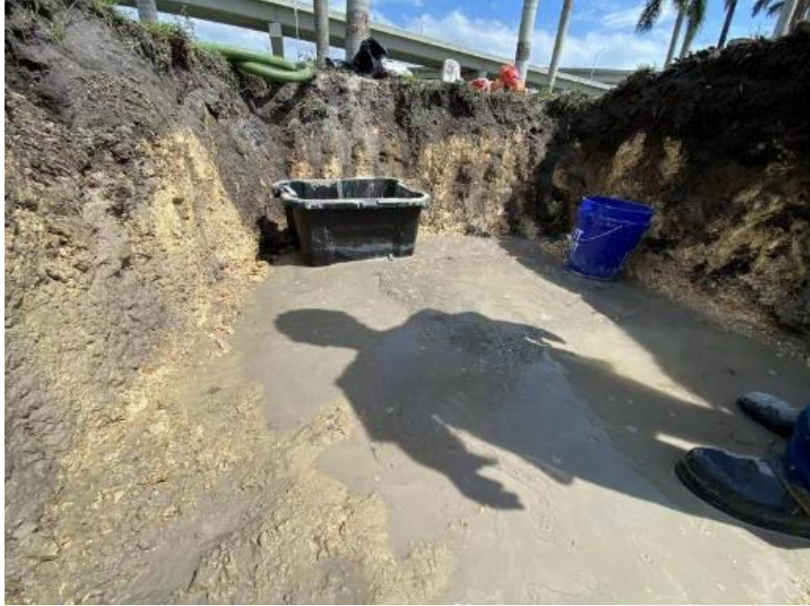
Figure 6-26 Fast setting concrete placement
