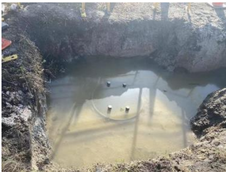
Figure 6-22 Picture of the east drilled shaft after two days of installation
