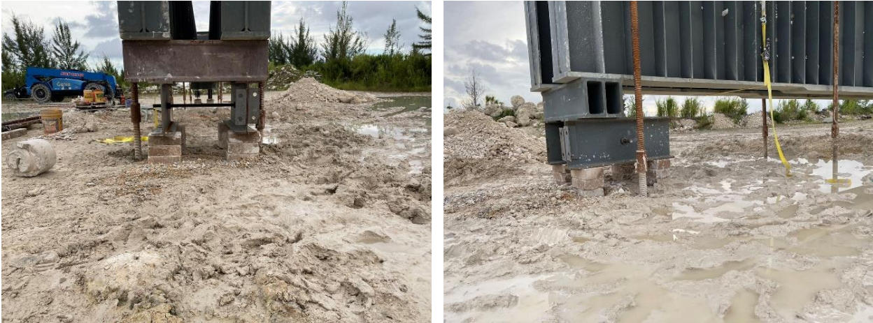
Figure 5-22 Twelve bricks under support systems at each end of girders
