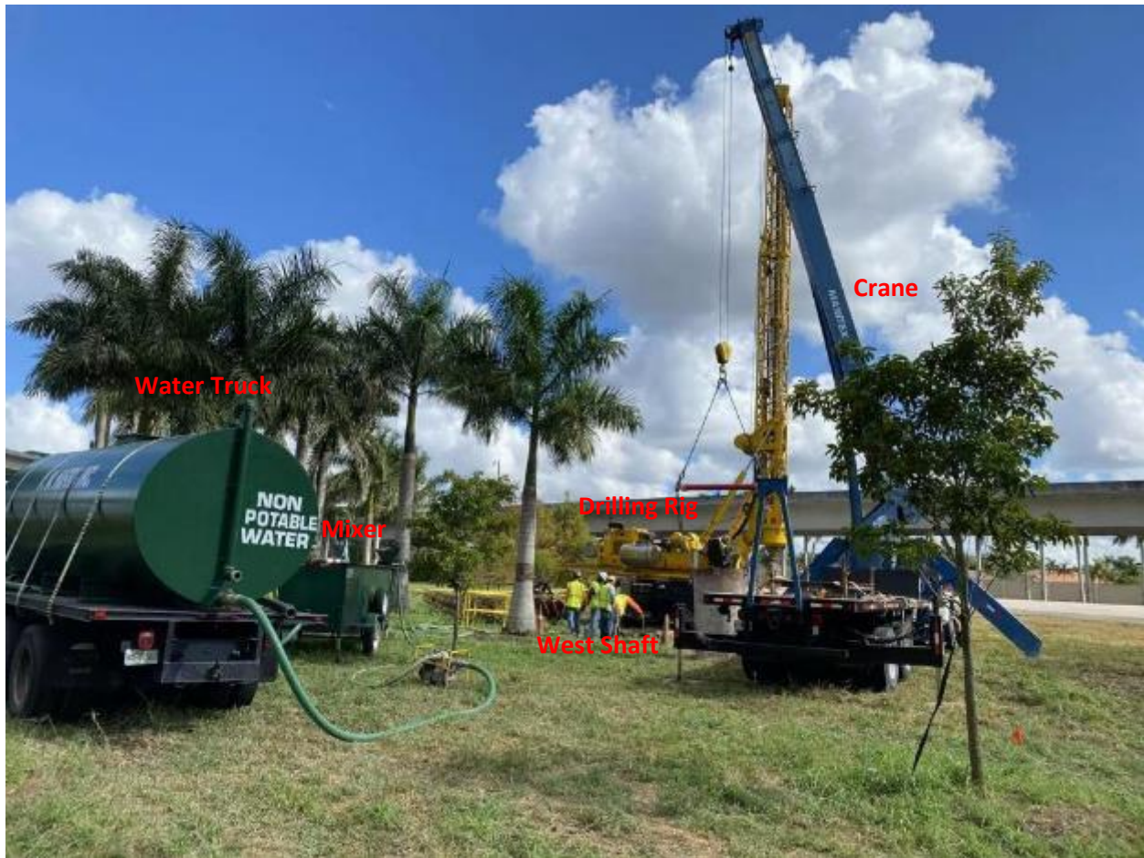
Figure 6-14 First attempt to install the west shaft
