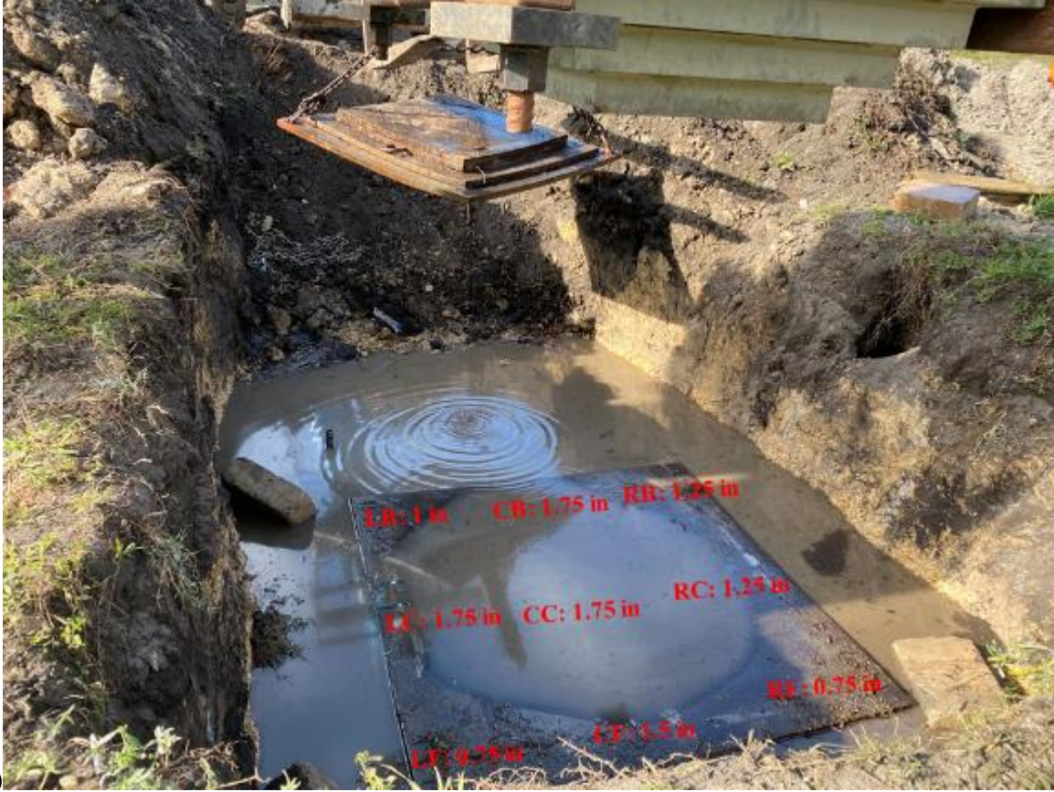
Figure 6-36 (a) picture of 28 in by 28 in steel plate before test; (b) picture of 28 in by 28 in steel plate after test; (c) picture of 48 in by 48 in steel plate after test with settlements at each location
