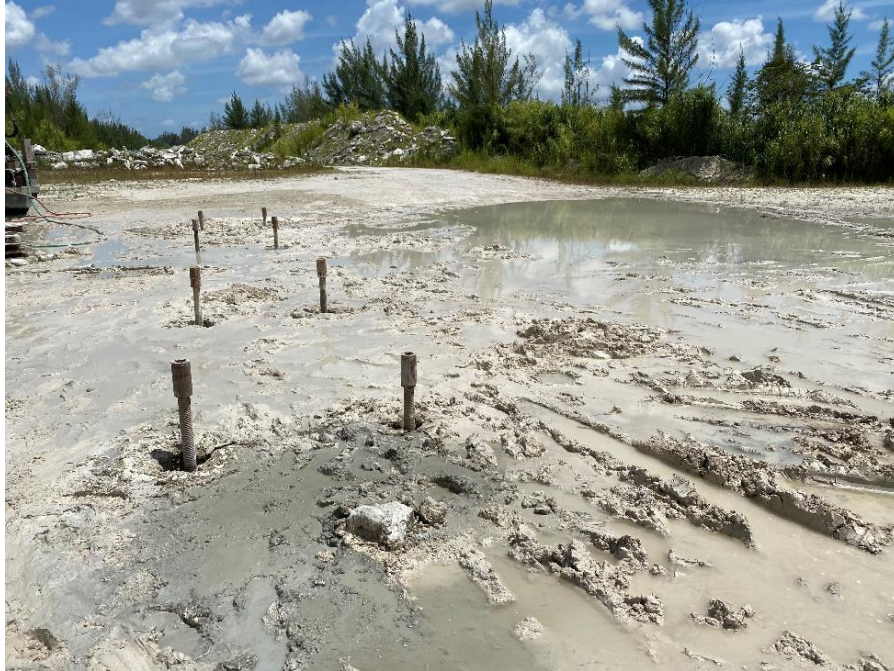
Figure 5-17 Eight micropiles after installation
