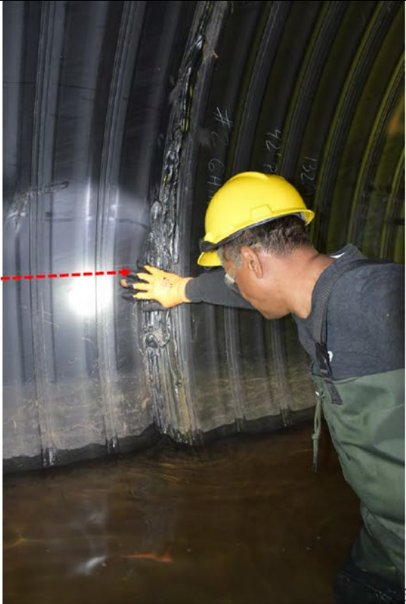
Several Cracks at the Bulkhead and Shape Distortion
