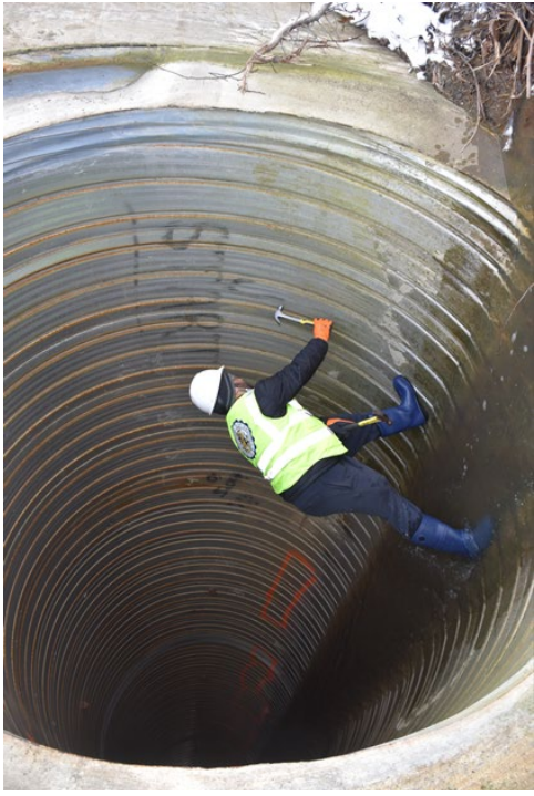
(a) Tapping the Liner Pipe with a Hammer
