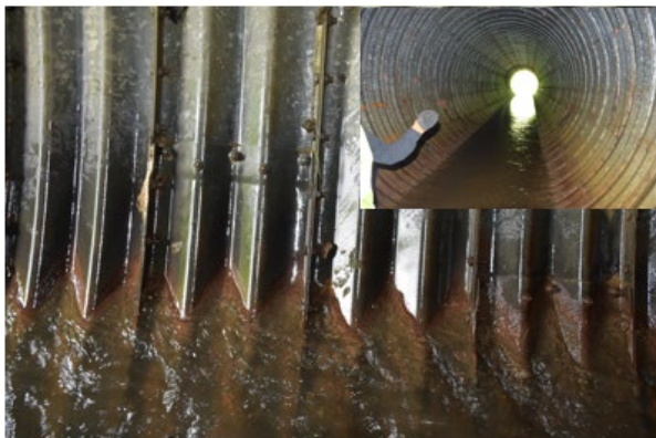
(c) Sectional Corrugated Metal Pipe
