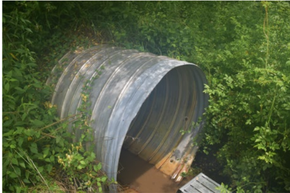
(a) Corrugated Steel Spiral Rib Pipe
