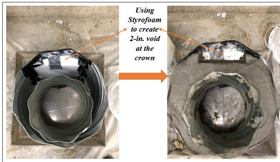
Figure F.22: Creating a Crown Void in the Sliplined Culvert.
