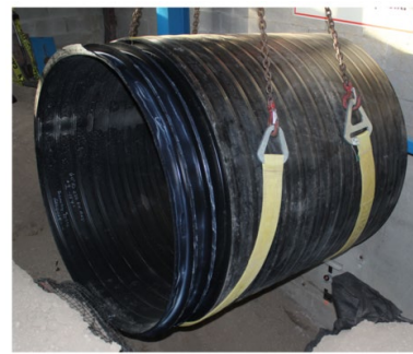
(b) HDPE liner pipe
