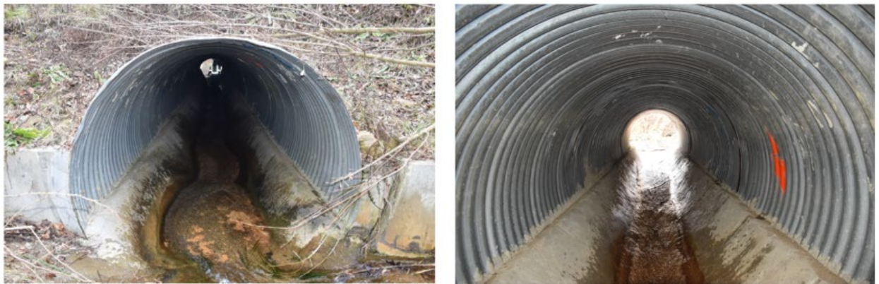
Culvert Access: This culvert was not a sliplined culvert.
