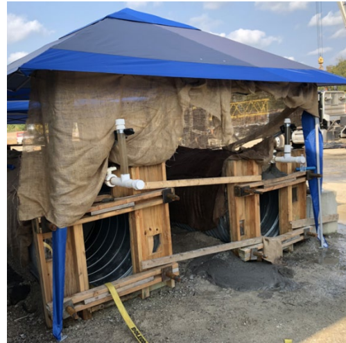
(c) Outlet side of culvert
