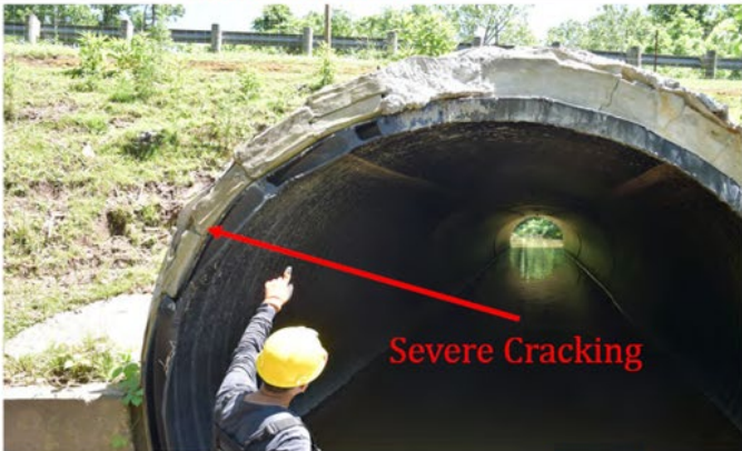
Several Cracks at the Bulkhead and Shape Distortion
