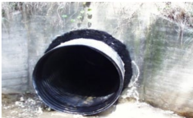
Figure A.13: After grouting, the pipes are sealed tightly together (Armstead 2015).
