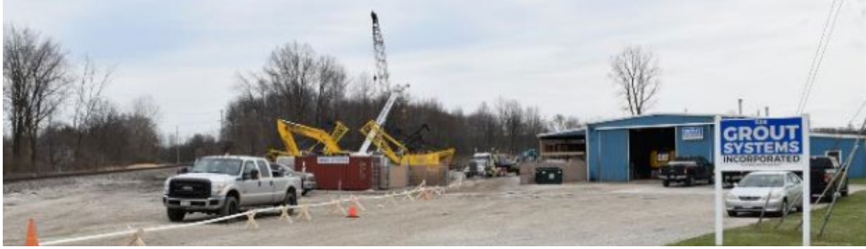
Figure 10: Field Pumping Tests of the Proposed CLSM or Cellular Grout C40.
