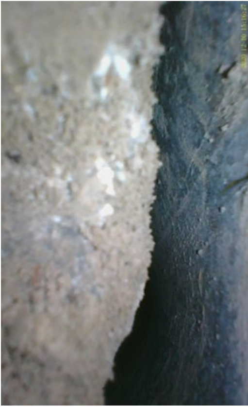
(c) Delamination (left: at the liner pipe; right: at the host pipe)
