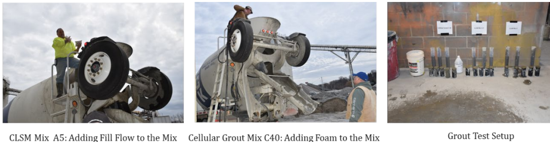
Figure 9: Commercial Scale Mixing of the Proposed CLSM or Cellular Grout C40.
