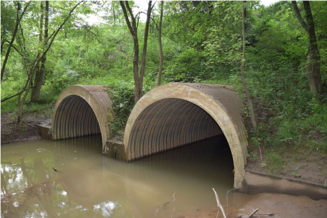
Culvert Access: High Water Level
