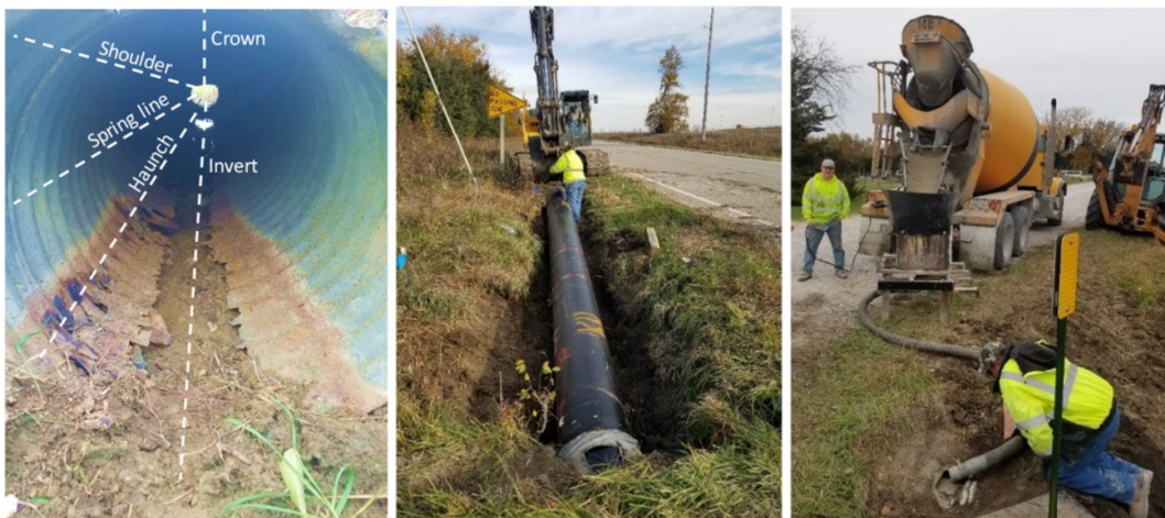
(a) Corroded corrugated steel pipe
