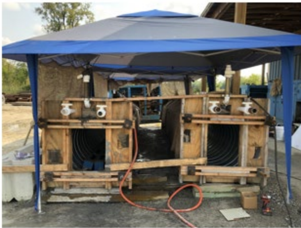
Grout Inlet End
