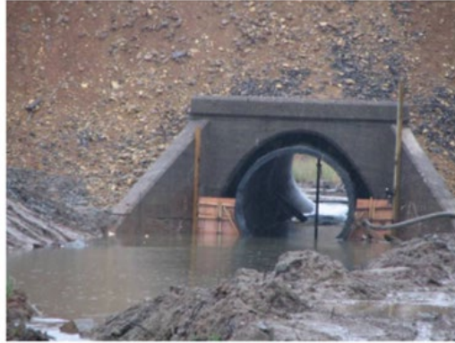
Figure A.5: A culvert renewed by sliplining (Source: Terrafix Geosynthetics Inc., Salem et al. 2010).
