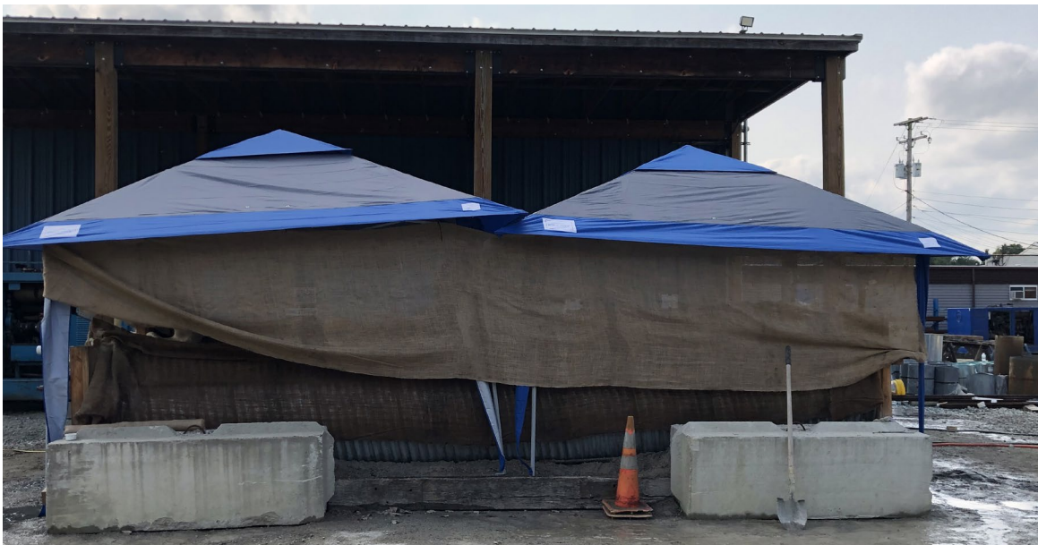
Figure 11: Culvert Grouting Tests: Setup of Two 20-ft.-Long Test Specimens.
