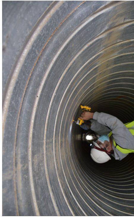
(c) Drilling a Hole in the Liner Pipe.
