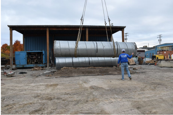
(a) Lifting of culvert specimens
