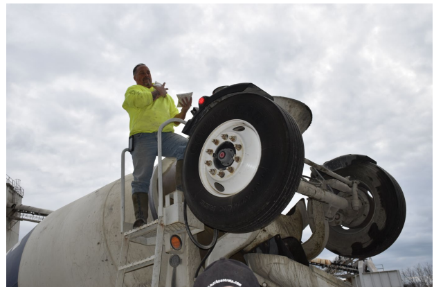
(b) Adding Fill Flow to CLSM Mix A5
