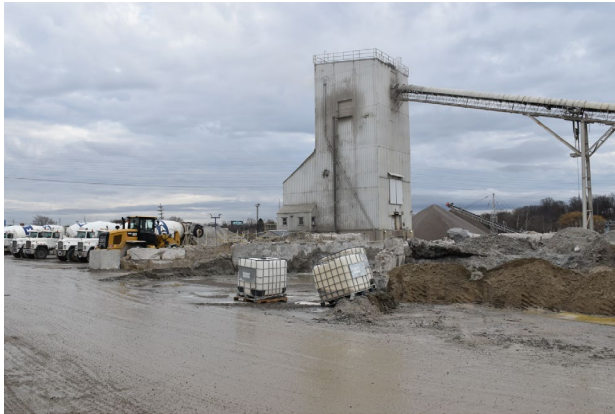
(a) Mack Ready Mix Concrete Facility
