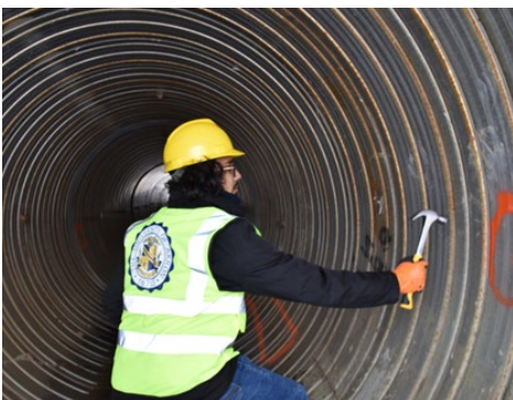
Figure 2: Sounding Method for Culvert Inspection ( Left ); Endoscope Camera for the Inspection of Voids ( Right ).
