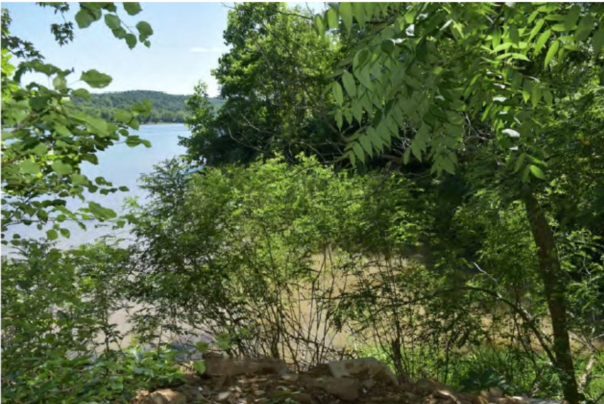
Culvert Access: Inspection was aborted due to high water level and unsafe access.
