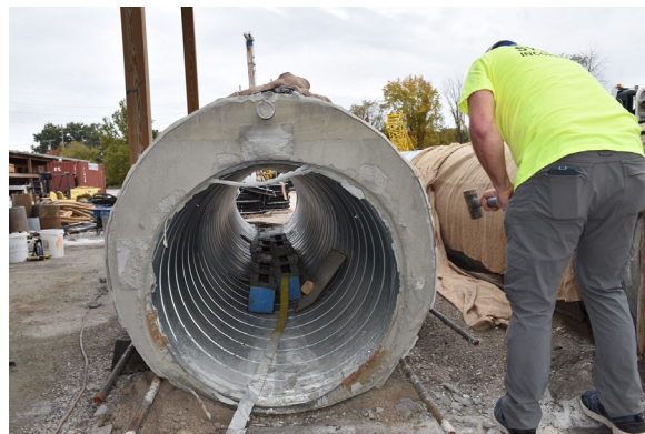
(b) Cellular Grout C40 at outlet
