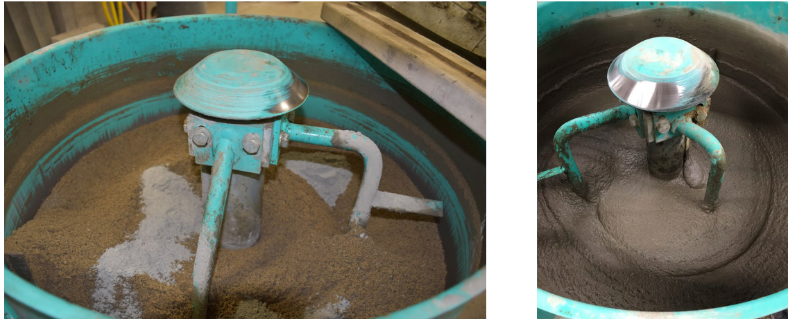
Figure F.6: Mixing CLSM Grout using a Mortar Mixer: Mixing Dry Components ( left ), CLSM Mix after Addition of Water ( right ).
