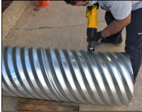
(a) Cutting the host pipe.
