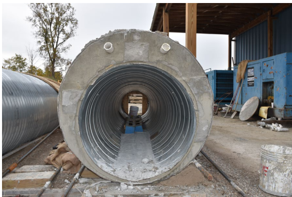
(a) Cellular Grout C40 at inlet
