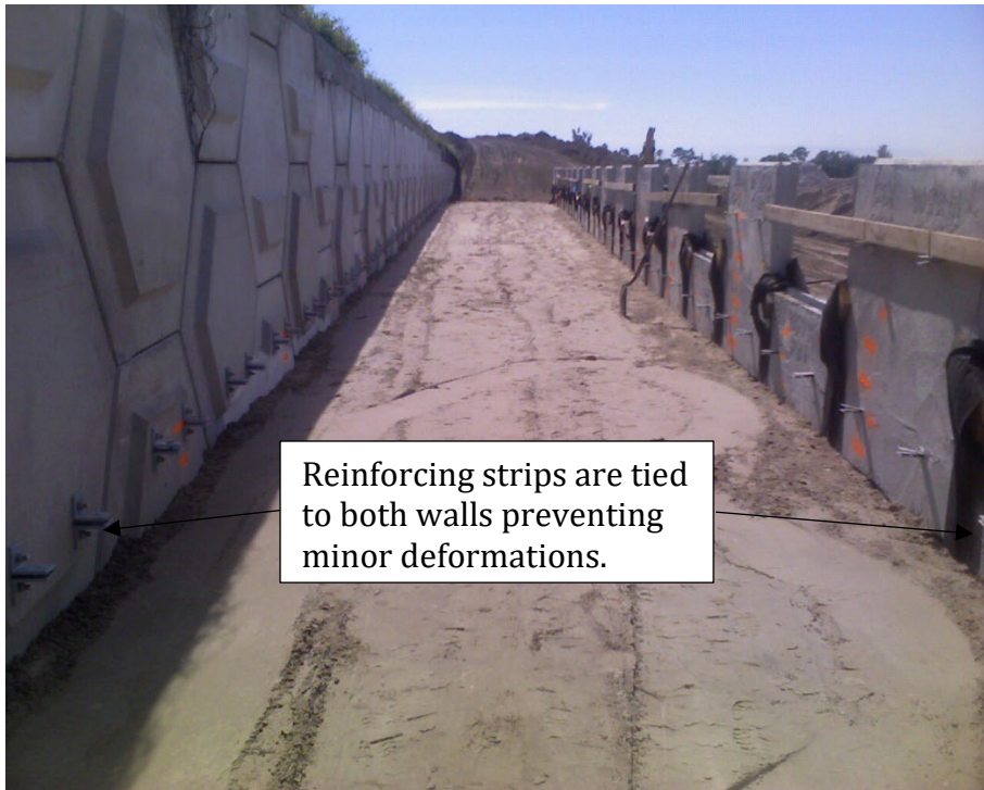
Figure 1-2. MSE wall embankment widening scenario.
