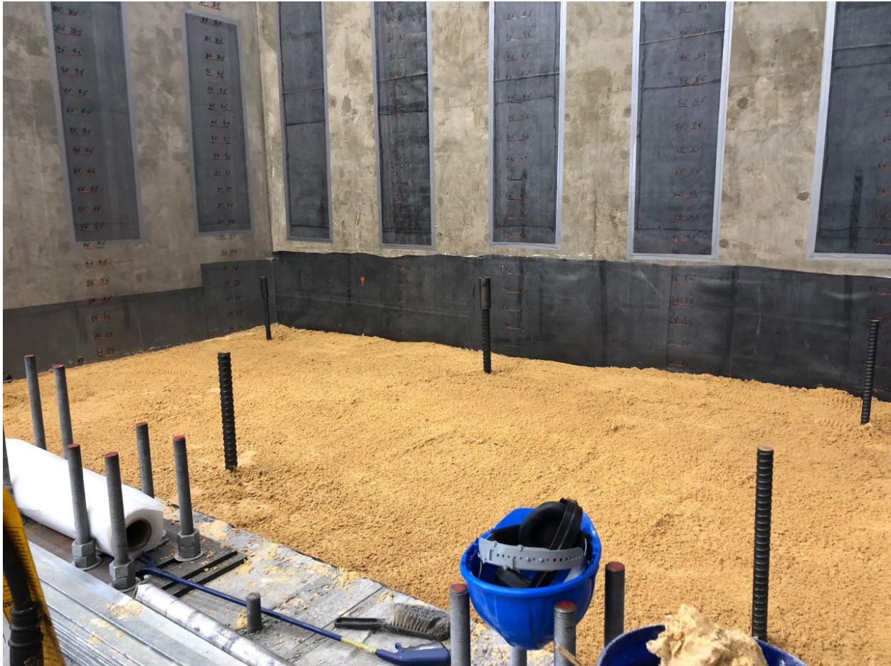
Figure 4-6. Base layer soil placement.
