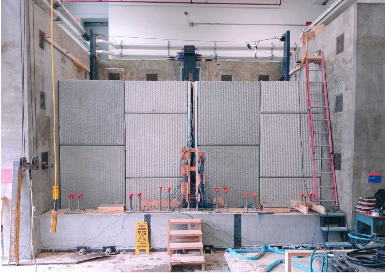
Figure 4-32. Temporary wall bracing removed after completing wall construction.
