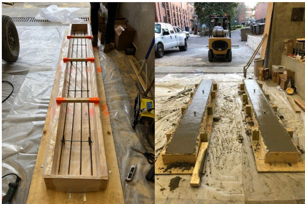
Figure 4-9. Building steel reinforced leveling pad forms and casting concrete.
