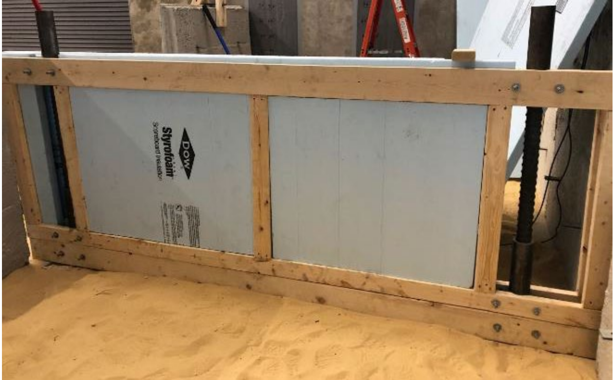
Figure 4-17. Constructing the frame for the compaction effort divider.
