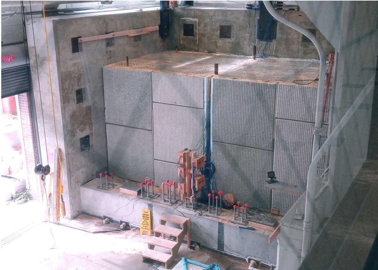
Figure 4-33. Overview of MSE wall area.
