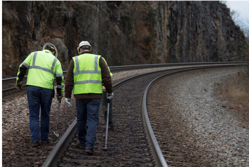
Figure 22. Walking inspection for broken spikes near Shawsville, VA
