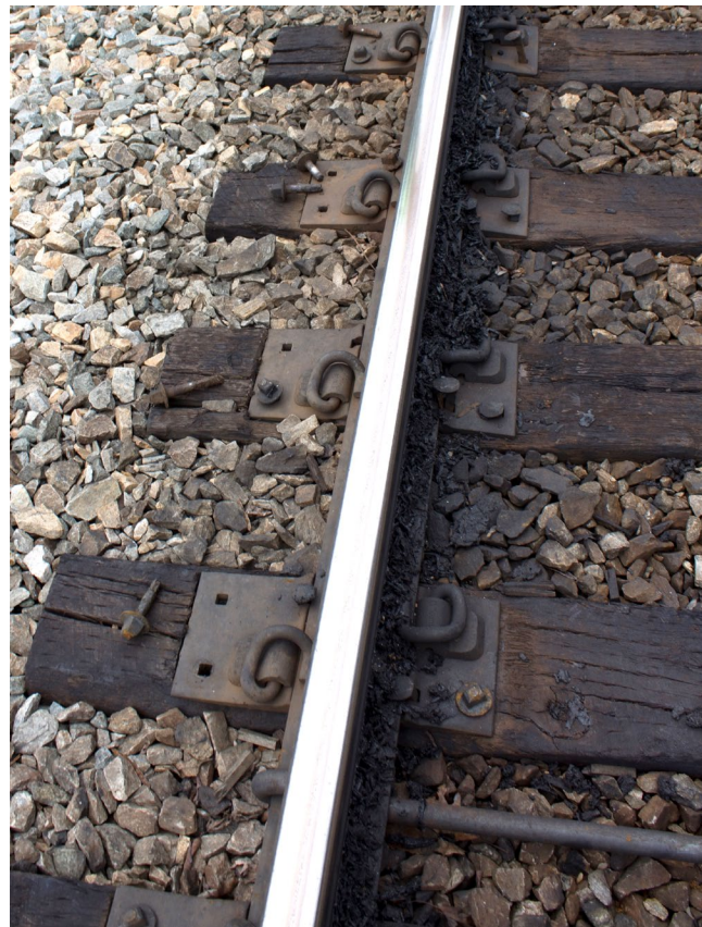
Figure 27. Location with cluster of broken spikes; note gage rod
