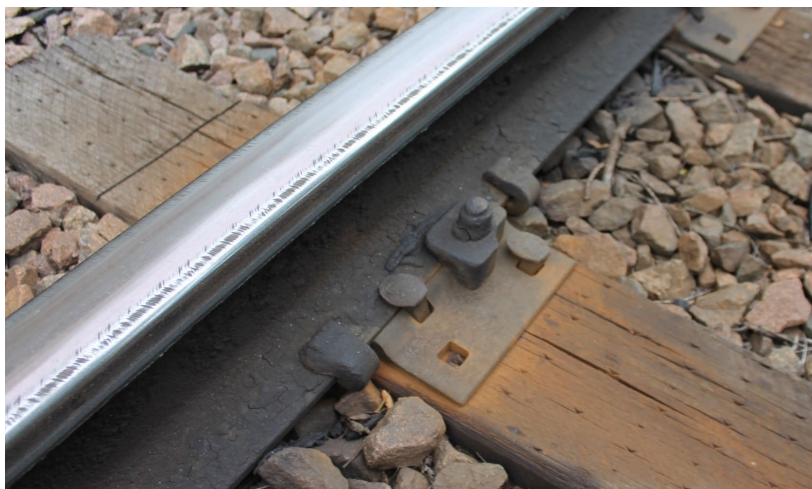
Figure 2. Traditional fastening system with curve blocks installed
