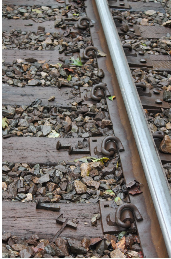
Figure 47. Cluster location with multiple plates in a row with broken spikes
