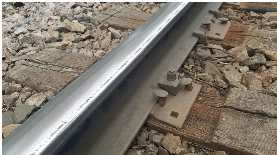
Figure 32. Example of a traditional tie plate with a curve block
