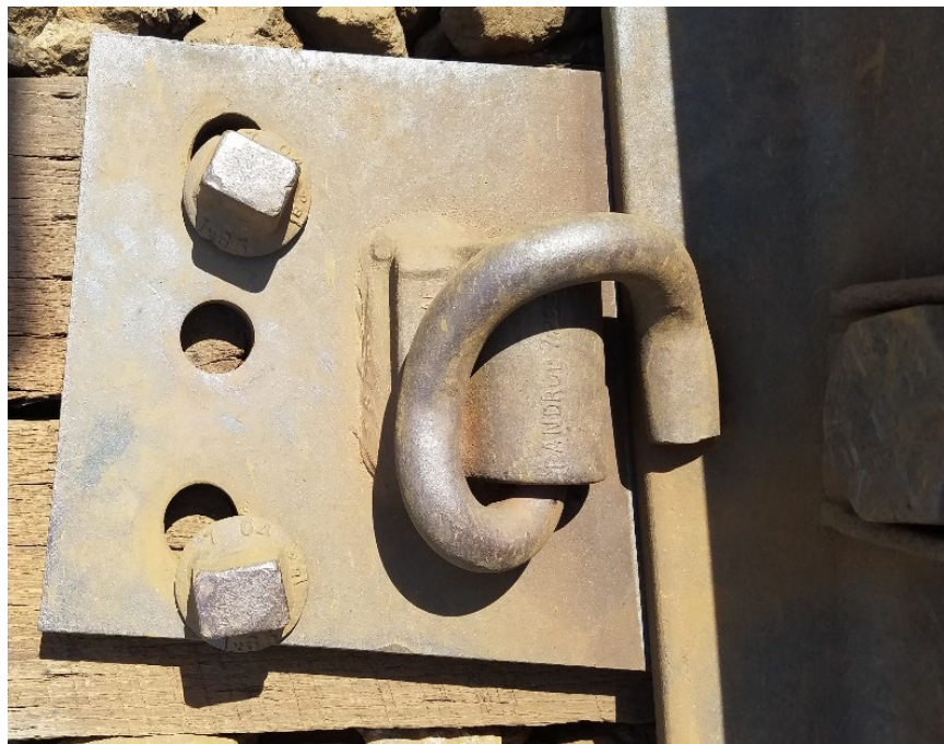
Figure 34. Longitudinal plate movement with stationary spikes
