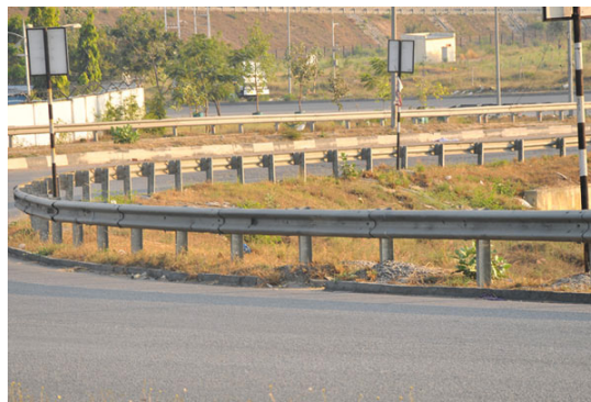
Figure 2.2: W Beam Guardrail on the outside of the lane
