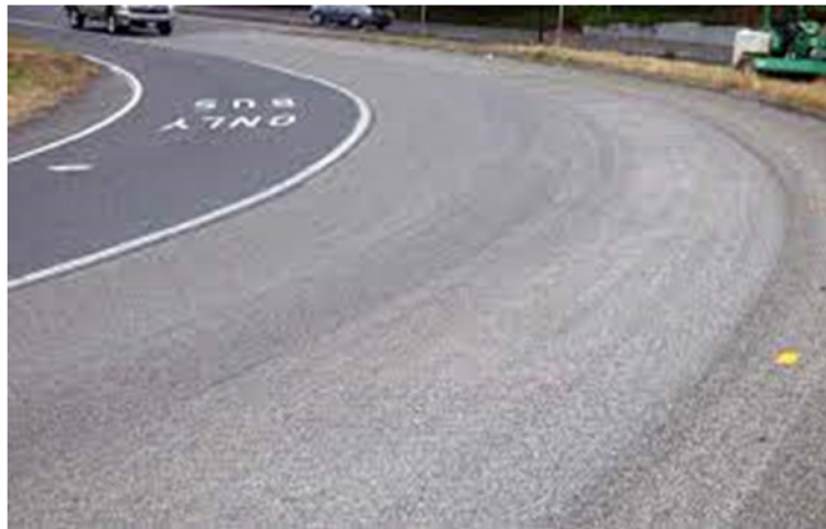
Figure 2.5 High friction road treatment (WSDOT, 2019)
