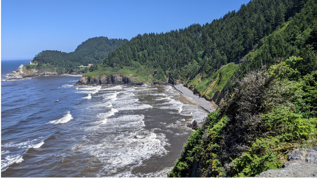
Figure 7.19: Northward view from the Sea Lion Point pullout (June 2022). The section that was recently repaired is located in the center right of the photograph.
