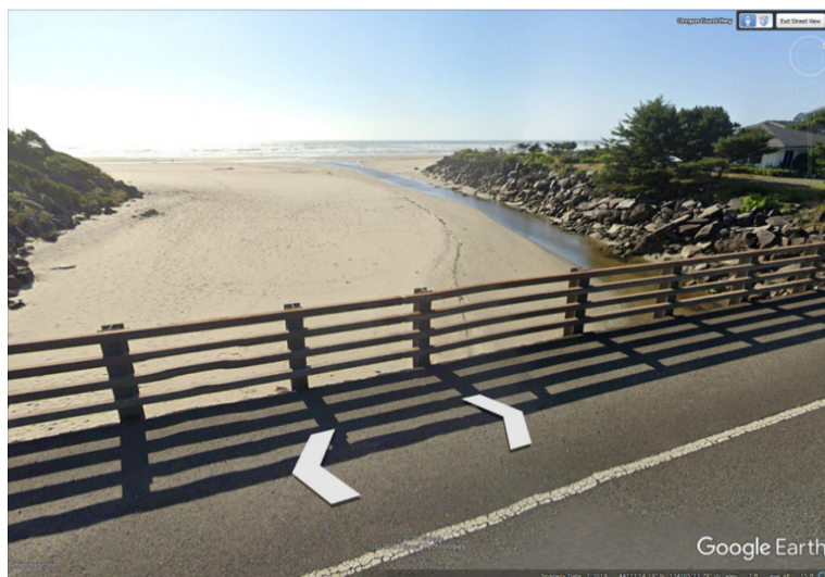
Figure 2.7: Riprap placed along the north and south stream banks and abutments at the bridge over Big Creek, MP: 160.15.
