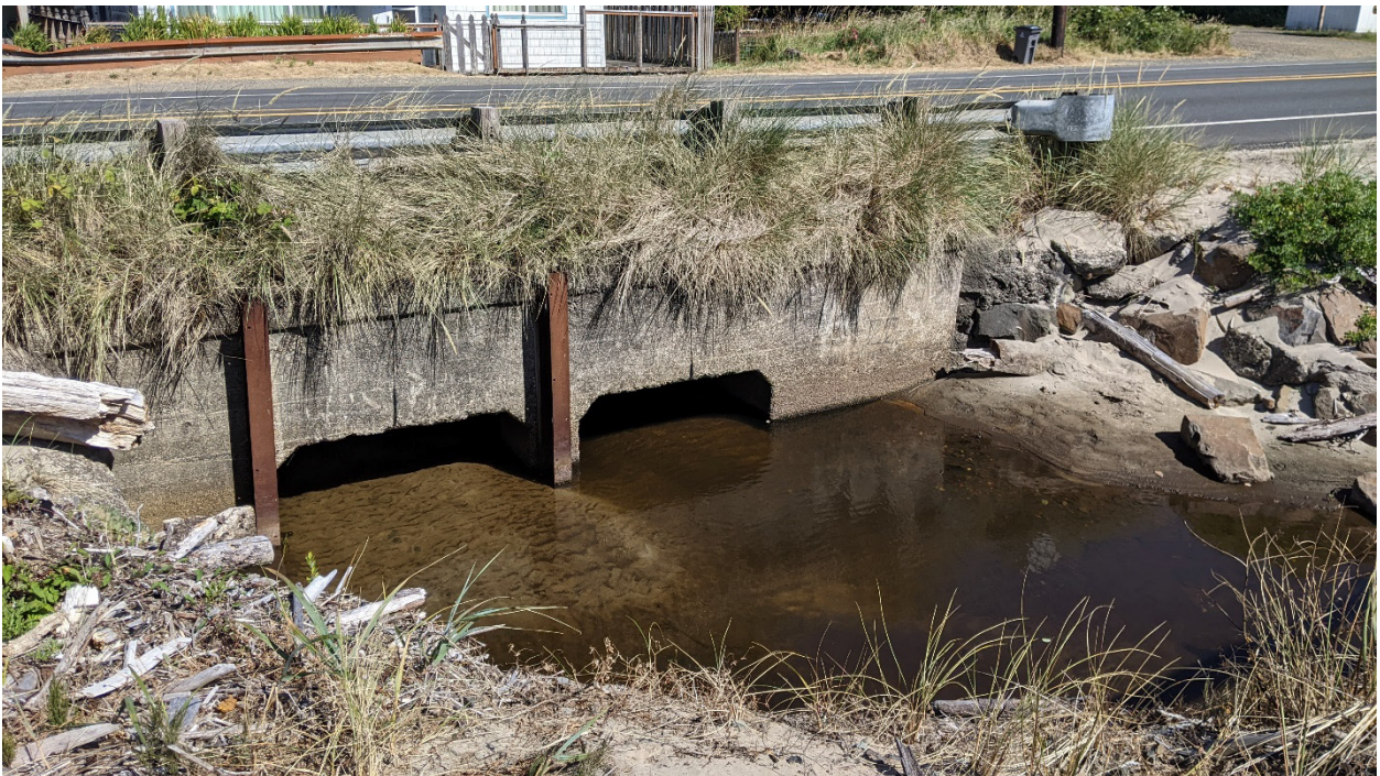
Figure 7.9: Photograph showing the culvert under the highway (July 2022).
