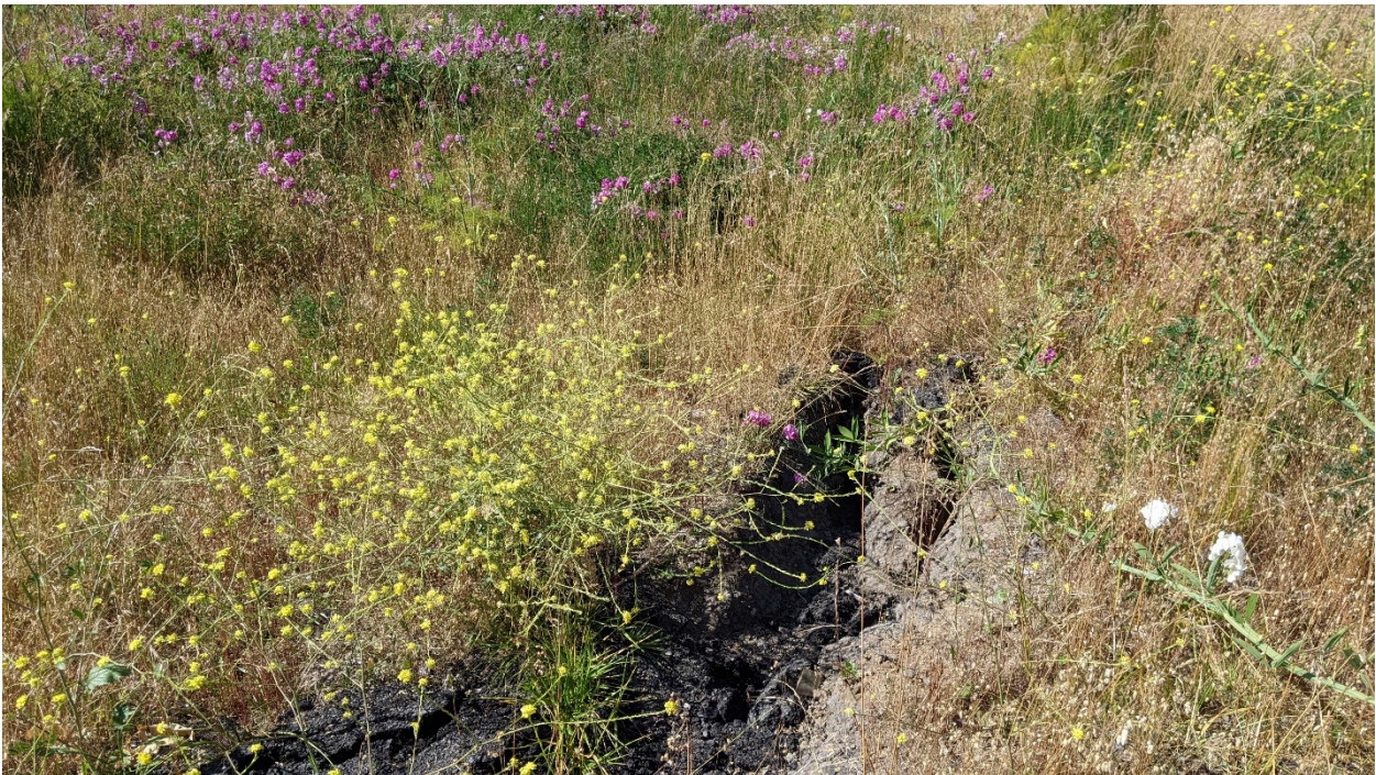
Figure 7.24: Large tension cracks present at the site (Photograph looking northwest, immediately west of the highway southbound lane & shoulder, July 2022)
