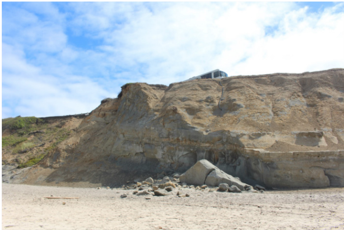
Figure 7.16: Example coastal seacliff failure at Spencer Creek (facing east, near MP 134, August 2016).
