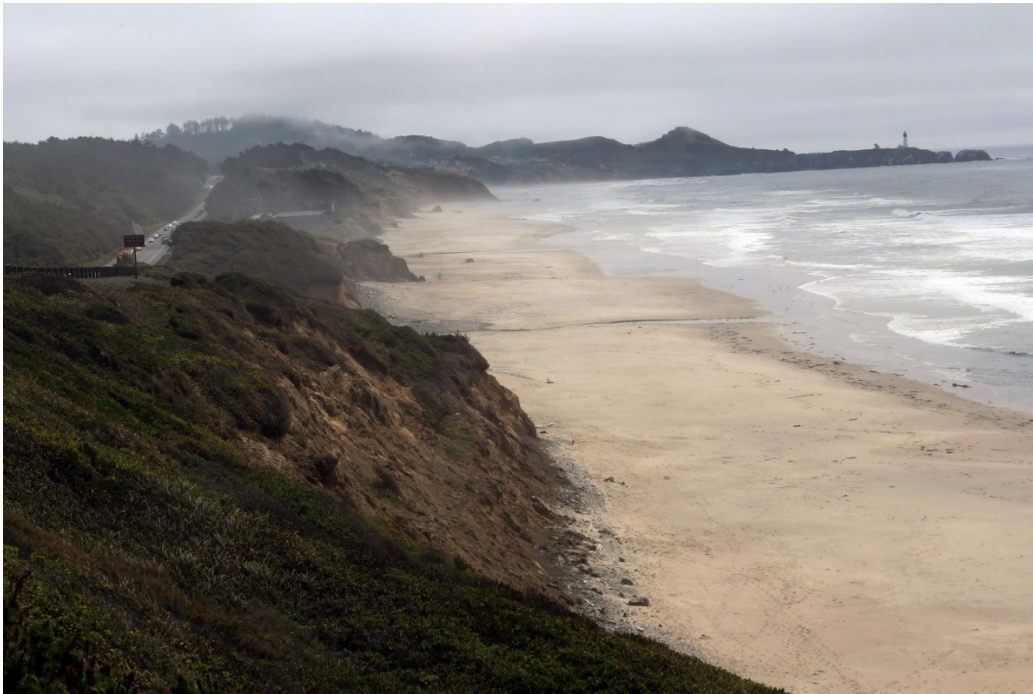
Figure 1.1: View of the Beverly Beach State Park highlighting the proximity of Highway 101 to the rapidly eroding seacliffs.
