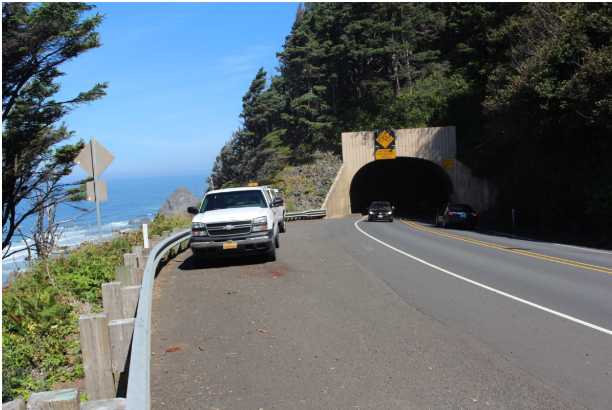
Figure 7.2: US Highway 101 facing north just before the Arch Cape tunnel (near MP36, August 2016).
