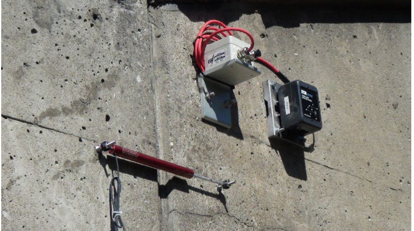
Figure 12. I-44 and Macklind Avenue – Tiltmeter and Crack meter Installation
