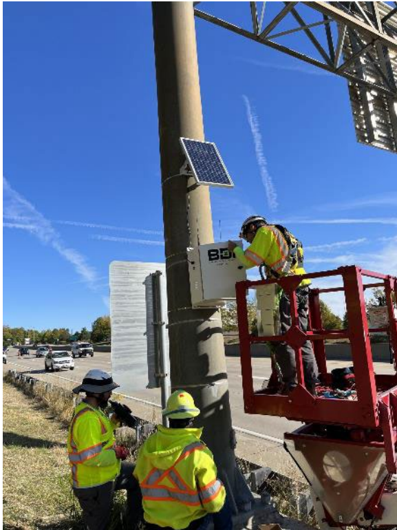
Figure 18. SB 141 at MO 100 – Gateway Installation
