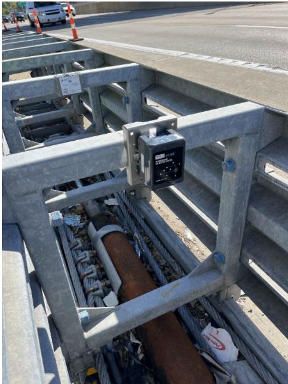
Figure 23. I-64 EB Exit Gore to Big Bend Boulevard – Accelerometer Installation
