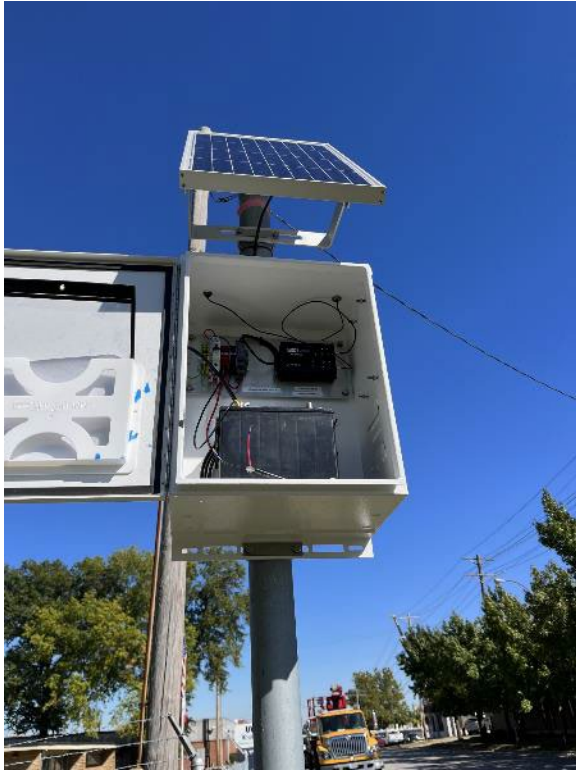
Figure 11. I-44 and Macklind Avenue – Gateway Installation
