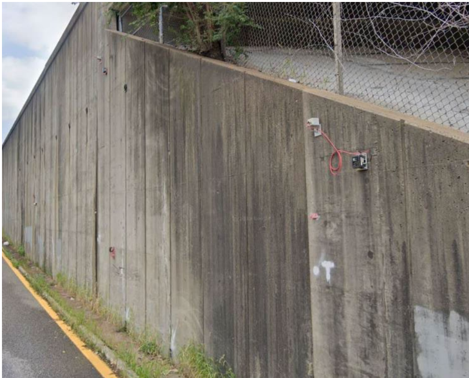
Figure 17. I-44 WB to Berry Road – Sensors Installed on Retaining Wall
