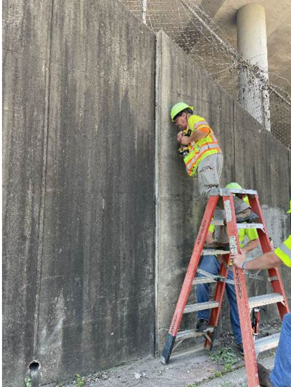
Figure 16. I-44 WB to Berry Road – Tiltmeter Installation
