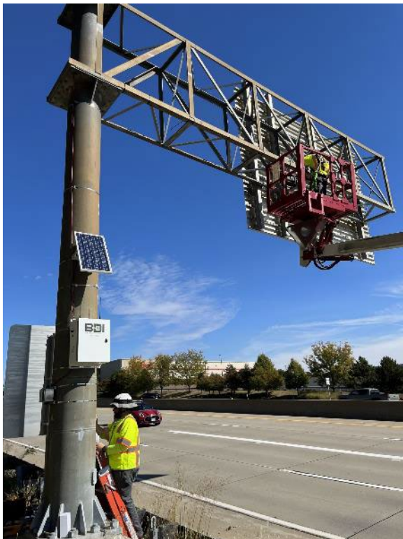
Figure 19. SB 141 at MO 100 – Accelerometer Installation on Cantilever
