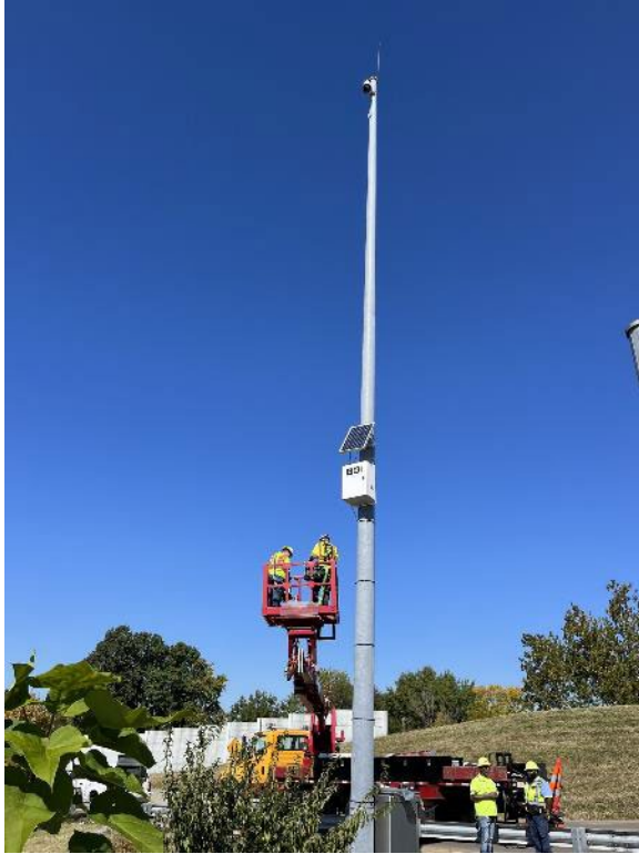
Figure 22. I-64 WB/EB Exit Gore to Big Bend Boulevard – Gateway Installation
