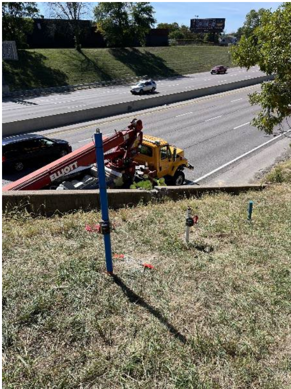
Figure 13. I-44 and Macklind Avenue – In-place Inclinometer and Piezometer Installation
