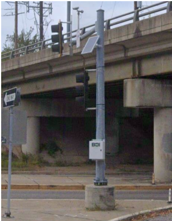
Figure 15. I-44 WB to Berry Road – Gateway Installation
