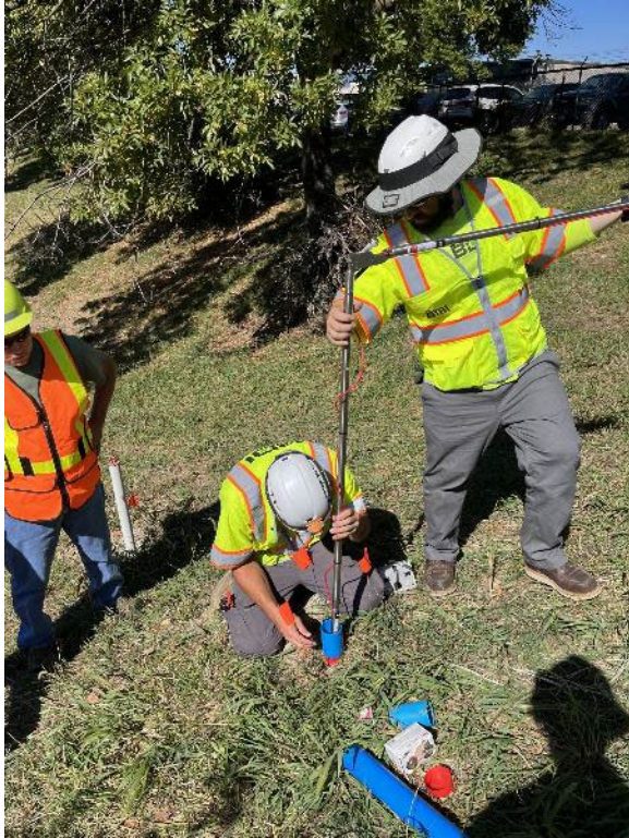
Figure 14. I-44 and Macklind Avenue – Installing In-place Inclinometer
