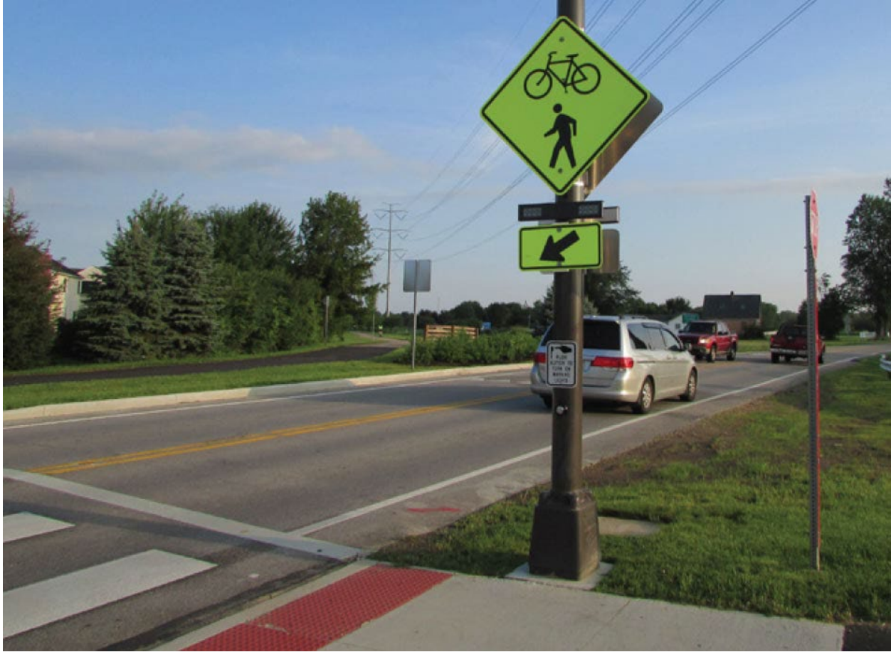
Figure 7-1 Example of RRFB (Source: FHWA-SA-21-053)
