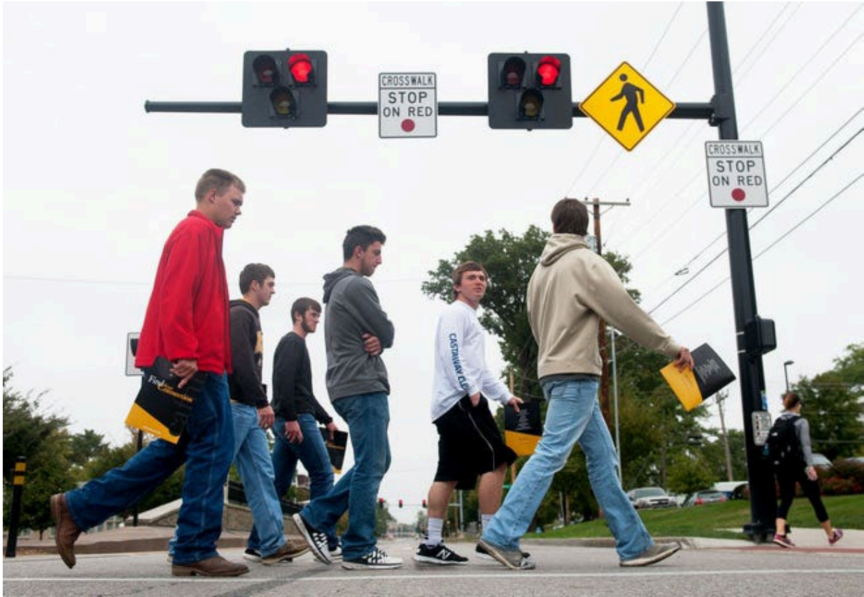
Figure 7-2 Example of PHB Signal (Source: Columbia Daily Tribune, 2015)
