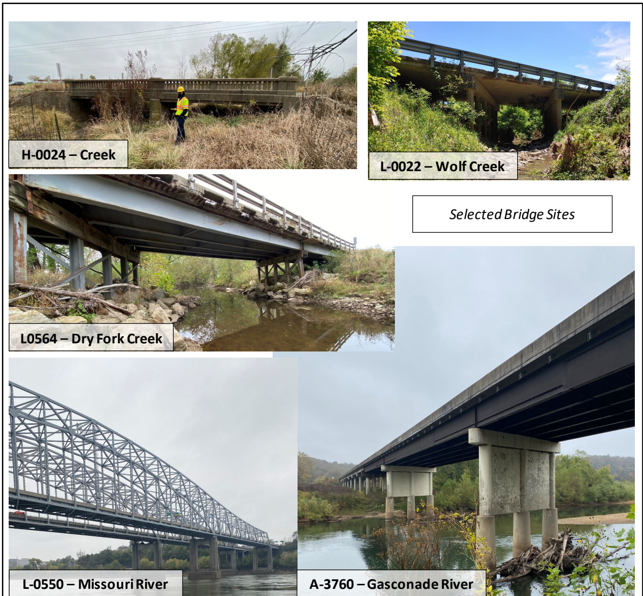
Figure 3-2. Composite of the five bridge sites selected for this study.
