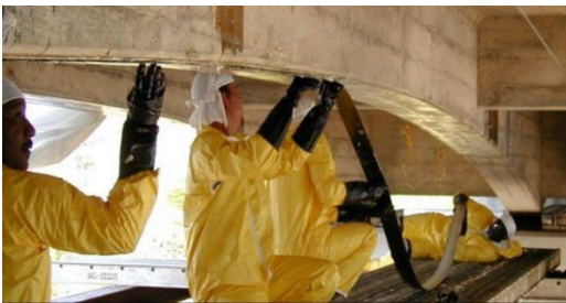
3. Application of FRP on substrate
