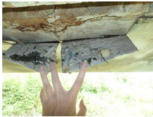
Figure 43 End peeling (Baniya et al. 2022)
