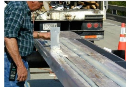
2. Application of resin on FRP and substrate
